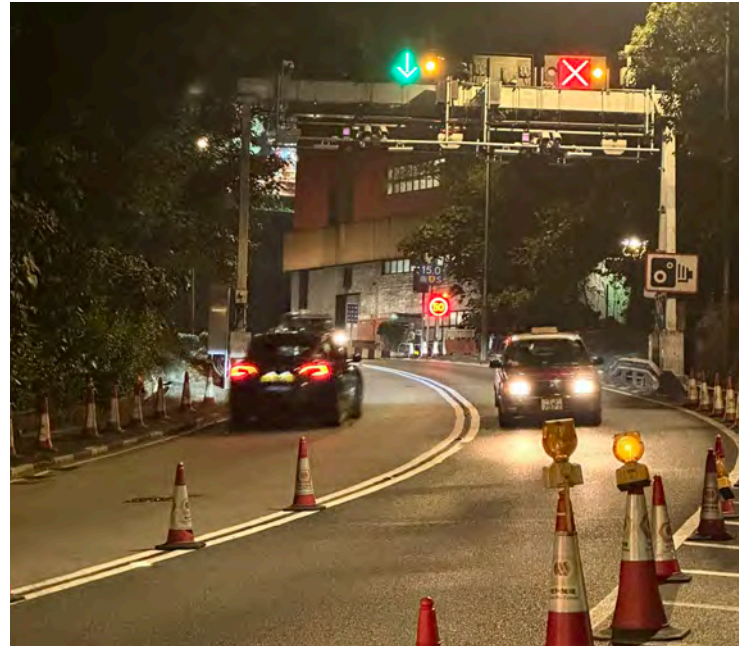
5: ANPR cameras capture front and rear vehicle number plates 6: The TKO-LTT was originally planned to implement the first FFTS in Hong Kong and designed without a toll plaza
