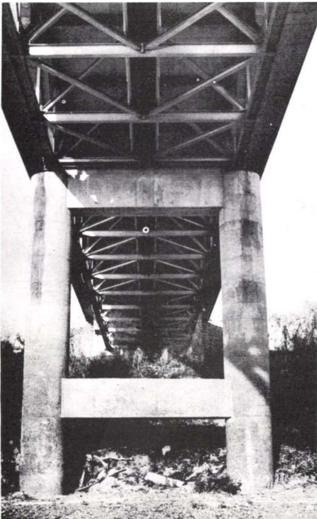
Below: General view from the underside
