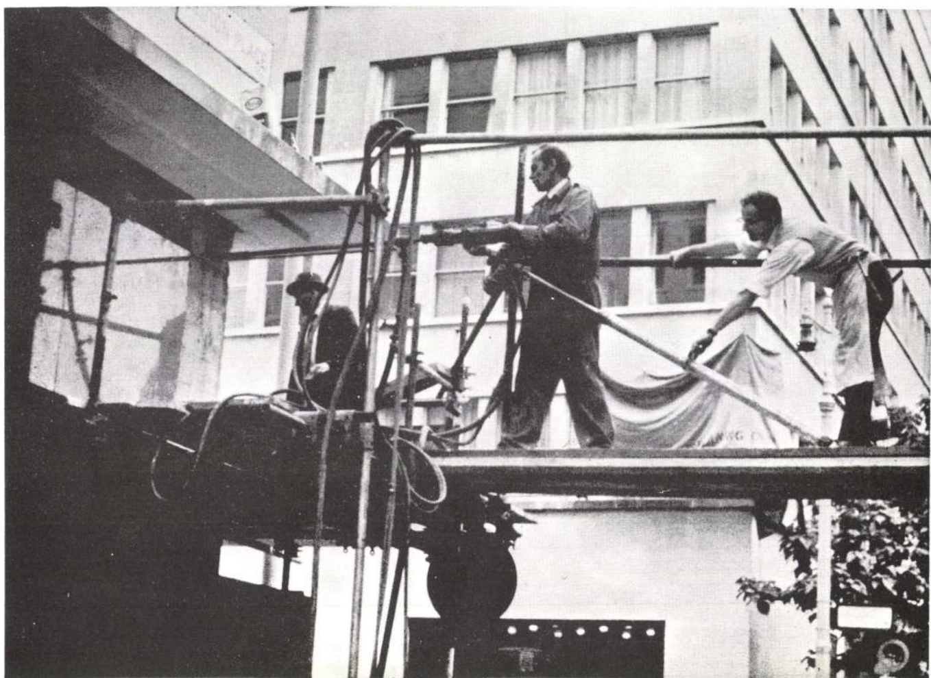
Fig 2. above The drill with 'air leg'
