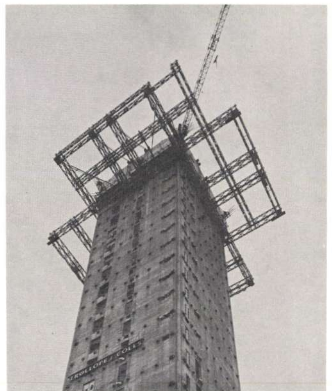
Fig. 5 Underside view of platform during erection (Photo: Fox Photos Ltd.)
