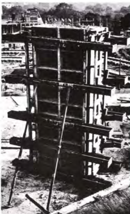
Fig. 16 left Shutter box for a lance-corporal column. All slim-jims and lance-corporals are in fairfaced concrete, and shutter bolts through the columns are not acceptable, hence the strong-backs (Photo: Sam Price)
