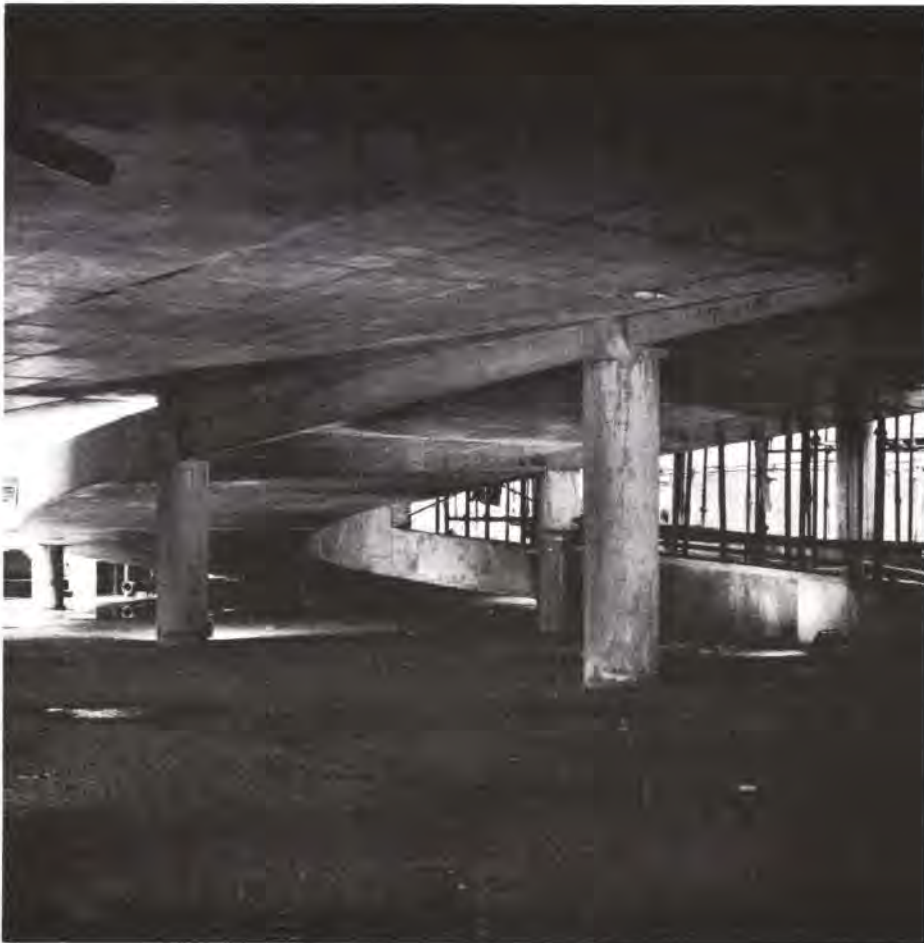
Fig. 8 above Portal beams erected. In situ connections still to be concreted (Photo: Sam Price)
