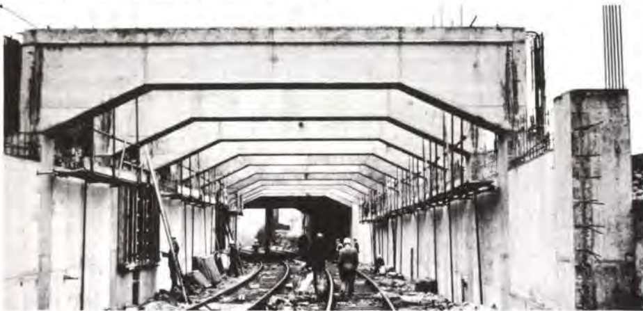
Fig. 8 above Portal beams erected. In situ connections still to be concreted (Photo: Sam Price)
