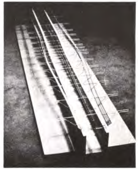
Fig. 13 Model showing prestressing cables for Derwent Bridge (Photo: David Osborne)
