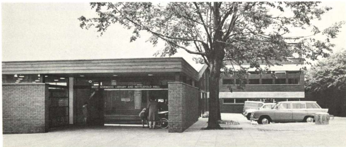
Fig. 4 Library main entrance (Photo: Ernie Hills)
