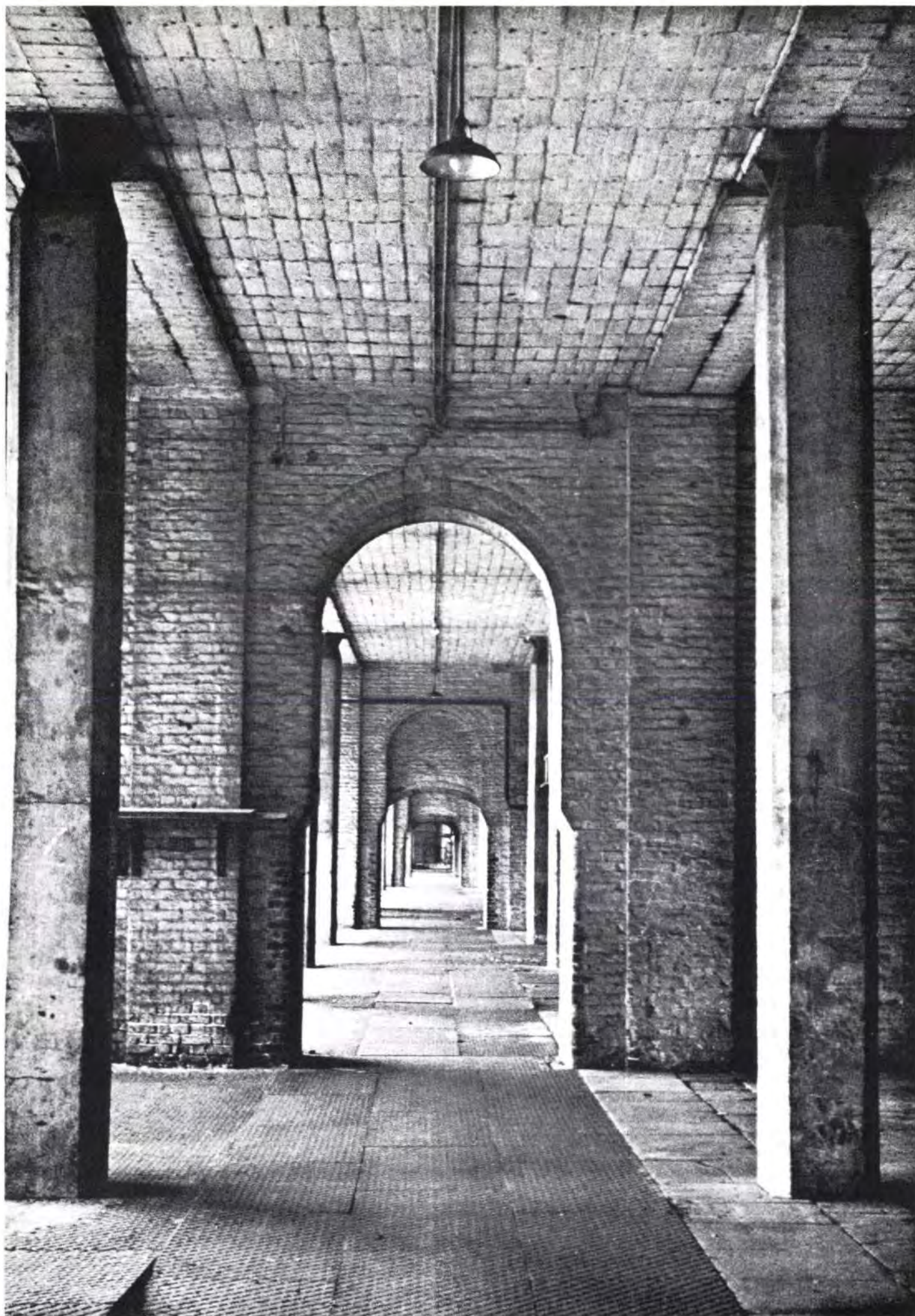
Fig. 6 View along the quay beneath B warehouse, interrupted at intervals by fire walls (Photo: Malcolm Tucker)
