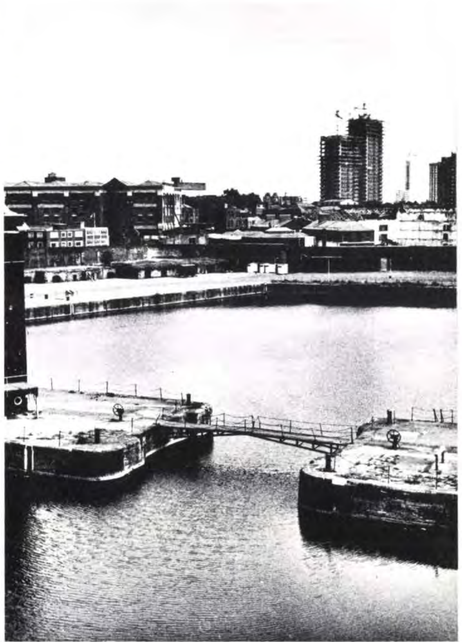
Fig. 16 below Recess in quay for the bowsprit of a sailing ship. Note mooring rig (Photo: Malcolm Tucker)
