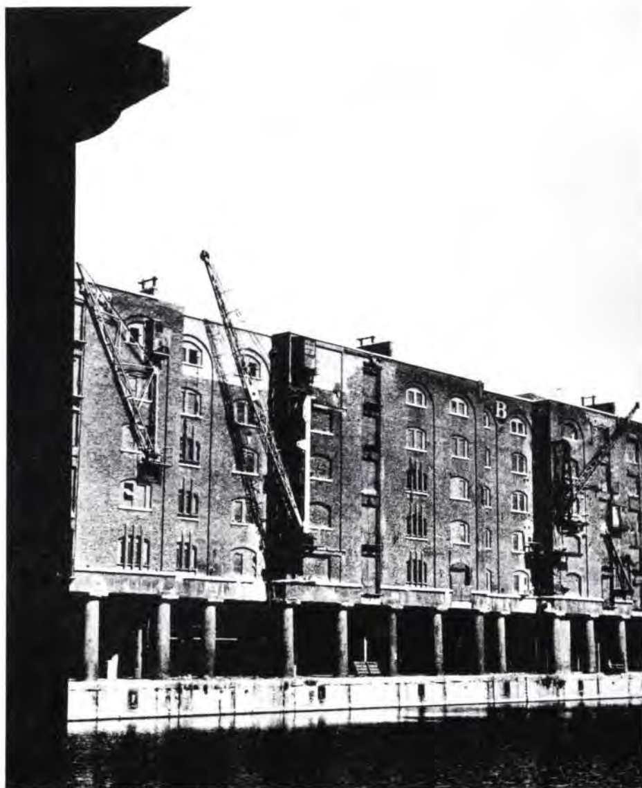
Fig. 4 B warehouse dock facade (Photo: Malcolm Tucker)
