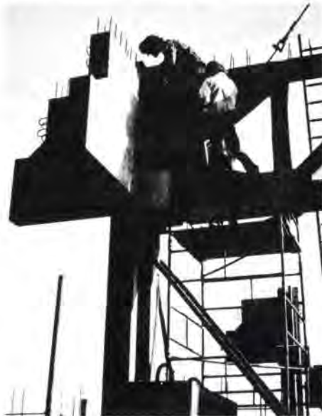
Fig. 5 Connection detail between corner column and precast truss. Side shutters for in situ concrete stitch being fixed (Photo: Beecham Research Laboratories)
