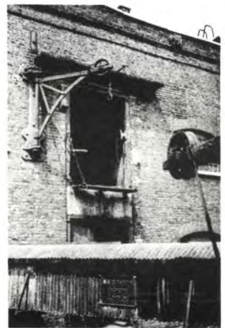
Fig. 17 below A jigger rib on H warehouse (Photo: Malcolm Tucker)
