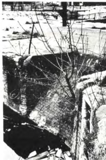
Fig. 16 below Recess in quay for the bowsprit of a sailing ship. Note mooring rig (Photo: Malcolm Tucker)
