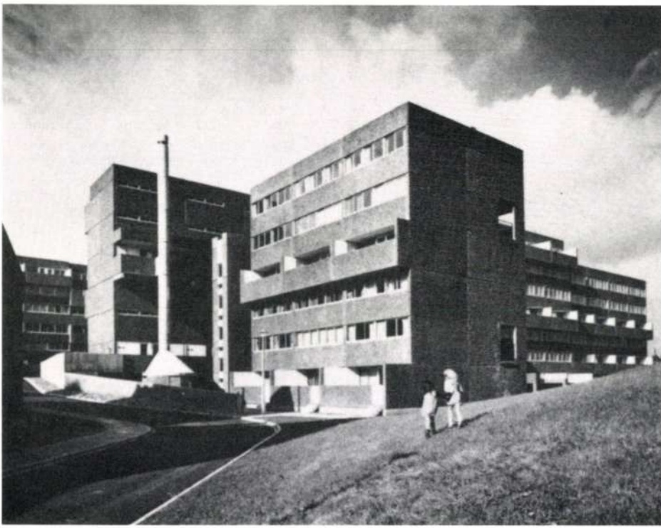
Fig. 2 above Yorkshire Development Group Mk. 1 System: The Leek Street Scheme, Leeds. The Yorkshire Development Group, consisting of the cities of Hull, Leeds, Nottingham and Sheffield, conceived and sponsored this medium-rise, high-density, deck access system, which was intended to provide 4,500 dwellings in three years. The contract was awarded to the Shepherd Building Group,
