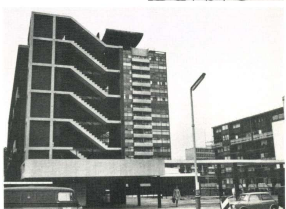
Fig. 6 below Typical staircase (Bowwater House after repair)
