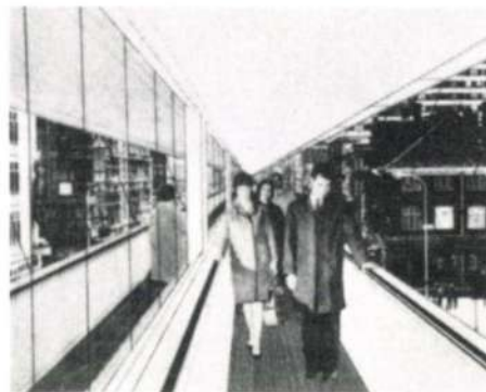
Fig. 4 Interior view of the Speedaway showing glazing spine truss and twin Starglide belt (Reproduced by courtesy of Brian Richards and the Dunlop Company Ltd.)
