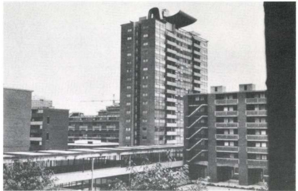
Fig. 3 below Great Arthur House, showing pick-hammered flank walls and roof canopy
