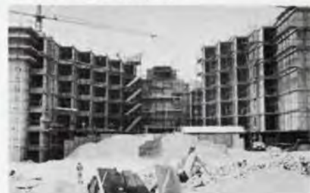
Fig. 9 Riyadh: back of service core (Photo: The contractors)
