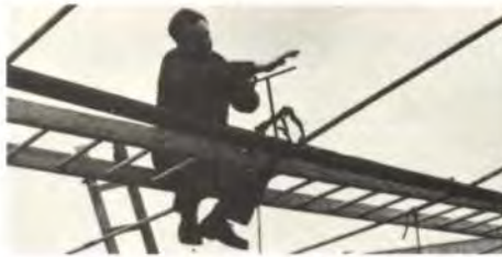
Fig. 3 Attaching the double angles
