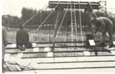
Fig. 4 Attaching the timber panels
