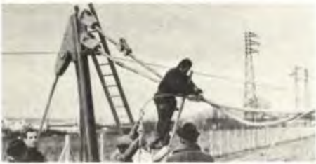
Fig. 1 Connecting cable to boundary cable
