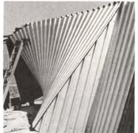
Fig. 10 Detail of the aluminium edge cladding
