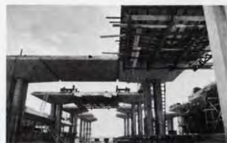
Fig. 10 Riyadh: conference centre, foyer roof (Photo: The contractors)
