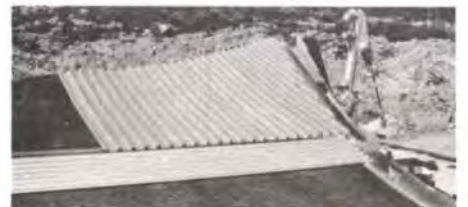
Fig. 11 Detail of aluminium roof cladding
