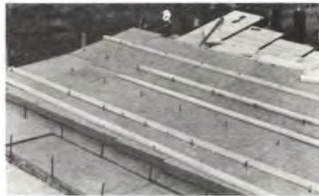
Fig. 5 Connecting the Sillan fibre glass panel
