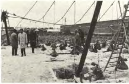
Fig. 2 The cable net with sandbags
