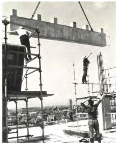
Fig. 9 Erection of precast spine beam (Photo: Keppie Henderson & Partners)
