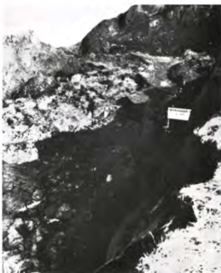
Fig. 7 View of 1953 slip from the centre looking east Photo: Courtesy Soil Mechanics Ltd.
