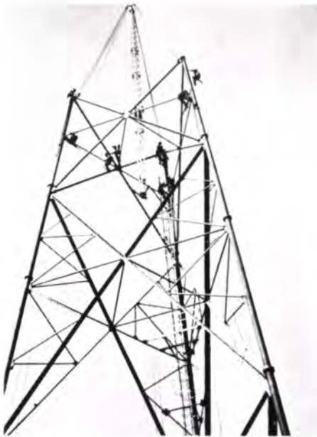
Fig. 10 Tower erection in Nigeria
