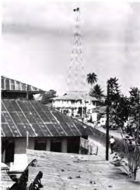
Fig. 12 Completed Heavy route tower
