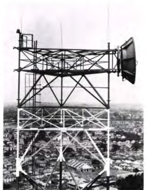
Fig. 13 Top of Heavy route tower showing aerial mounting panel
