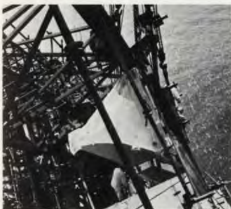
Fig. 4 Holding a rib segment in place while glueing is carried out (Photo: Max Dupain)
