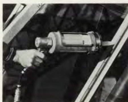
Fig. 27 Application of silicone rubber seal (Photo: Harry Sowden)
