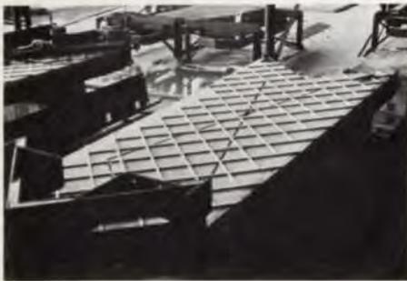
Fig. 31 A tile-lid mould with aluminium strips (Photo: Courtesy Structural Engineer)
