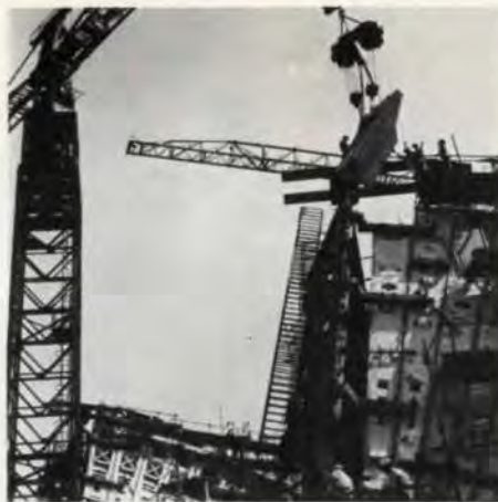
Fig. 2 Lifting a rib segment into position (Photo: Max Dupain)
