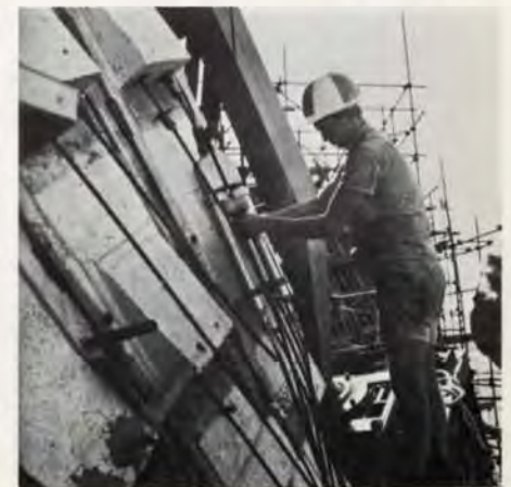
Fig. 35 Special double-piston jack in use for temporary stressing (Photo: Max Dupain)
