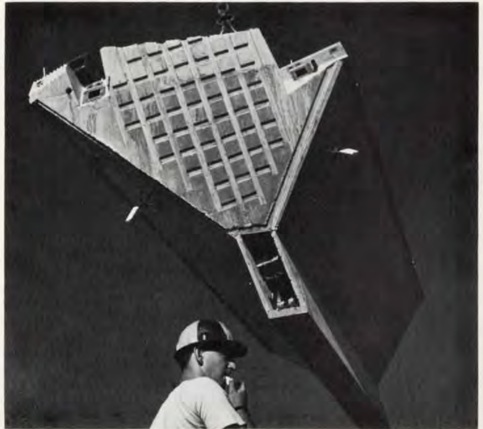
Fig. 23 A top segment of a rib (Photo: Max Dupain)
