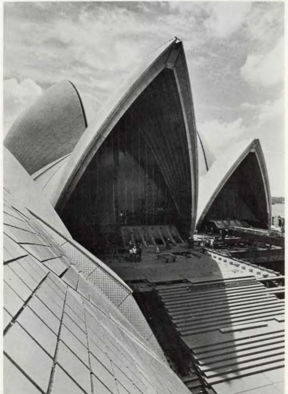
Fig. 10 Glass wall A4: structure (Photo: Harry Sowden)
