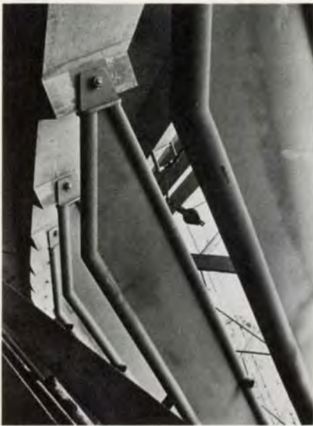
Fig. 8 Detail of corbels (A4) (Photo: Harry Sowden)
