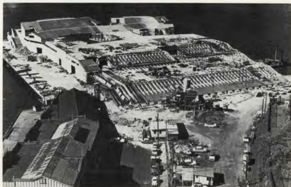
Fig. 11 Aerial photograph of site showing Concourse area
