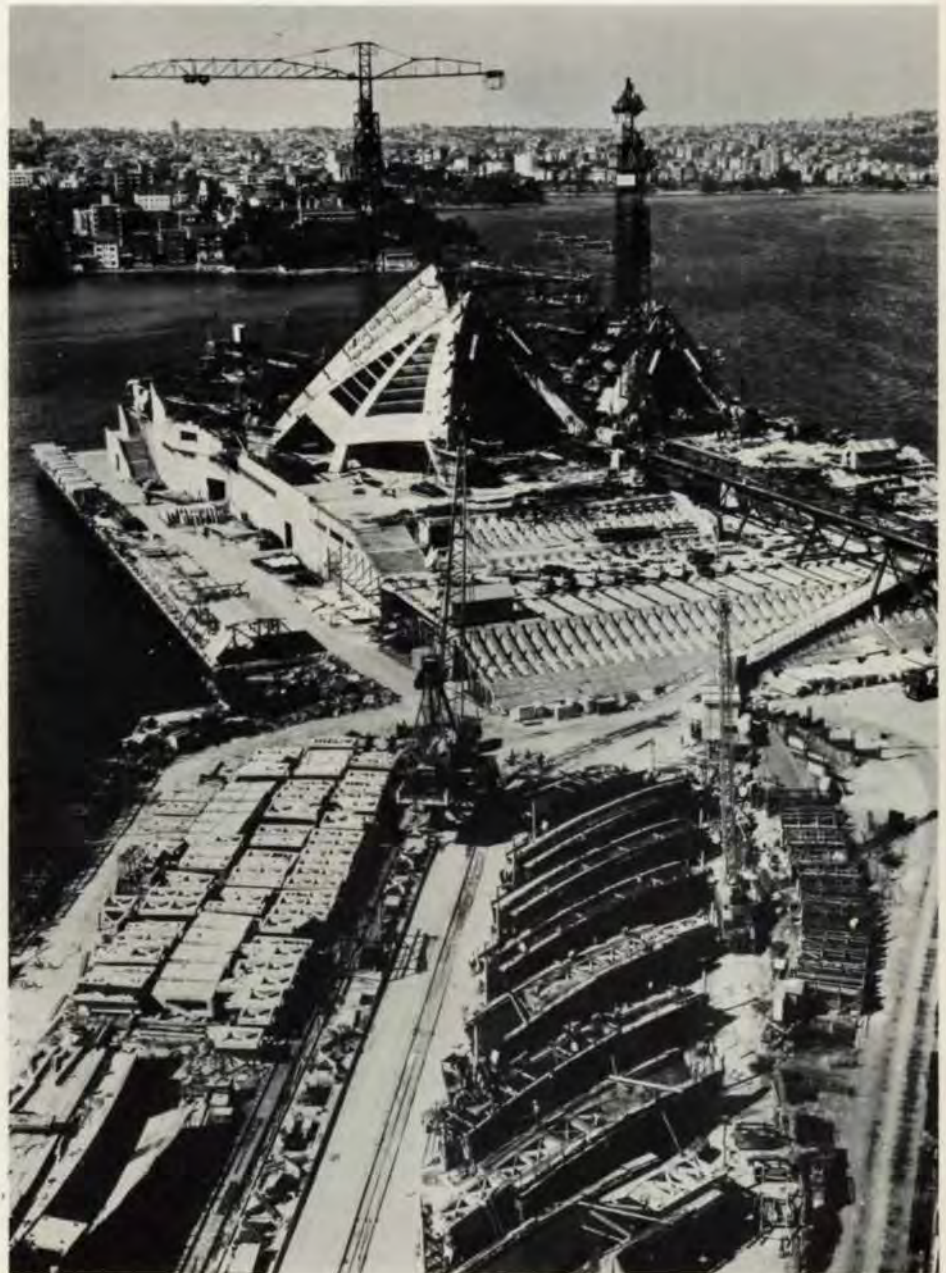
Fig. 30 The precasting yard and the site (Photo: Max Dupain)
