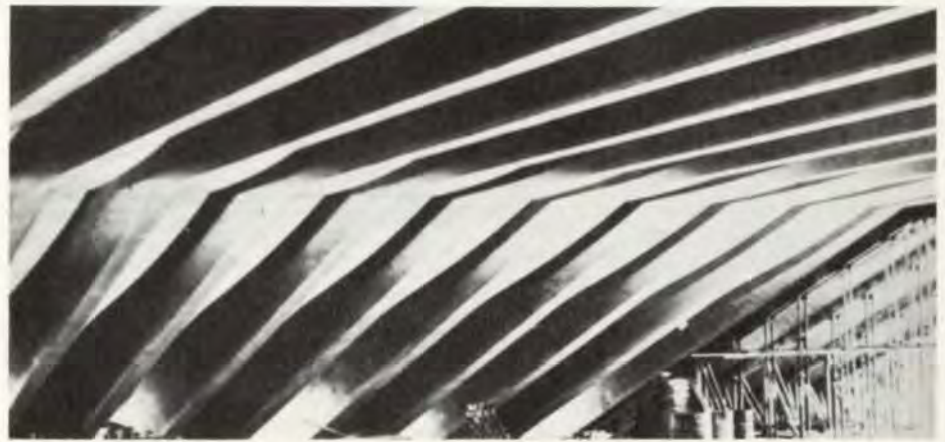
Fig. 16 View of the concourse soffit
