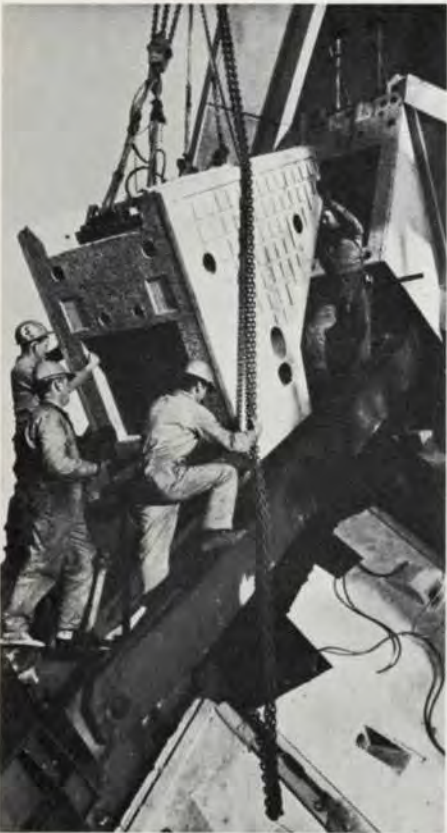
Fig. 25 A ridge segment going into position (Photo: Max Dupain)
