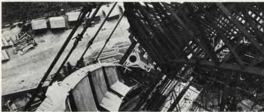
Fig. 3 View down a rib under construction (Photo: Geoffrey Wood)
