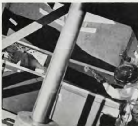
Fig. 5 Applying the epoxy resin adhesive to both surfaces (Photo: Max Dupain)
