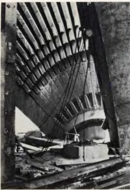
Fig. 24 Shell A2 pedestal and lower segments showing anchorage pockets (Photo: David Dowrick)
