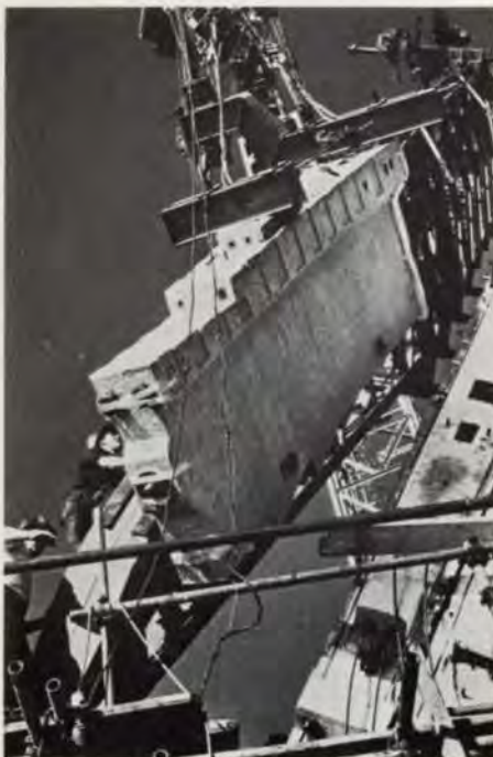
Fig. 33 Erection of a segment (Photo: Max Dupain)
