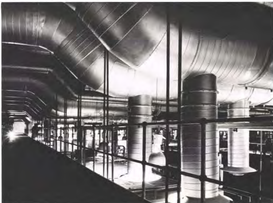
Below: Bottling hall: view from visitors walk way showing ventilation trunking (All photos in this section: Colin Westwood)
