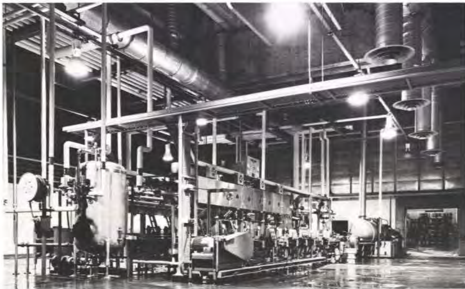
Below: Bottling hall: view from visitors walk way showing ventilation trunking (All photos in this section: Colin Westwood)
