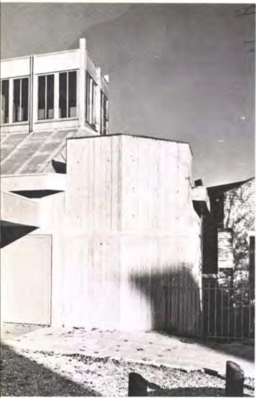
Fig. 6 Pedestrian entrance off Lawn Terrace
