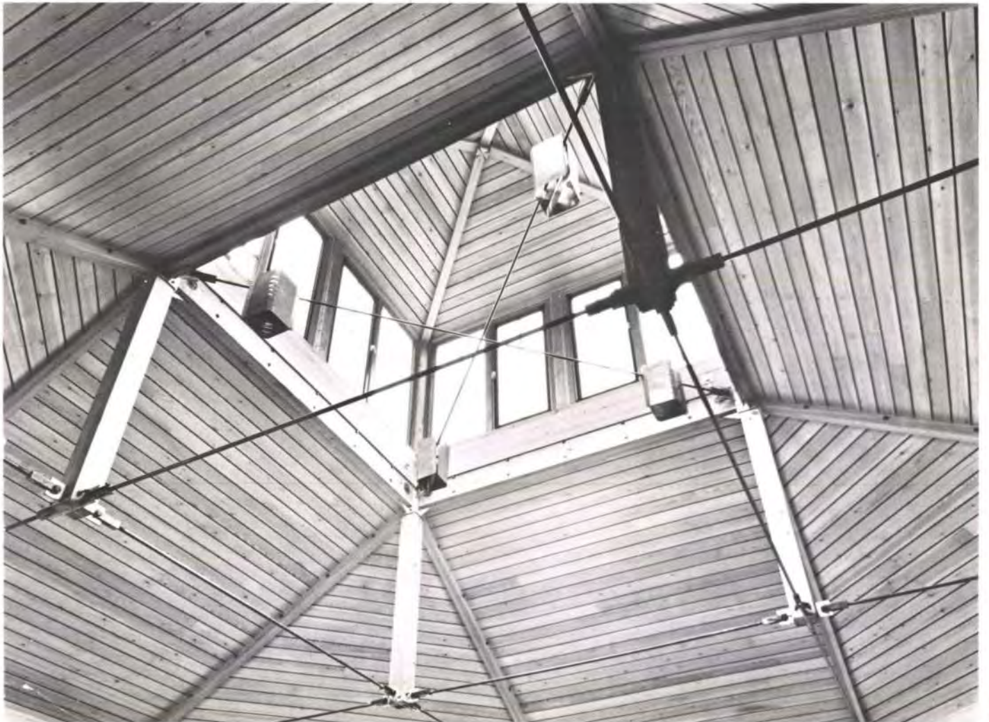
Fig. 7 Roof structure showing lantern and steel ties
