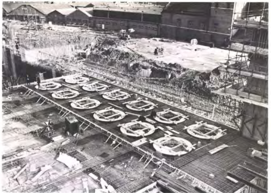
Above: Fermenting cellar: ground floor slab
