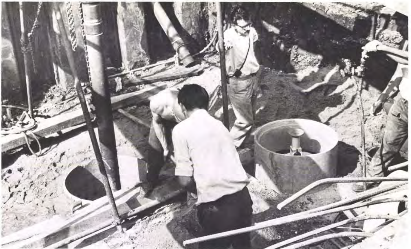
Fig. 12 Site installation of earth pressure cell and pile load cell
