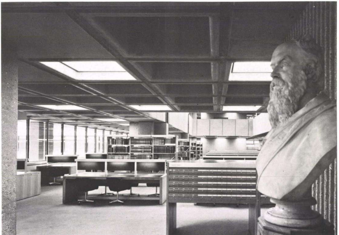
Fig. 20 Reference library – Entrance to science and technology library on the 5th floor with marble bust of Samuel Timmins. Note junction of ribbed grit blasted wall and smooth coffer ceiling
