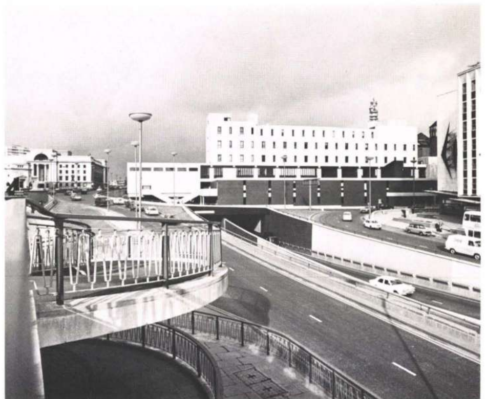
Fig. 6 School of music with shopping centre beneath. Note recital room adjacent to busy road with underpass beneath
