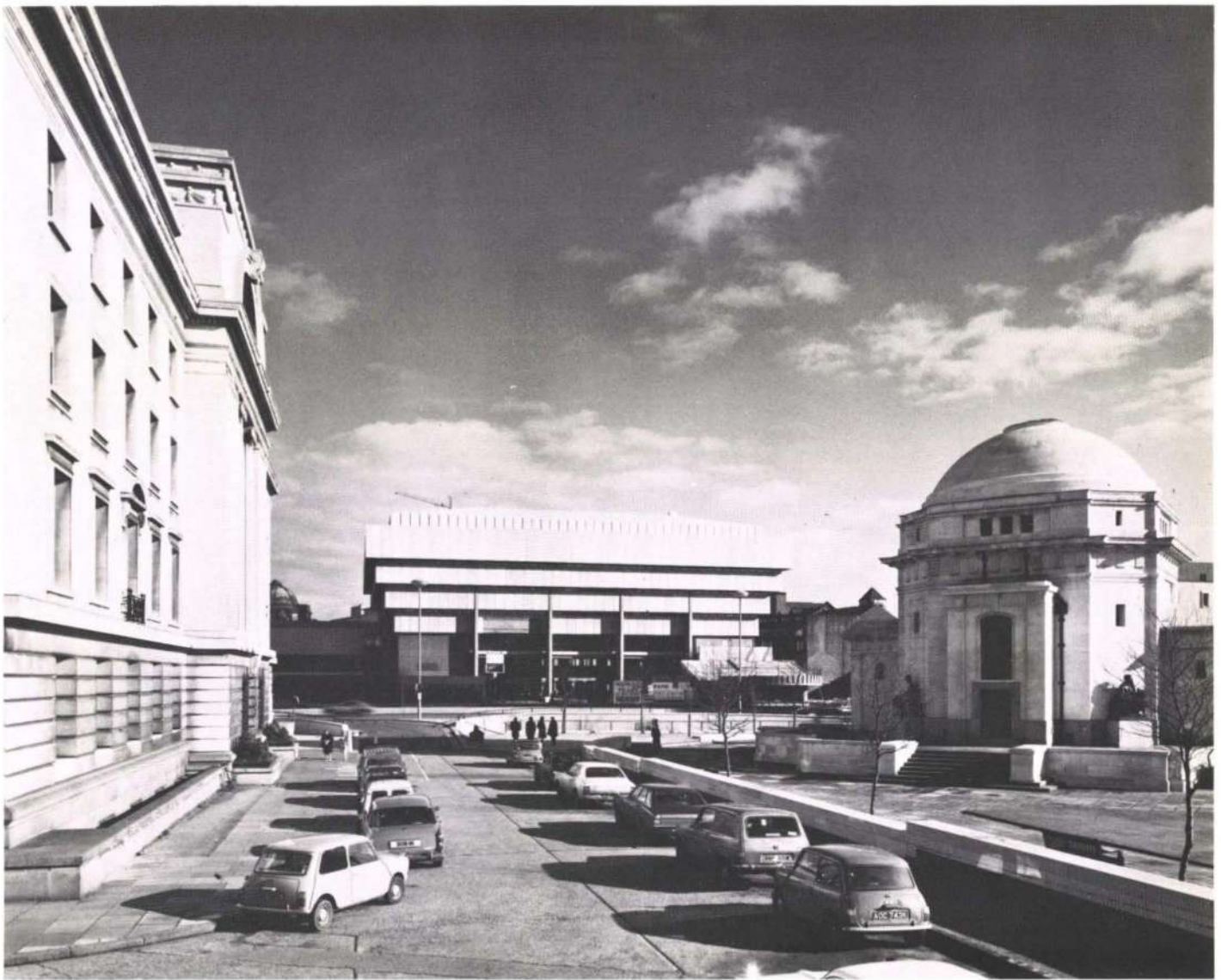
Fig. 5 View of reference library with Baskerville House and Hall of Memory in foreground
