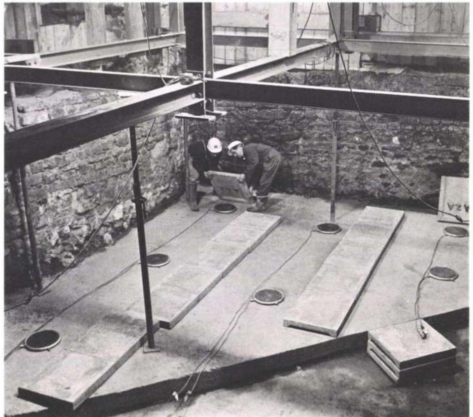
Fig. 8 Placing flatjacks and inverted concrete troughs prior to casting foundation extension to central tower of York Minster
