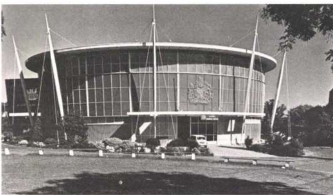
Fig. 9 UK Pavilion, Rand Centre near Johannesburg. The cables were stressed by raising the pylons on flatjacks. (Photo : Brian Jouxsov)
