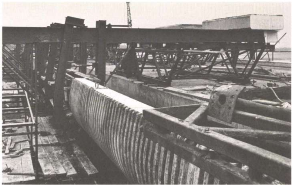
Fig. 15 Ribbed edge & steel frames for edge forms. (Photo: Harry Sowden)
