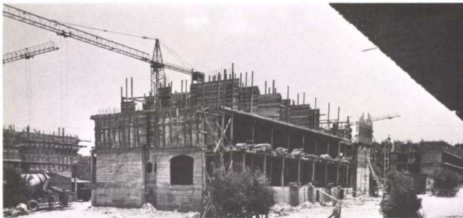
Fig. 10 Dormitories – House 6 – Block 5. View from south west
