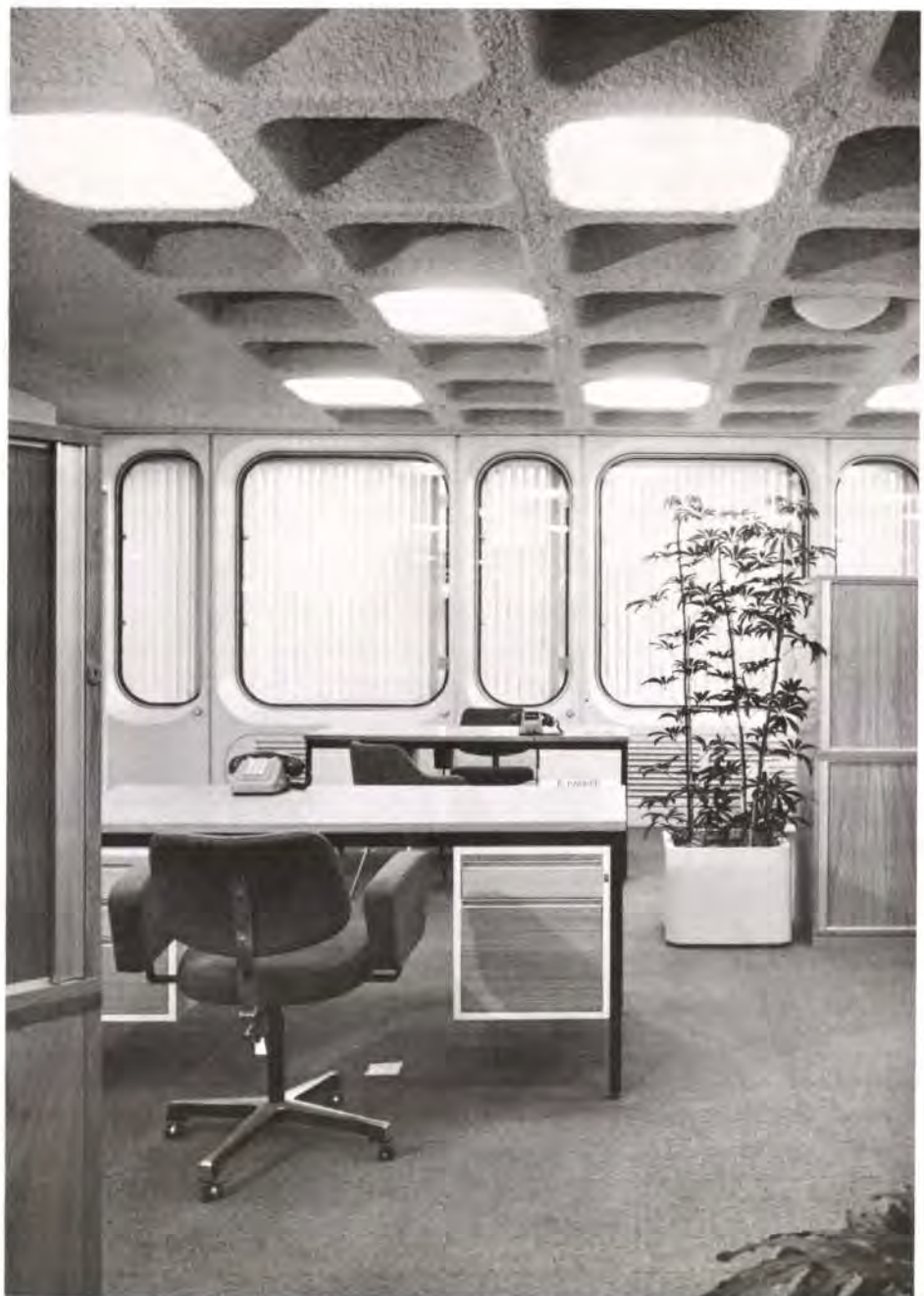
Fig. 8 Typical office interior showing the GRP liners and the acoustic treatment to the coffered soffit
