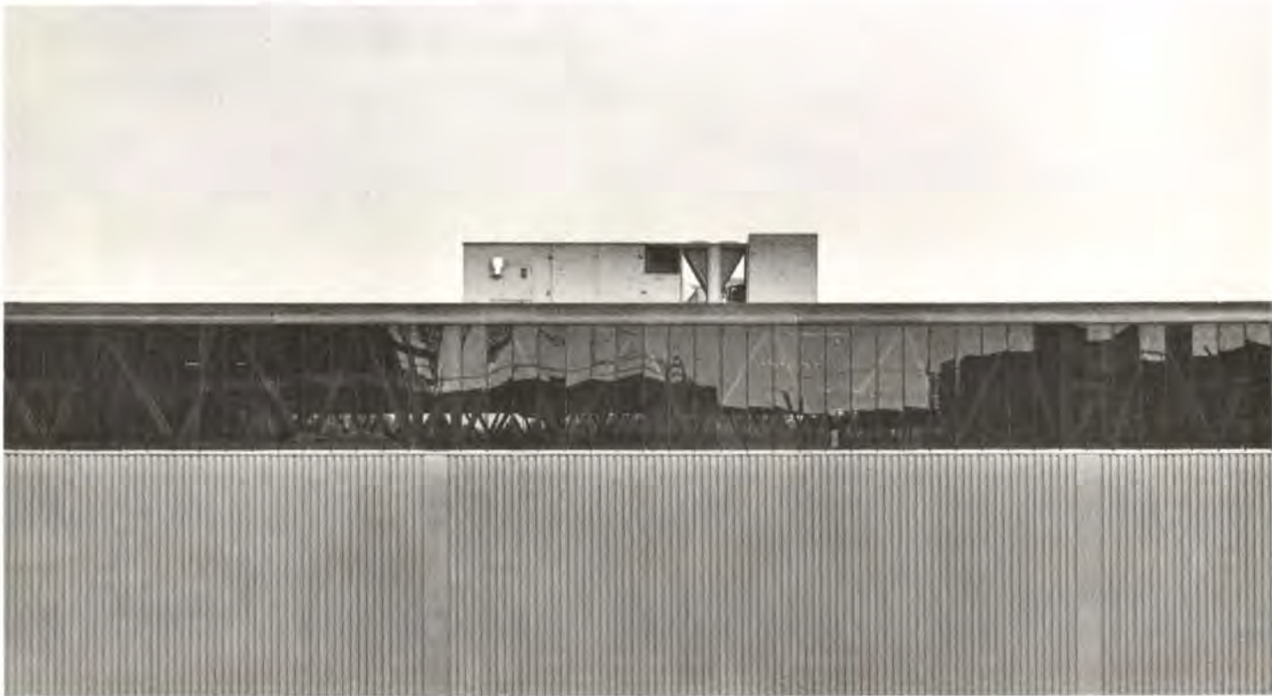
Fig. 1 Exhibition Hall cladding and glazing with air handling unit. (Photo: Harry Sowden)
