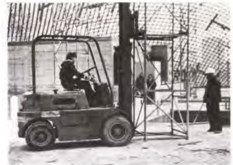
Fig. 20 Fork lift truck being used to raise a tower
