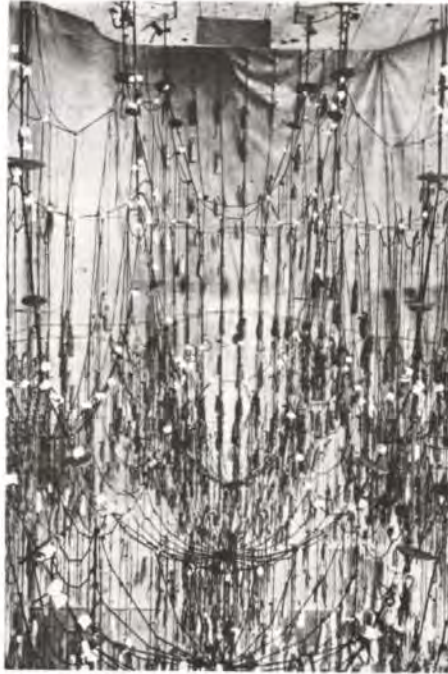
Fig. 2a Hanging model by A. Gaudi
