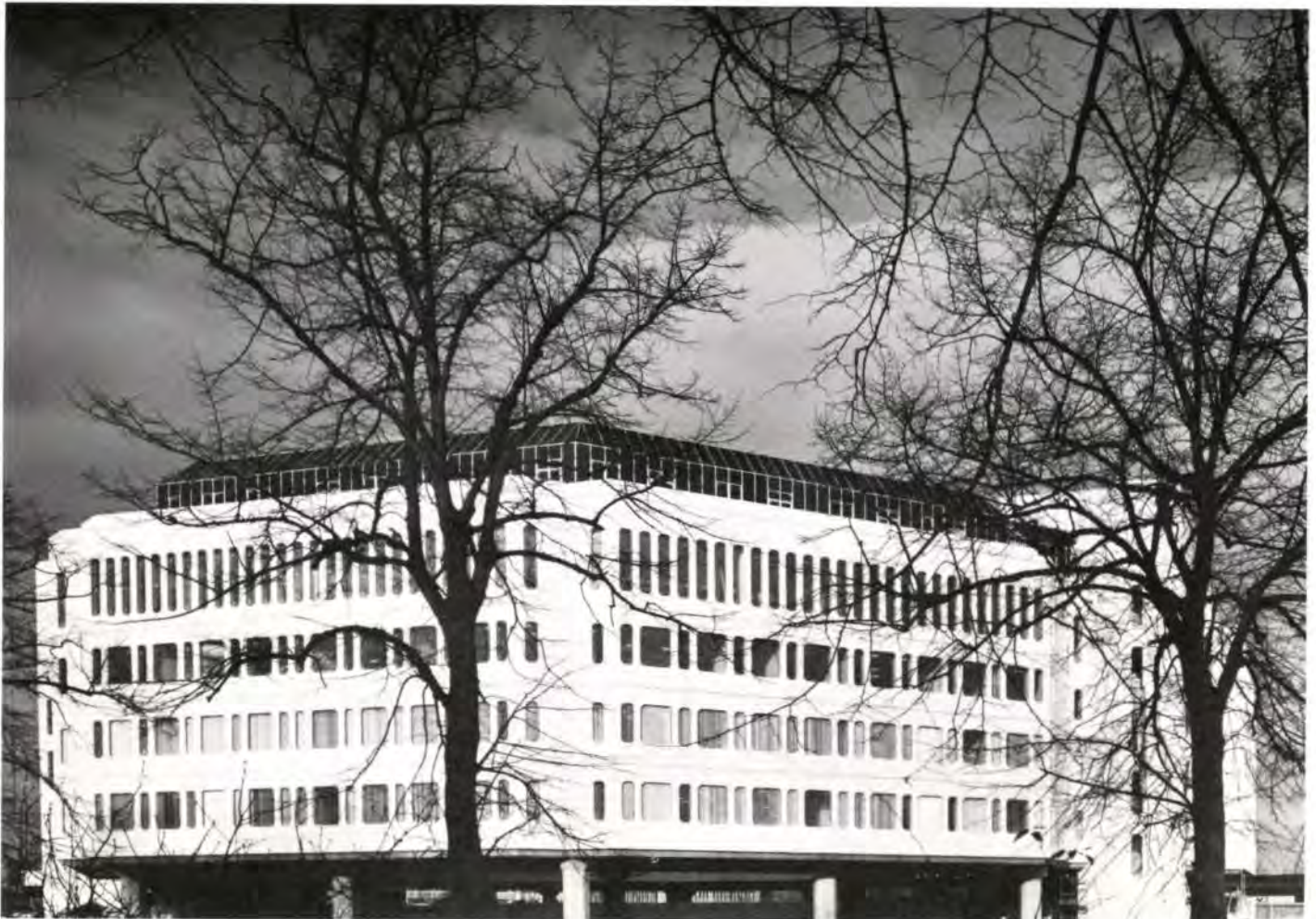
Fig. 4 Elevation of the office block (nearing completion) from the Forbury road
