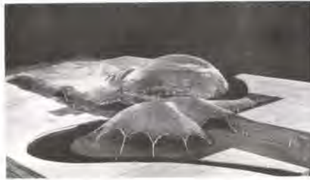
Fig. 9 Frei Otto's wire mesh model for Mannheim
