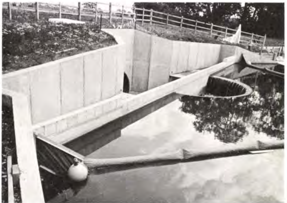
Fig. 8 Lake outfall, the hydraulic control structure and oil booms
