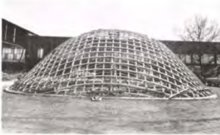
Fig. 3 Lattice dome at Essen 1962
