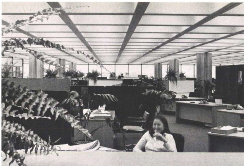
Figs. 18 & 19 Interior views of the offices
