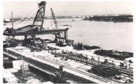
Fig. 17 The mechanical unloader being assembled (Photo: Geoffrey Wood)
