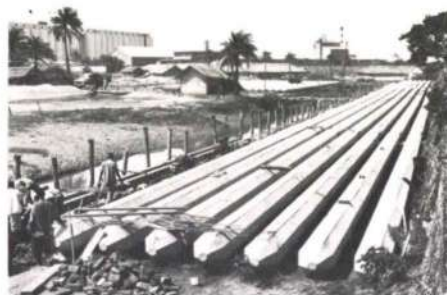
Fig. 7 Pile casting yard adjacent to Khal 7 (Photo: Ove Arup & Partners)
