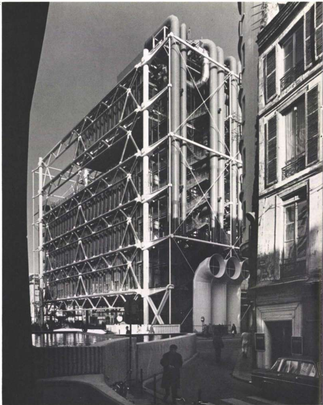
Fig. 2 View from Rue St. Marie showing services on rear façade at right of photograph (Photo: Martin Charles; courtesy of Architects' Journal )
