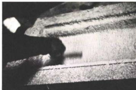
Fig. 6 Compacting GRC with hand roller (Photo: Brian Cole)
