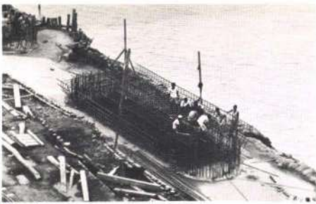
Fig. 12 Assembling the rear beam reinforcement cage (Photo: Ove Arup & Partners)
