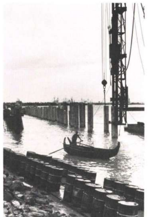
Fig. 8 Pile driving with pile-carrying pontoon in foreground (Photo: Dick Wright)
