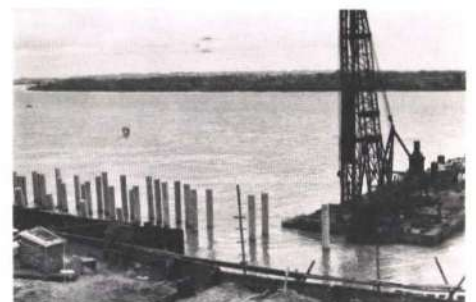
Fig. 11 Barge mounted piling rig (Photo: Dick Wright)
