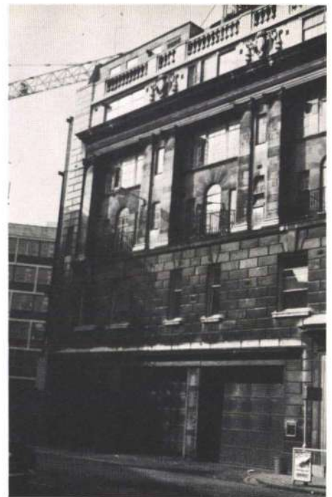
Fig. 7 Existing fire station building showing steel tie back restraint at left corner (Photo: Michael Courtney)
