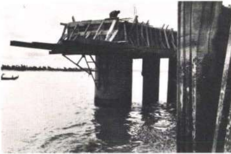
Fig. 14 below Fender panel steelwork (Photo: Geoffrey Wood)
