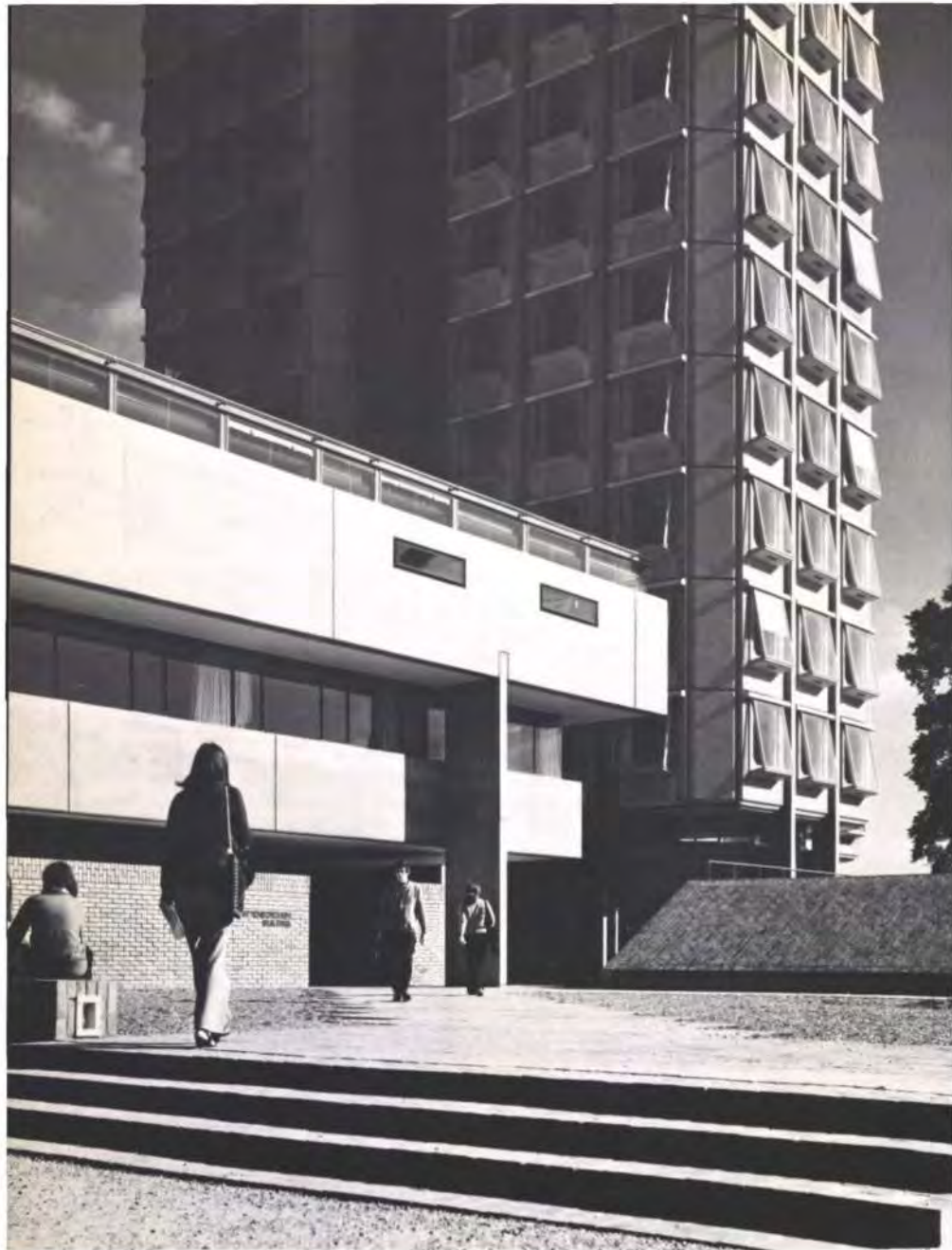
Fig. 53 Arts & Commerce tower: Lecture theatre and seminar rooms in low block linked to 17 storey office tower
