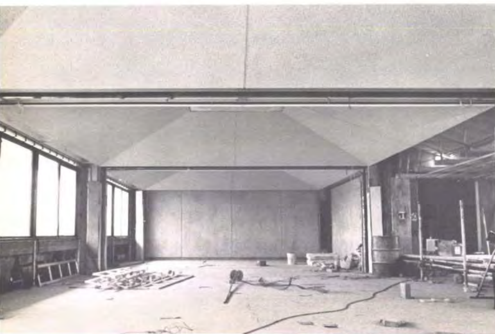
Fig. 27 right Lloyd's under construction. 'Spaces within'
