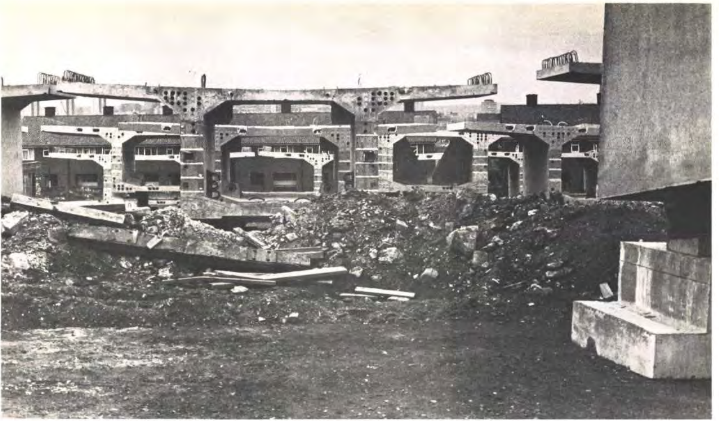
Fig. 8 Stacked segments. Near the centre is a segment with a diaphragm (Photo: Bill Smyth)
