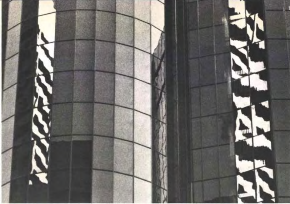
Fig. 50 Reflections and the play of light and fractured images reduce the apparent mass of the building
