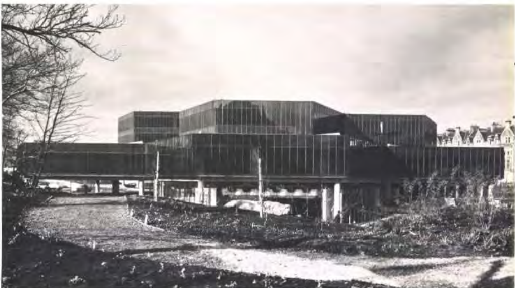
Fig. 8 View of building from landscaped car park roof (Photo: Henk Snoek)
