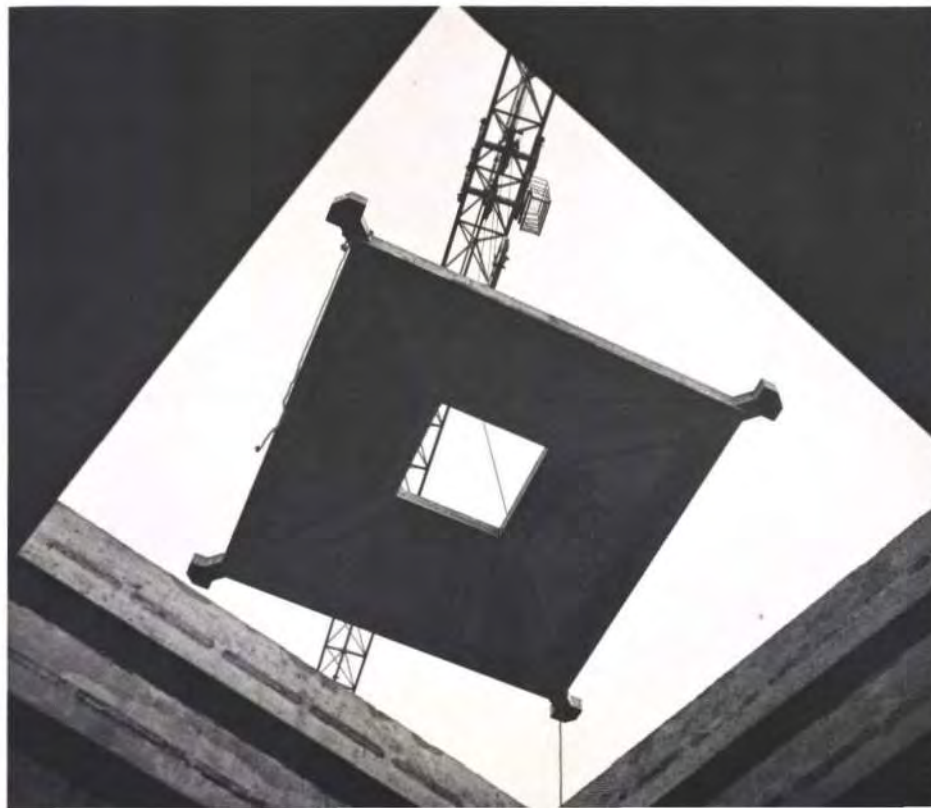
Fig. 25 Lloyd's: erection of an 8.5 tonne precast pyramid
