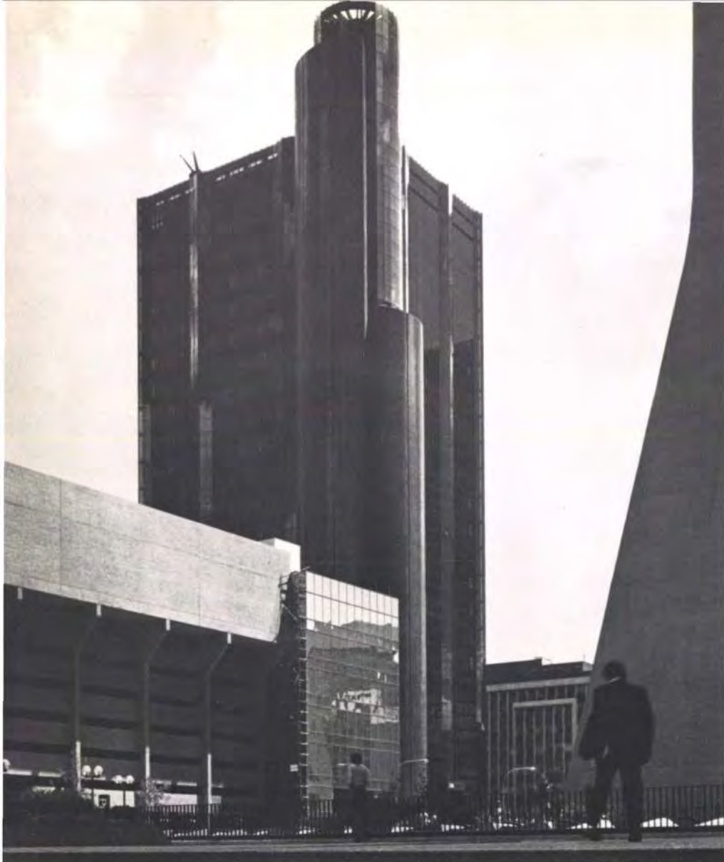
Fig. 47 IBM Johannesburg: external core with low and high rise lift segments
