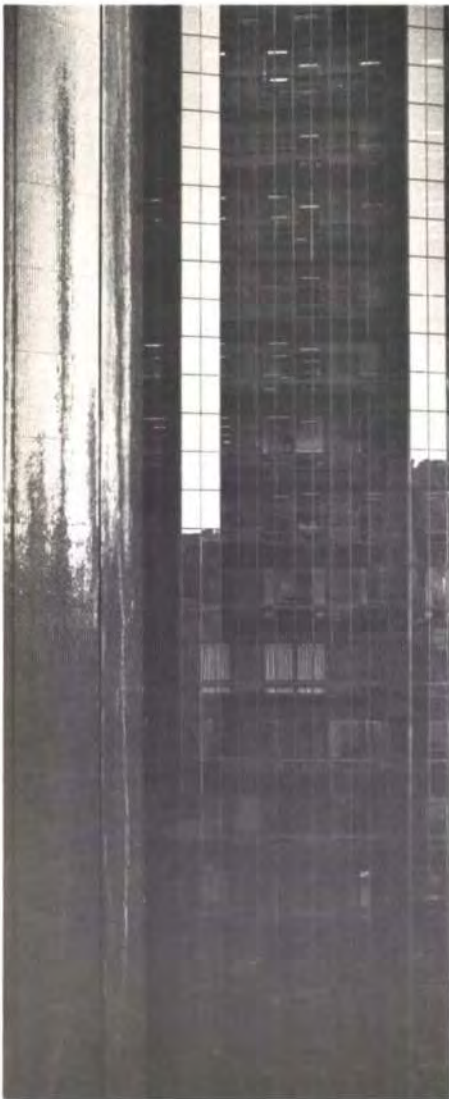
Fig. 51 The elevation showing the random arrangement of partitions on the inner skin
