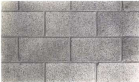
Fig. 4 Detail of blockwork (Photo: Harry Sowden)
