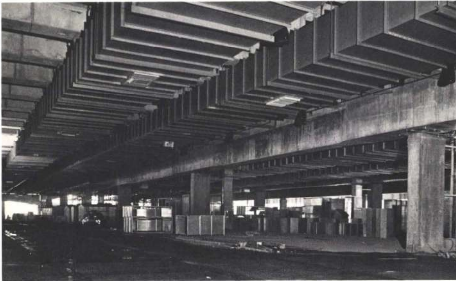
Fig. 8 Depot during installation of services (Photo: M. T. Walters)
