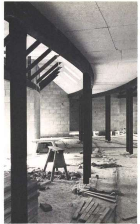
Fig. 5 The curved laminated timber beams in the library (Photo: Harry Sowden)
