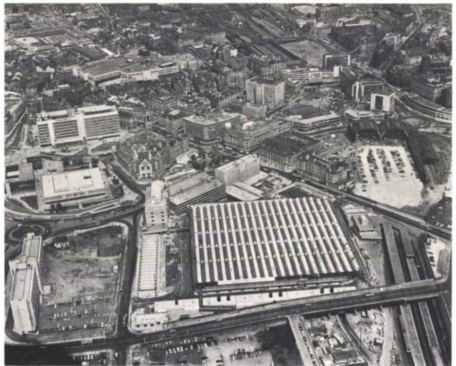
Fig. 1 The interchange nearing completion showing its relationship to the city centre, looking north; Centre right – what remains of the old Exchange Station. Centre left – City Hall and Law Courts (Photo: Bradford Telegraph and Argus )
