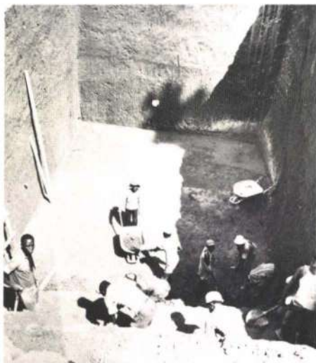
Fig. 17 Excavation for the stout brewery malt intake substructure
