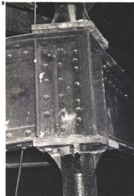
Fig. 9 The original steelwork (Photo: Tony Broomhead)
