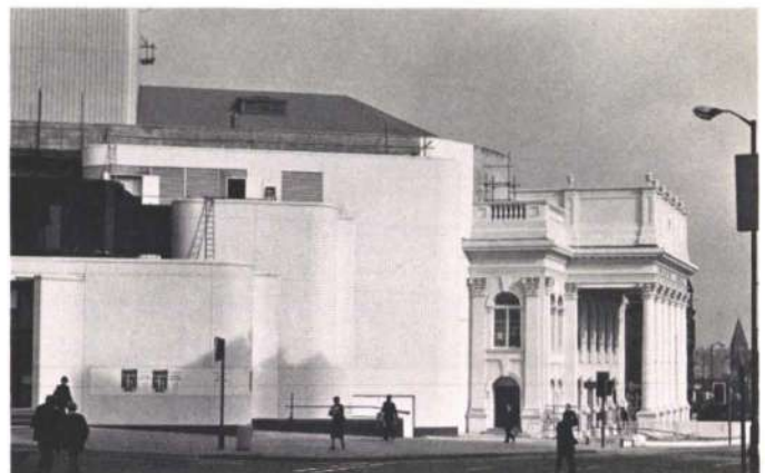
Fig. 23 Exterior view showing new dressing rooms and existing portico (Photo: Courtesy of Renton Howard Wood Levin Partnership)
