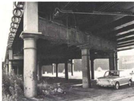
Fig. 4 Croft Street bridge before underpinning (Photo: British Rail)
