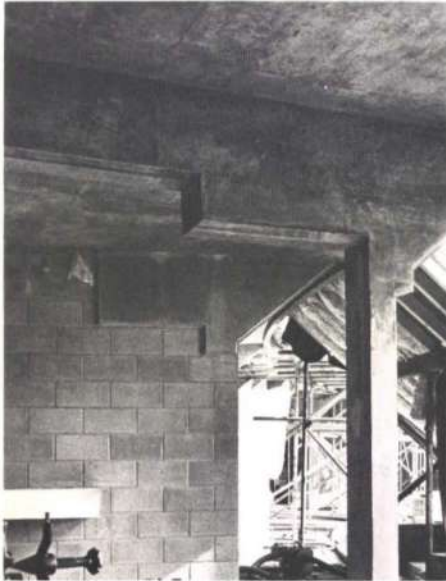
Fig. 3 The fairfaced blockwork in the interior (Photo: Harry Sowden)
