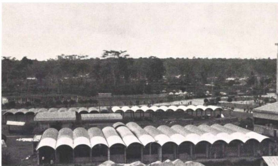
Fig. 19 View during extension of amenity buildings
