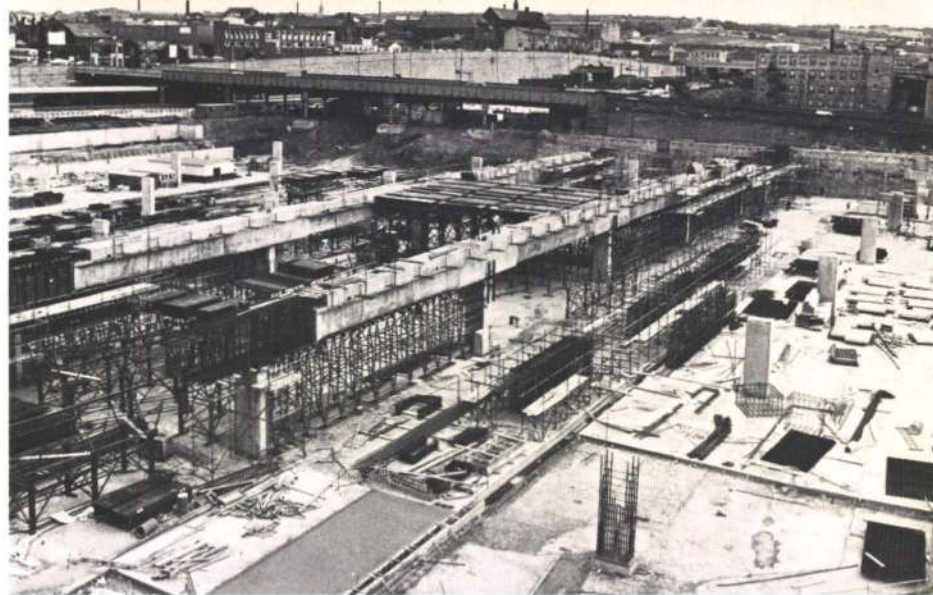
Fig. 7 Bus station deck under construction with underpinned bridge and diaphragm wall in background (Photo: M. T. Walters, Mexborough)
