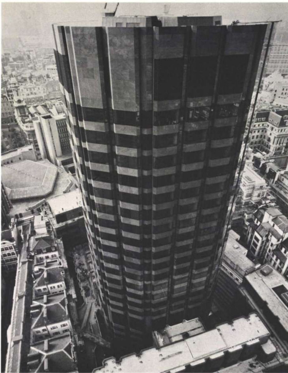
Fig. 7 North elevation of tower at August 1978 (Photo: Sir Robert McAlpine & Sons Ltd)
