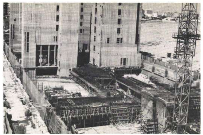
Fig. 8 Close-up of slipformed cores under construction, 17 April 1977 (Photo: Oscar Matri, Kuwait)
