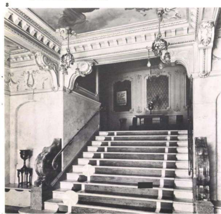
Fig. 9 The main foyer and staircase during restoration (Photo: F. Jewell-Harrison)
