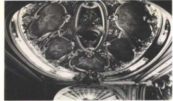
Fig. 4 The auditorium ceiling before restoration (Photo: Arup Associates)
