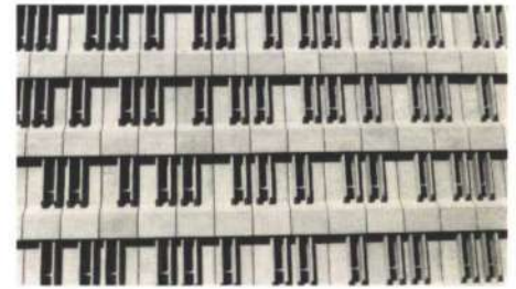
Fig. 6 Detail of cladding panels (Photo: Bob Walster)
