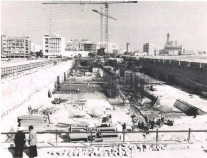
Fig. 4 The excavation at 26 December 1976, showing wellpoint dewatering (Photo: Oscar Matri, Kuwait)
