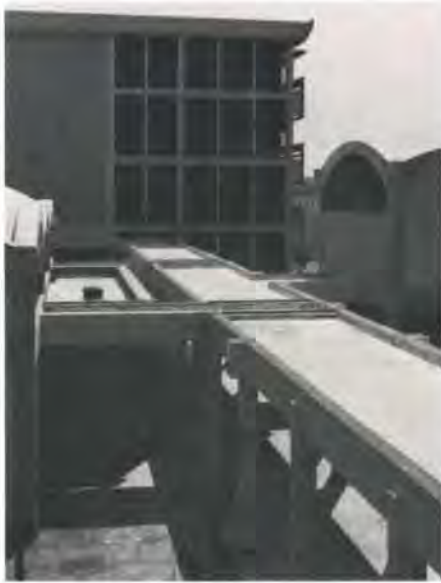
Fig. 7 Faculty of Agriculture: covered walkway adjacent to recreation centre and bookshop (Photo: James Cubitt, Fello Atkinson & Partners)
