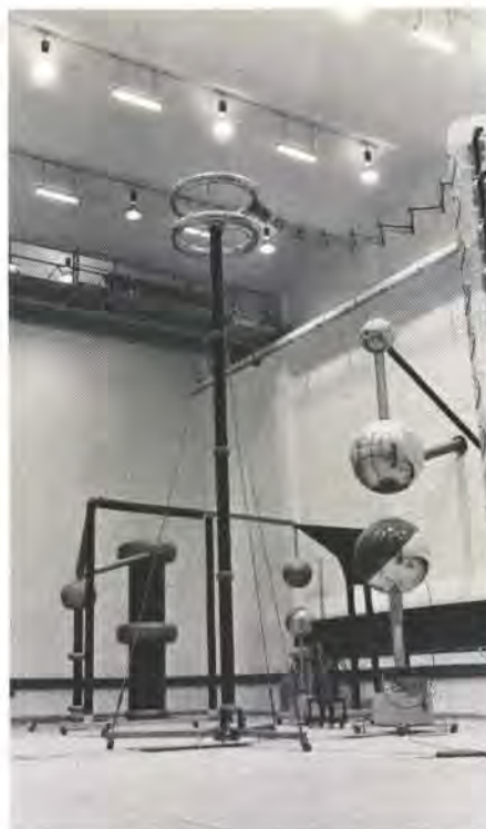
Fig. 18 High Voltage Laboratory: main test hall showing test equipment and overhead crane (Photo: Colin Wade)
