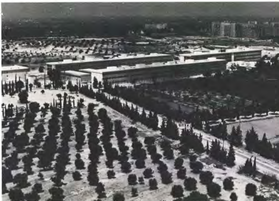
Fig. 19 High Voltage Laboratory and Faculty of Agriculture: view from top of central plant chimney (Photo: Colin Wade)
