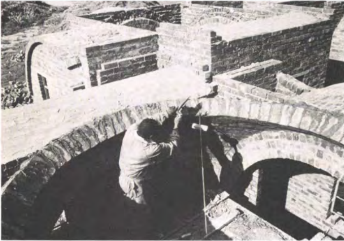
Fig. 5e Low-cost housing : dome and vault (Photo : Ove Arup & Partners, Zimbabwe)
