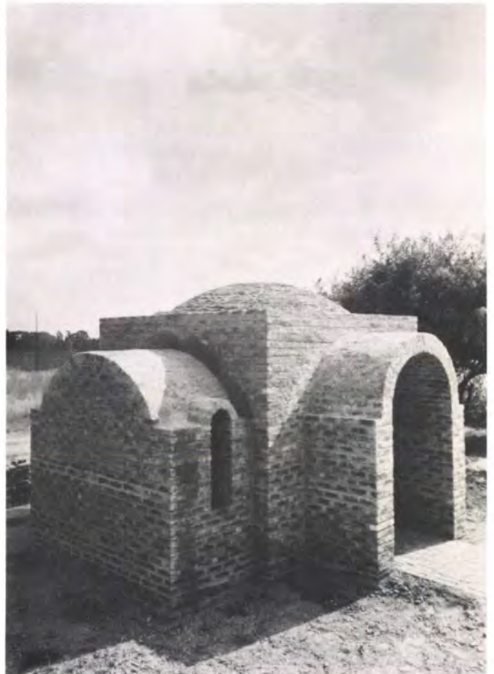
Fig. 5c Experimental house : 4.24m diameter vault and dome (Photo : Ove Arup & Partners, Zimbabwe)
