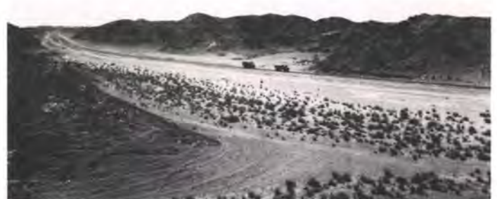
Fig. 3 Existing road through wadi in igneous rock terrain (Photo: Keith Law)
