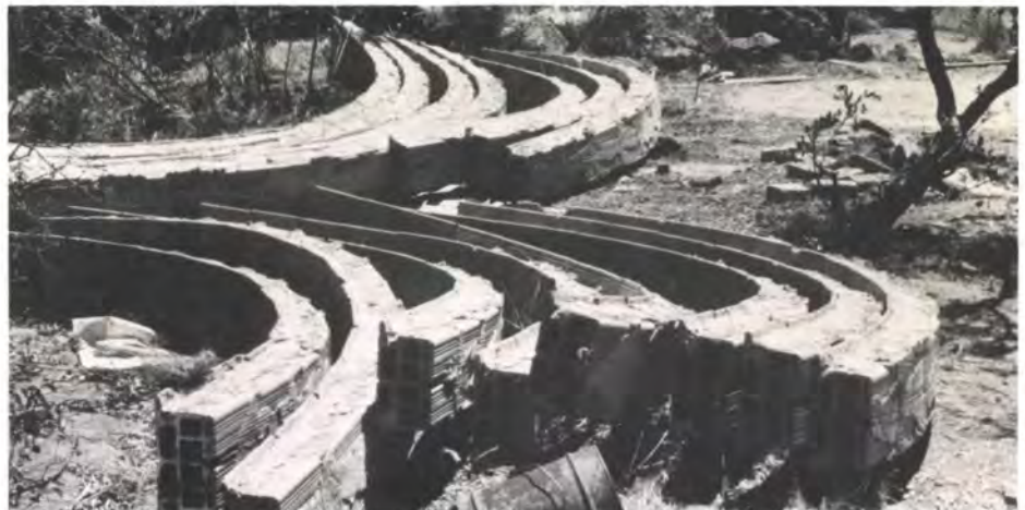
Fig. 4b Cullinans: prefabricated units (Photo: Ove Arup & Partners, Zimbabwe)
