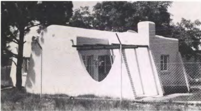
Fig. 5a Complete low-cost two-bedroom house without parapets : 3m span (Photo : Ove Arup & Partners, Zimbabwe)
