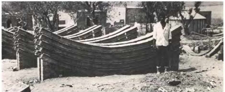
Fig. 4a Chobe, Botswana: prefabricated units (Photo: Ove Arup & Partners, Zimbabwe)
