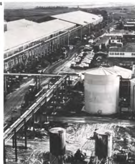
Figs. 4-5 Main fibre production, spinning plant, pipe racks, main access road, chemical store for water treatment
