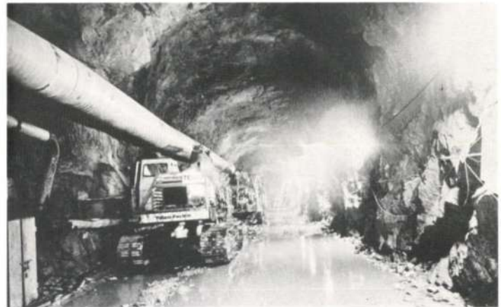
Fig. 18 The tunnel excavation
