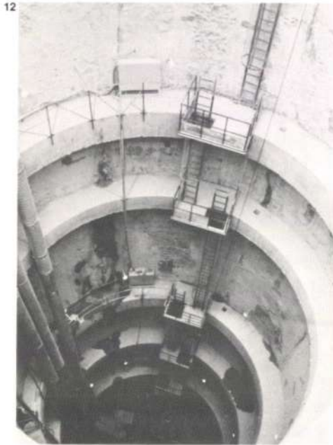
Fig. 11 Shaft No 2: The start of excavation
