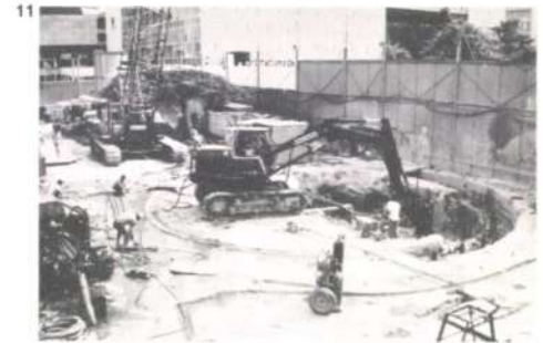
Fig. 13 Excavation of a top heading in the tunnel
