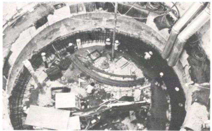
Fig. 11 Shaft No 2: The start of excavation
