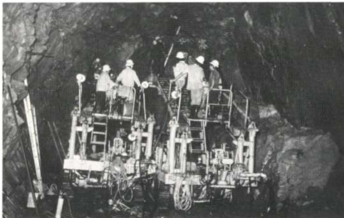
Fig. 16 Drill jumbos in the tunnel
