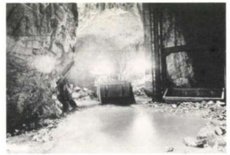
Fig. 17 LHD and muck skip at the base of Shaft No 2
