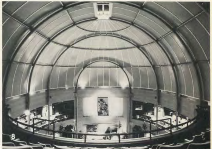
Fig. 5 Completing the inside of the Great Hall dome. The rising floor is in the 'up' position; dark areas on the roof show where the blackout system of liquid-filled panels has been installed. The liquid turns opaque on the application of heat, either electrical or natural.
