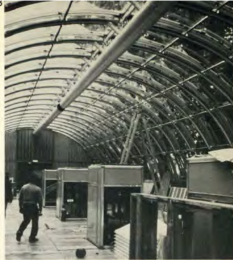
Fig.17 Arch components in the factory during fabrication (Photo: Robert Kinch)
