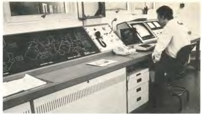
Fig.7 Security control console showing the mimics on the left and the VDU in front of the security offices (Photo: Bob Wood)
