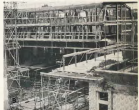
Fig. 5 Completing the inside of the Great Hall dome. The rising floor is in the 'up' position; dark areas on the roof show where the blackout system of liquid-filled panels has been installed. The liquid turns opaque on the application of heat, either electrical or natural.
