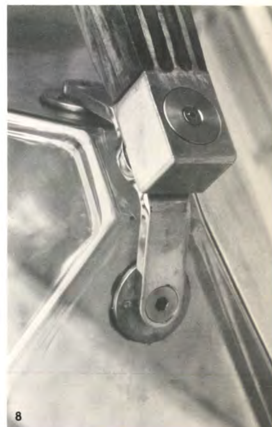
Fig.8 Bottom joint between external timber and pyramid (Photo: the architect)
