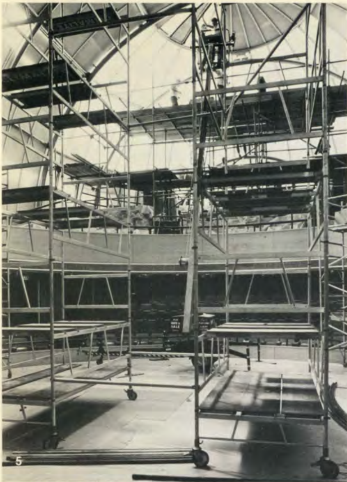
Fig. 5 Completing the inside of the Great Hall dome. The rising floor is in the 'up' position; dark areas on the roof show where the blackout system of liquid-filled panels has been installed. The liquid turns opaque on the application of heat, either electrical or natural.
