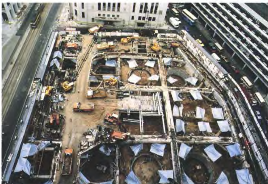
Fig. 16 Access caisson excavation (Photo: The Hongkong Bank)
