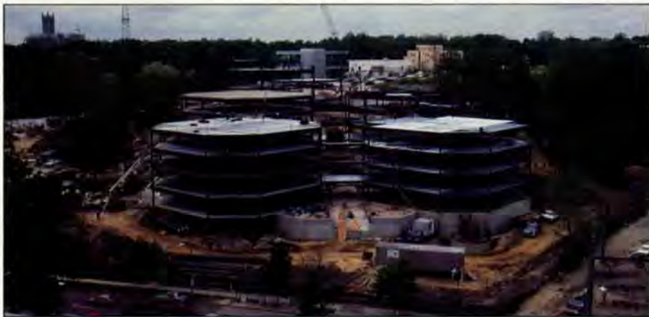
5. Connecticut Avenue elevation during construction (Photo: Bill Thomas)
