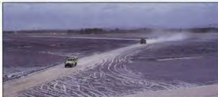
4. Terminal and car park area: after reclamation, before construction
