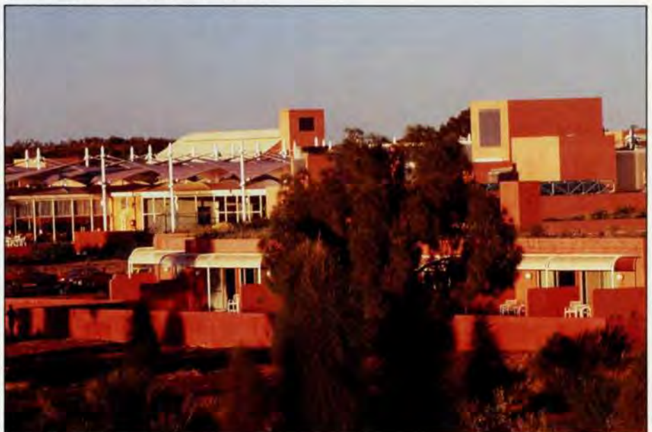
Sheraton Hotel rooms and central facilities
