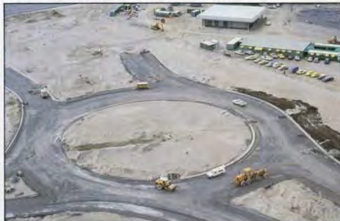
5. Roundabout under construction
