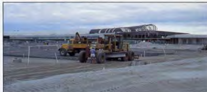
6. Subgrade trim and sub-base laying
