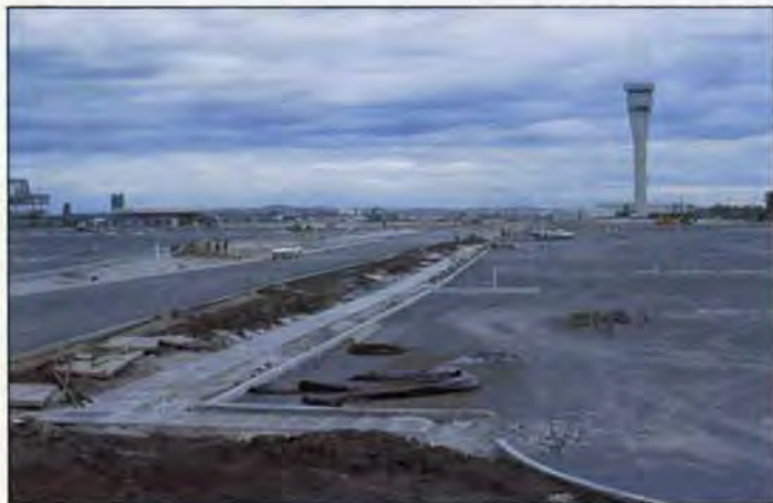
3. Car park and internal access roads under construction
