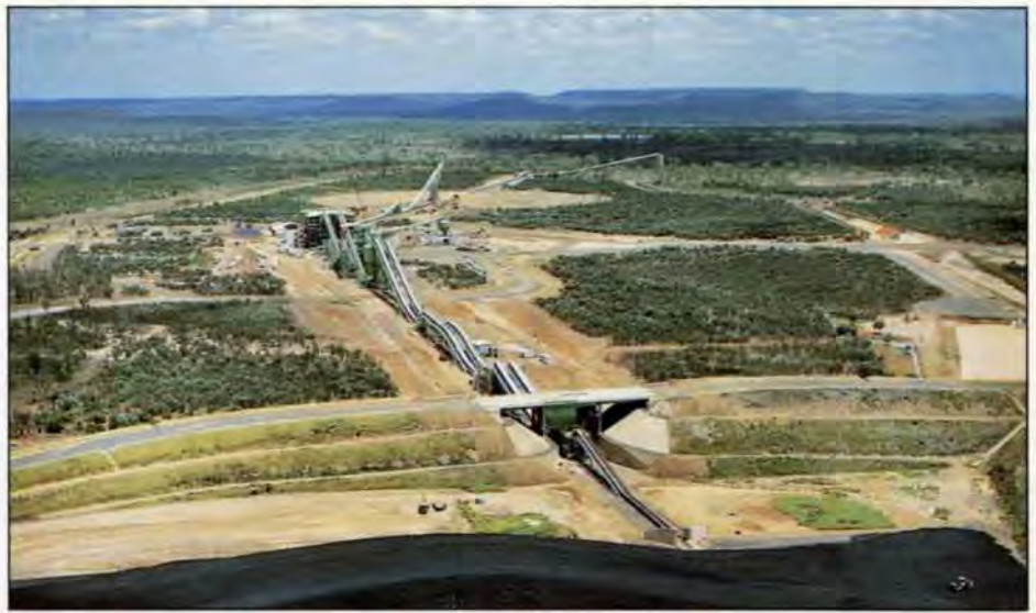
4. Coal preparation plant
