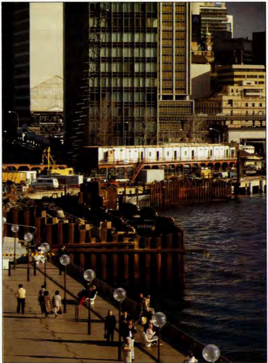
13. Construction in July 1986 (photo: John Nutt)
