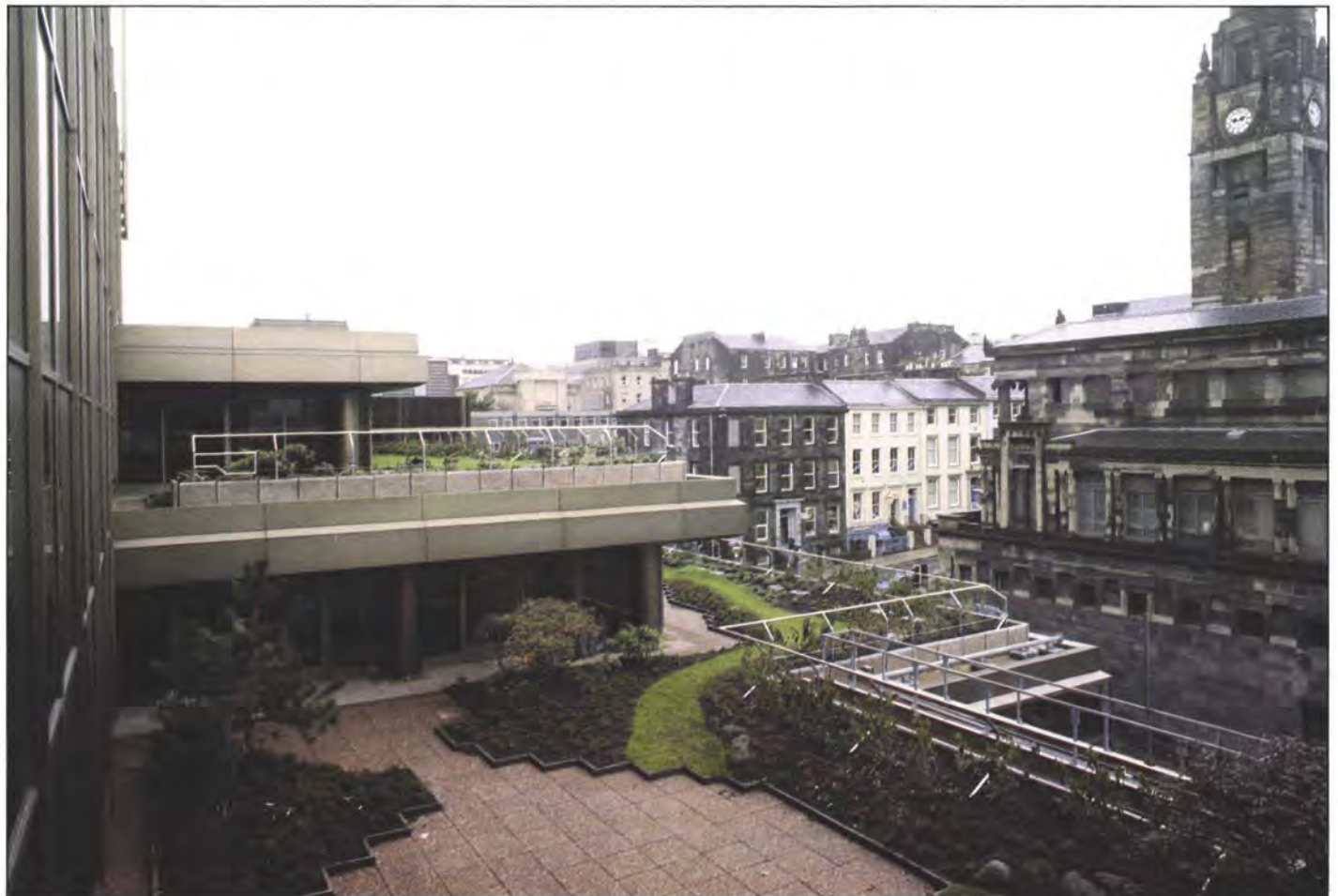
Landscaped roof terraces (north east) (Photos: Guthrie Photography)
