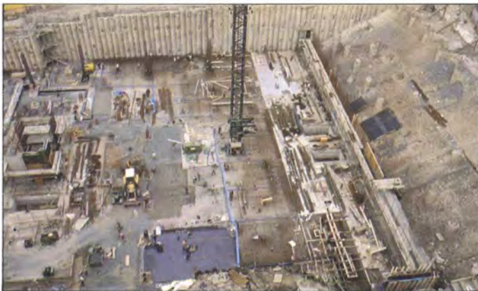
Deep excavation at east end
