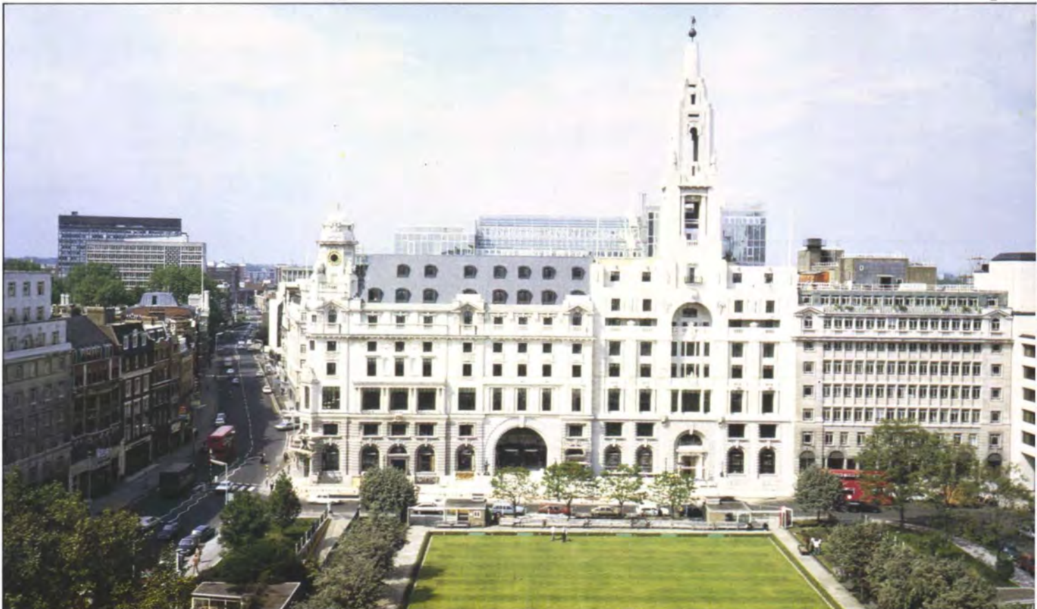
2. Triton Court viewed from Finsbury Square
