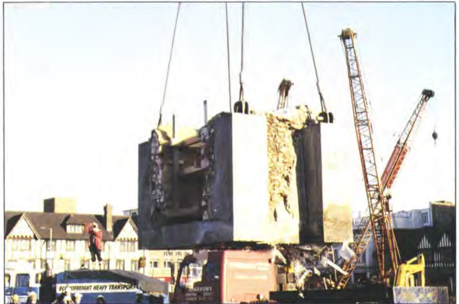
11. The stair section aloft (Photo: Ian McVitty)
