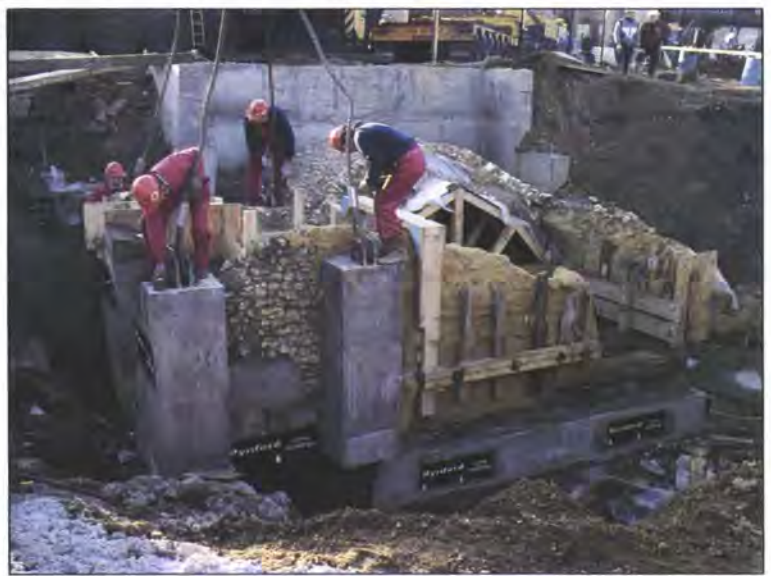
10. Cables being attached to stair section (Photo: Peter Benson)
