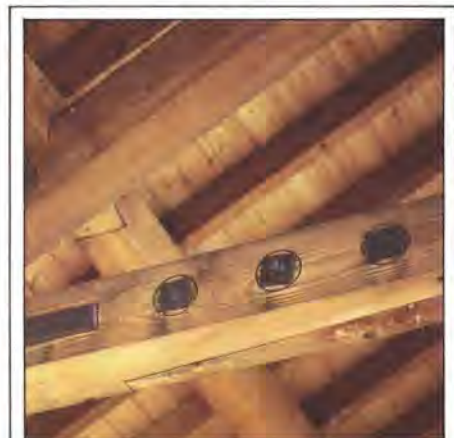
9. Truss repair (Photo: Peter Mackinven)
