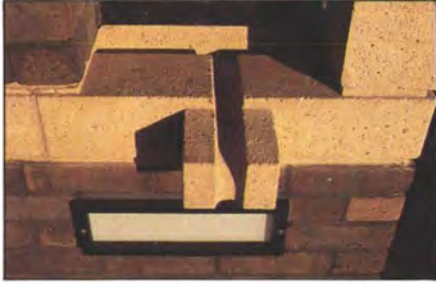
7. Precast unit with gutter and gargoyle
