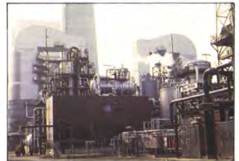
2. Voerde Power Station, West Germany, showing limestone gypsum FGD installation in foreground (Photo: Malcolm Noyce)
