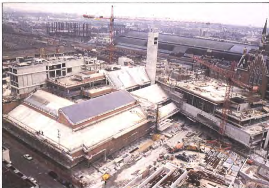
Phase 1A structure: SRL half completed
