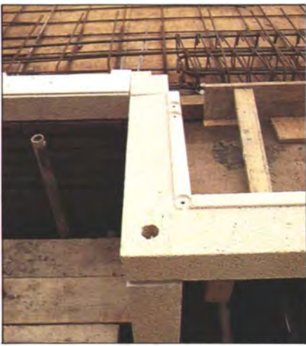
6. Precast unit in place prior to casting slab
