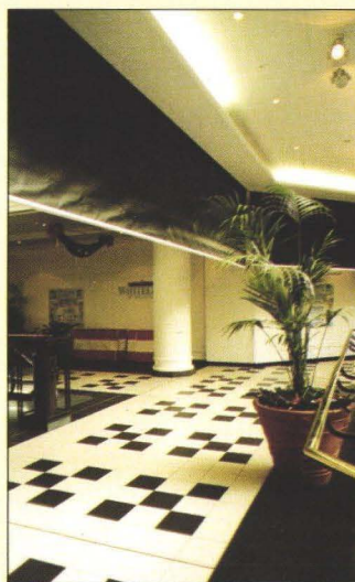
Smoke curtain fully deployed on atrium floor. (Photo: Roger Olsen)
