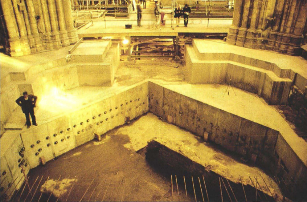
2. York Minster: concrete extensions to tower foundations.
