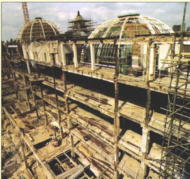
Above: Rear bay of the Belcher building after demolition works.
