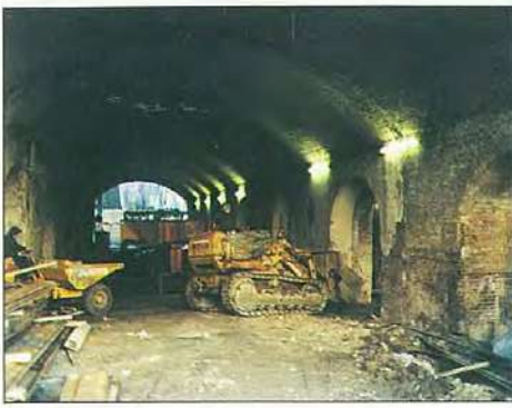
18. View of the brick vaults beneath the station during construction.
