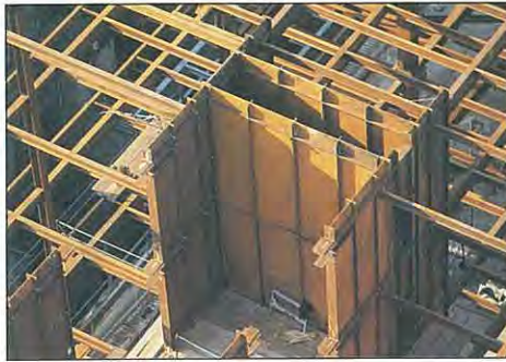
11. Part of the steel plate core.
