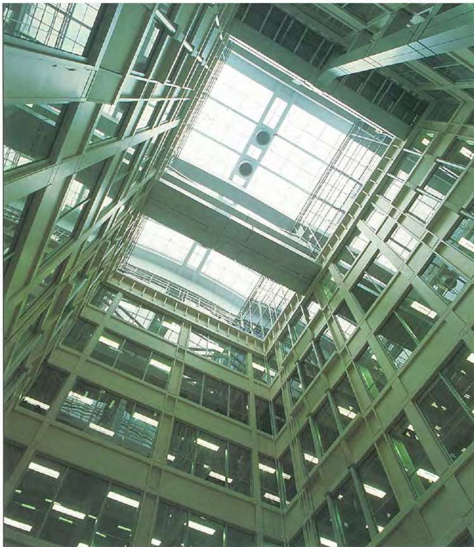
25. Inside a completed atrium.
