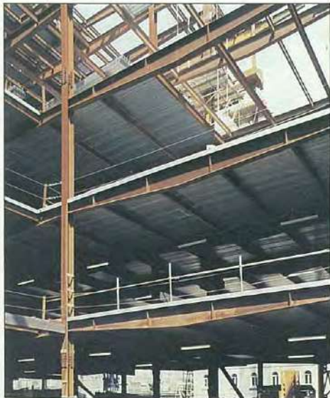
23. Tapered beams at the edge of the atrium.
