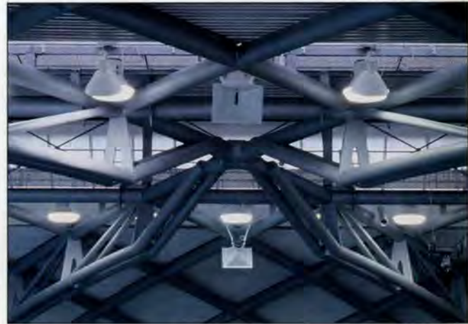
7. right: Crown of pool hall roof.
