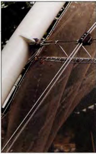
4. Showing cable cross-over clamp, cable connection to arch and hanger bar system which connects cable net to mesh panels.
