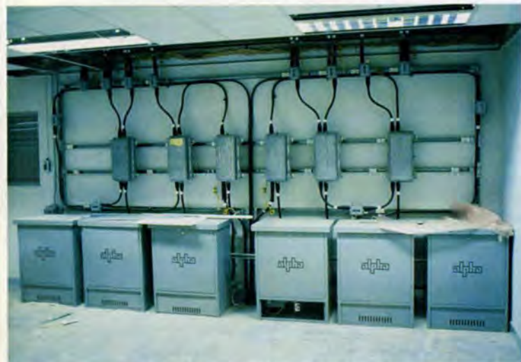
3. Toyota broadband installation. (Photo: Ove Arup & Partners)
