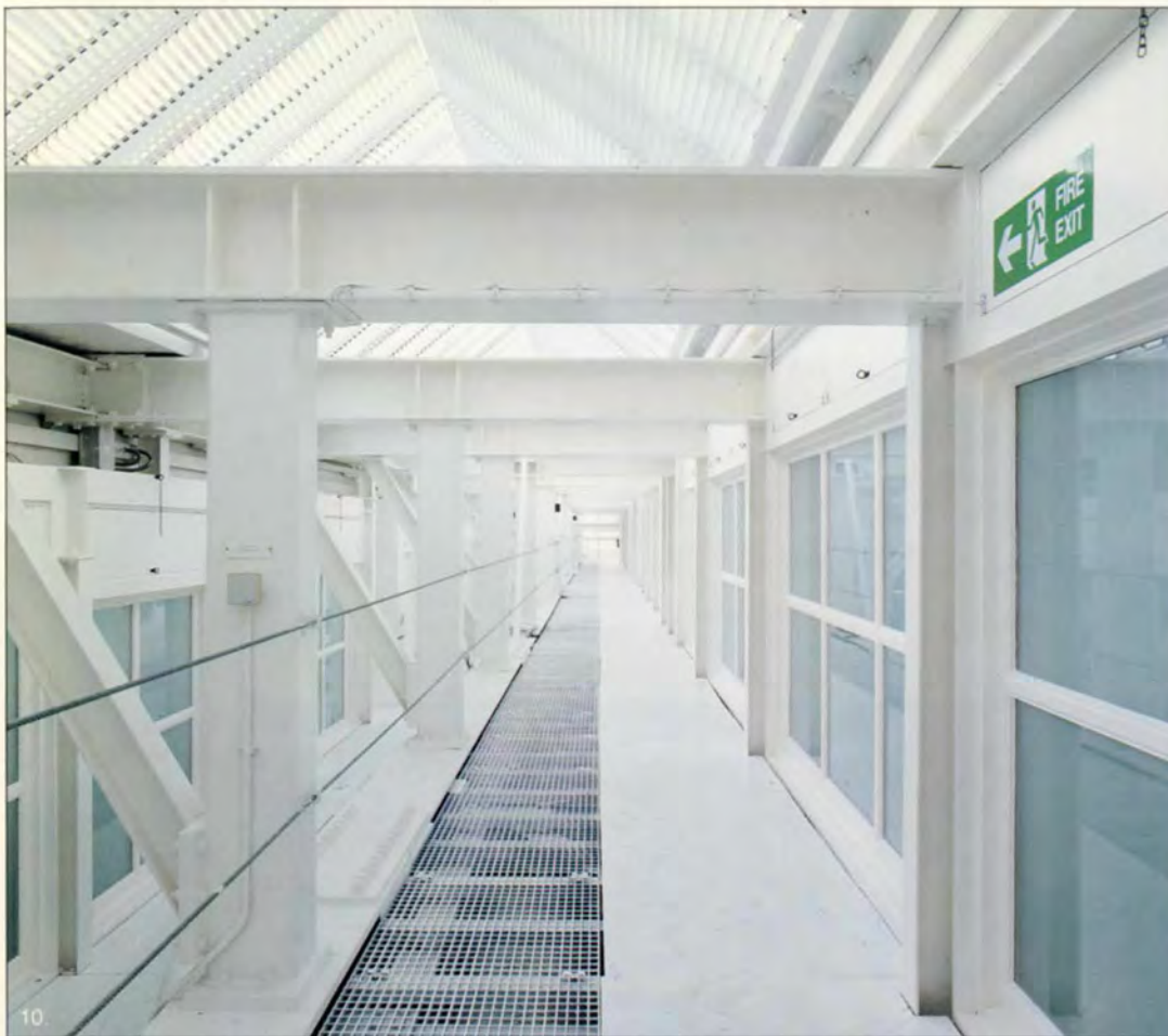
10. Clerestory glazing showing natural lighting control mechanism.
