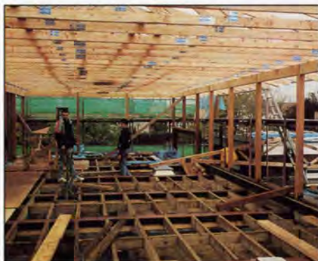
1. The new timber frame under construction.
