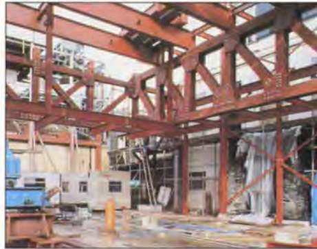
7. Steelwork transfer girders for cineplex.
