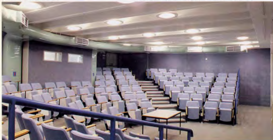
△ 11. Clinical lecture theatre: note exposed structure and services.
