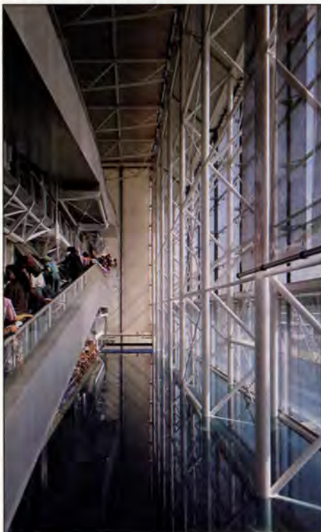
5. Travelators and east wall.
