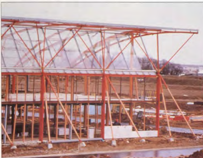
5. Right: Placing the inner cladding deck.
