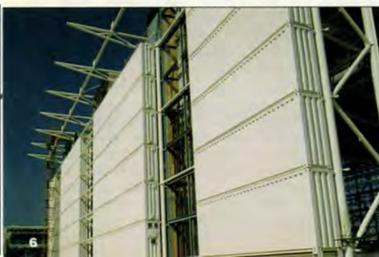
15. West tank wall, made up of mini-containers.
