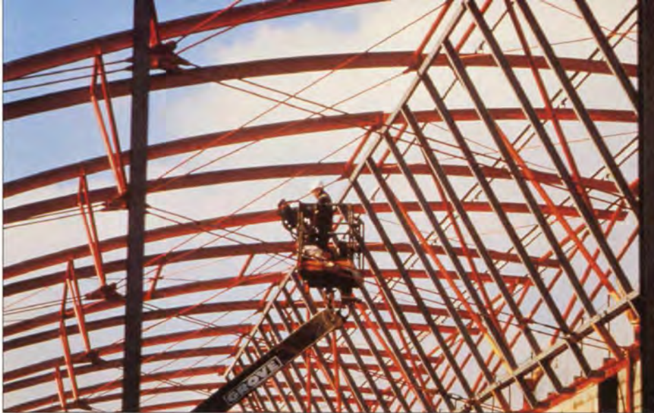
6. Installation of ties.
