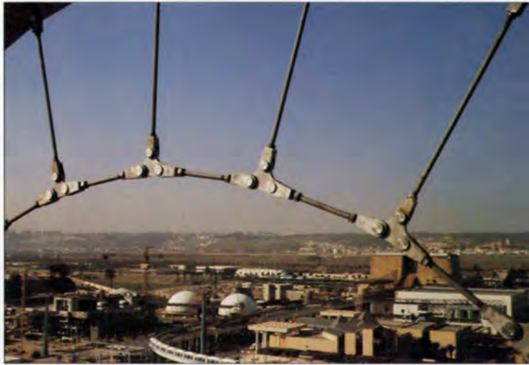
2. Steel components in tension ring inside arch. ▶
