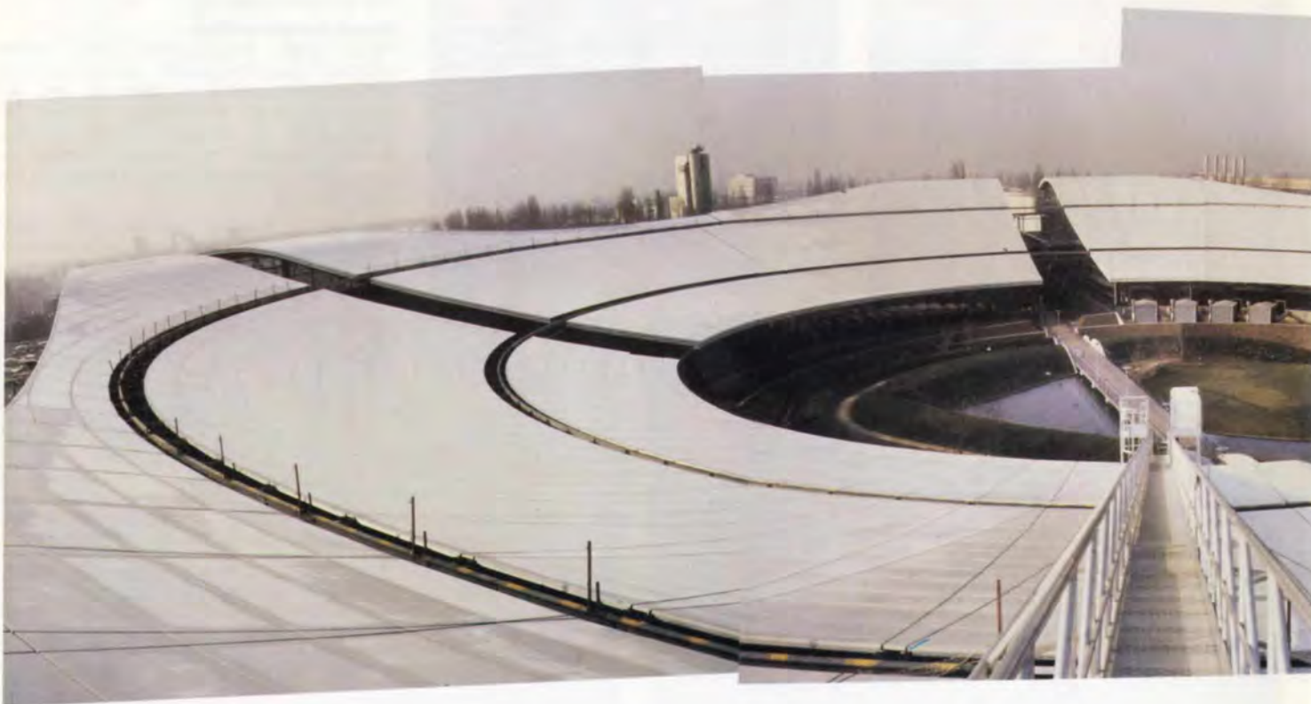
10. Roof nearing completion (panels at cleaning cradle tracks yet to be installed).
