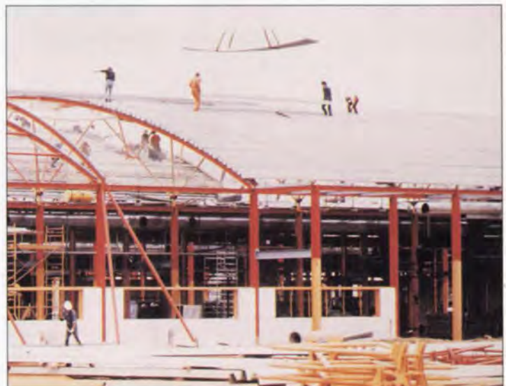
5. Right: Placing the inner cladding deck.
