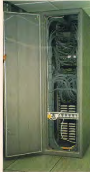
B. Rear of cabinet for structured cabling termination patch panel.
