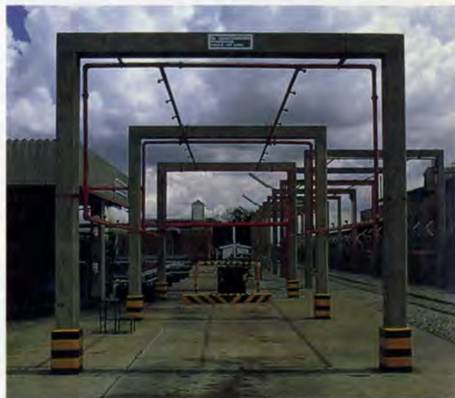
▼ 8. Sprinkler support portals, LPG decanting area.
