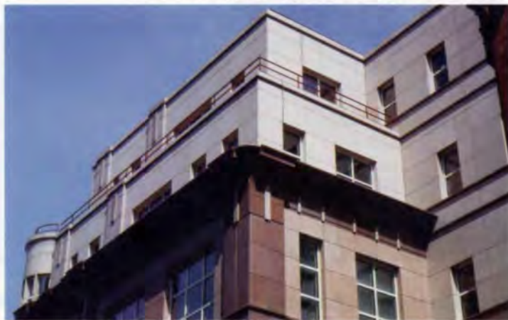
4. North-west corner new buildings, showing stepping of façade and colours.
