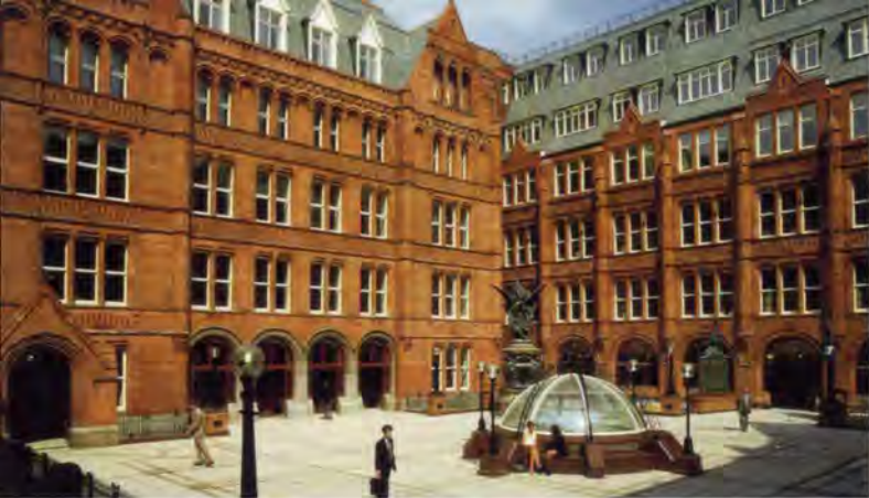
9. The central courtyard.
