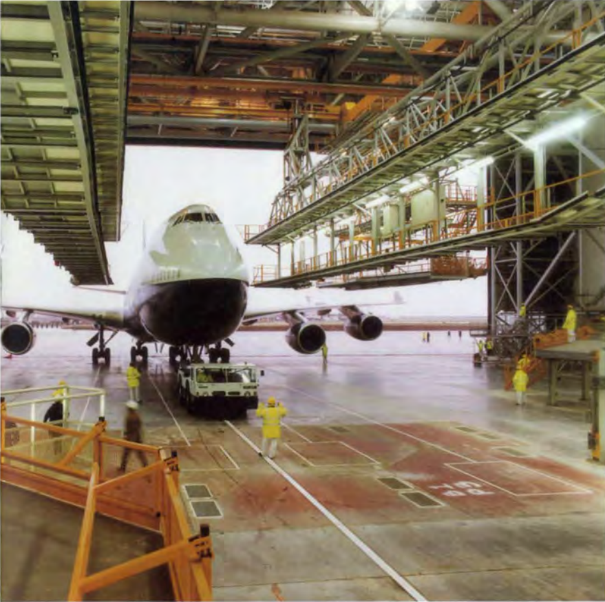
◀ C. Aircraft City of Cardiff entering the hangar during construction for access docking trial fit.
