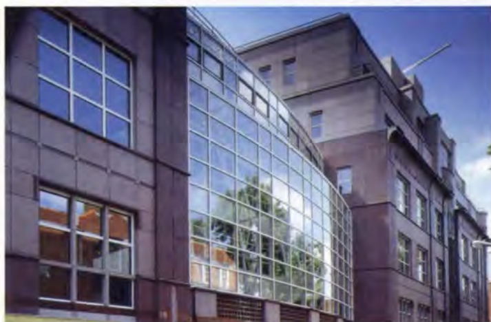
15: North elevation with conservatory stepped to preserve rights of light for existing residential building opposite.
