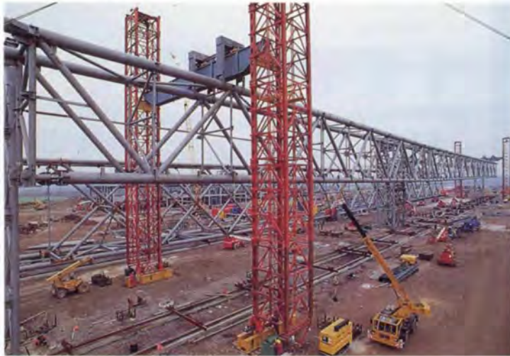
7. 600 tonne door girder lift, January 1992.
