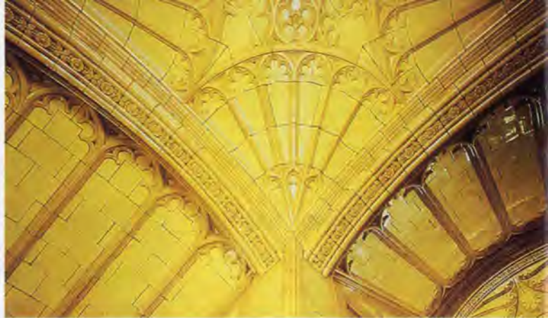
10. Faience roof in the Flagship.
