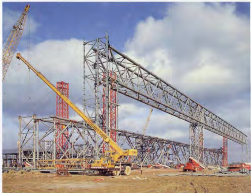
8. Door girder fully erected, 1000 tonne spine girder awaiting lift, February 1992.
