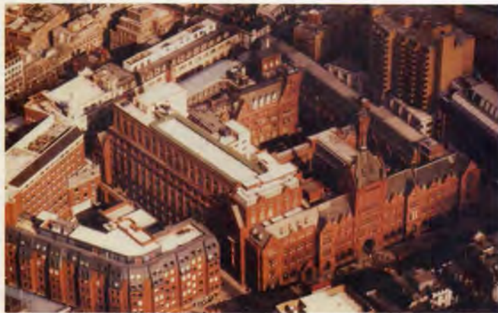
3. The site from the south-west, before redevelopment.
