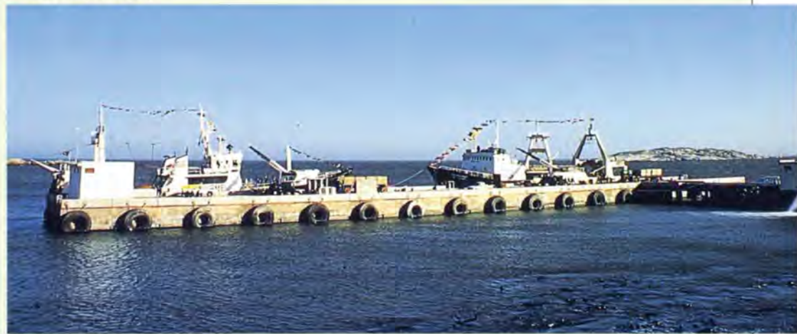
C. The completed jetty.
