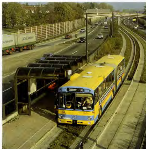
2. Guided busway in Essen.
