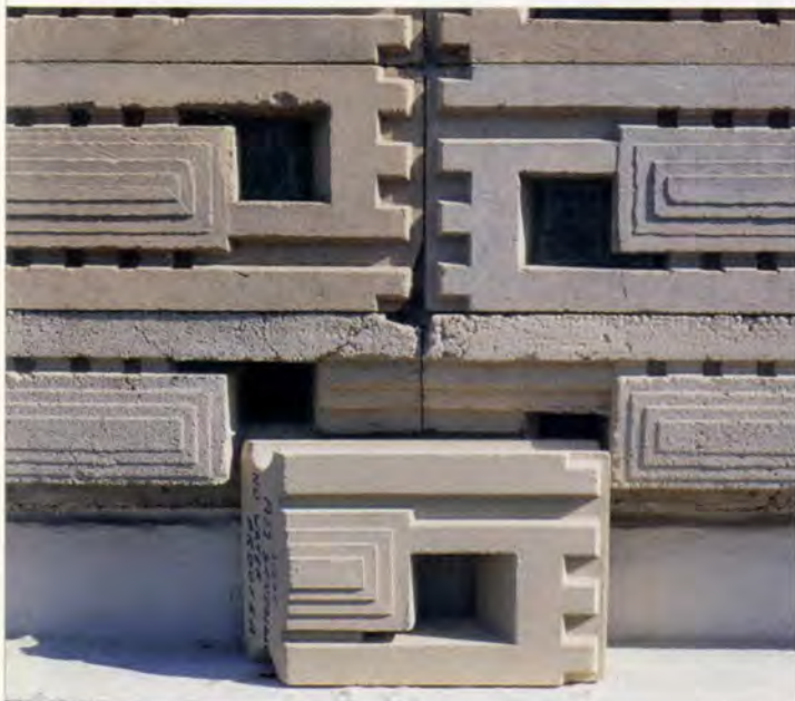
8. Use of chevron corner blocks and insufficient movement joints has caused unsightly cracking, allowing water ingress.
