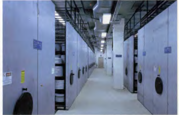
15. Medium-term storage vault, showing shelving/structure/services.
