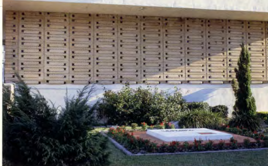
5. Annie Pfeiffer Chapel is constructed of structural reinforced concrete with 'textile' block infill walls.
