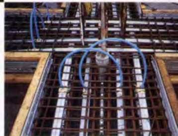
6. Post-tensioned beams: intersection detail.
