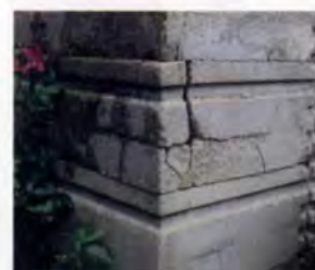
8. Use of chevron corner blocks and insufficient movement joints has caused unsightly cracking, allowing water ingress.
