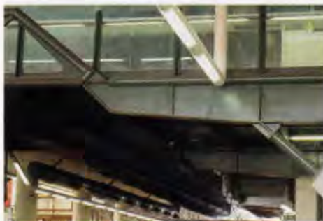
Cantilevered main beam on Mezzanine Bridge.
