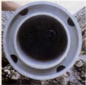
11. Section through polypropylene process sewer.
