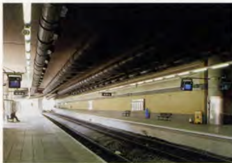
8. Platforms 5 and 6 central with exhaust ventilation ducting above.
