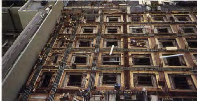
5. Second process building showing the post-tensioned beams and the beam-and-column structure in the open or reserve section.
