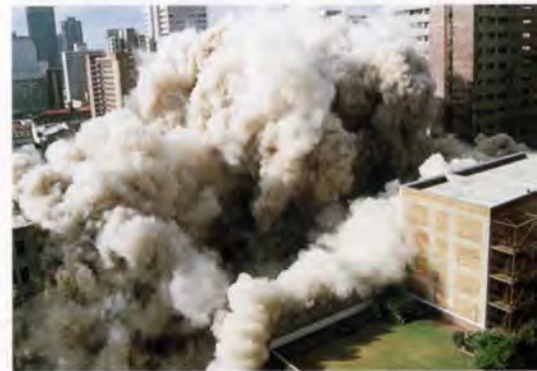
6. Five buildings demolished by one implosion.
