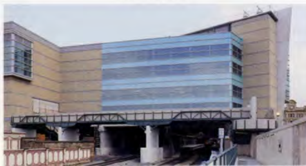
4. The West Bridge with platforms in background below and office building for Arena above.
