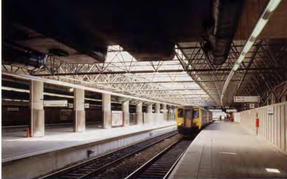
Platforms 3 and 4 west, with new canopy and exhaust ventilation systems above.
