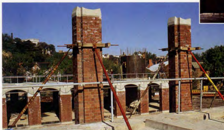
7. Brick piers ready for floor units.
