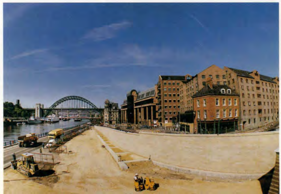
12. Below: Completed retaining wall A, September 1993.
