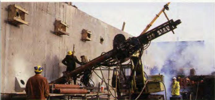
16. Retaining wall D - installation of ground anchors, January 1994.
