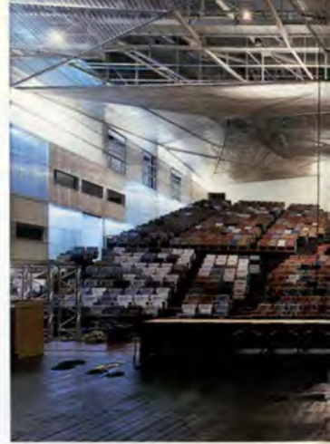
13. Above: Interior of 1500-place lecture theatre, showing transparent articulating suspended acoustic ceiling.
