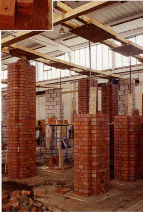
4. Brick piers under construction.
