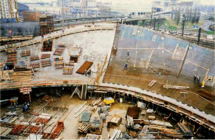
9. Above: Warped gallery floor slab under construction: one half cast, one half decked out with formwork.
