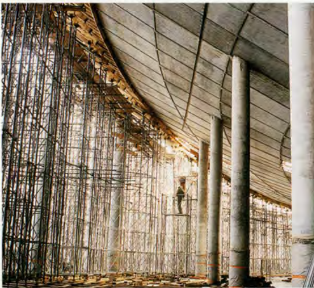
10. Below: Striking the gallery floor slab to reveal the formwork pattern.
