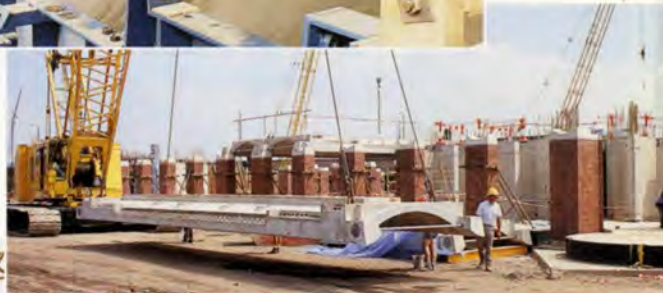
10. Lifting a floor unit.
