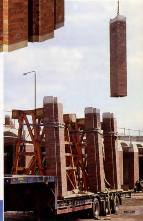
6. Lifting a brick pier.
