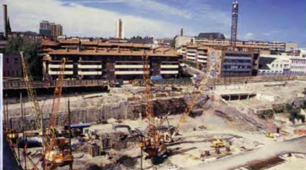
13. Left: Retaining wall B - Reinforcement cage, September 1993
