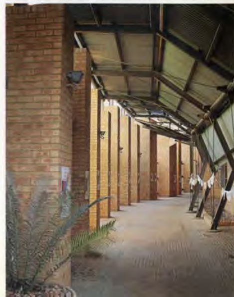
5. Covered walkway on south side of building.
