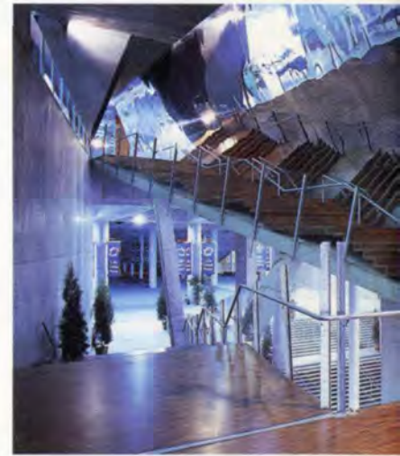
5. Above: The overlapping ramped main staircase of Congrès, enclosed by inclined stainless steel clad walls.
