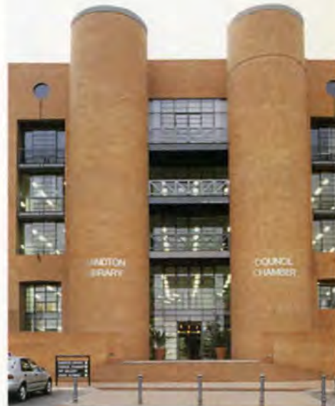
4. East elevation entrance from the forum, showing cylindrical stair and lift cores.
