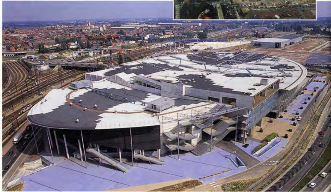
1. Aerial view to the south, with inset 2. showing the Lille Grand Palais in the foreground, and the Euralille commercial centre and TGV station beyond.
