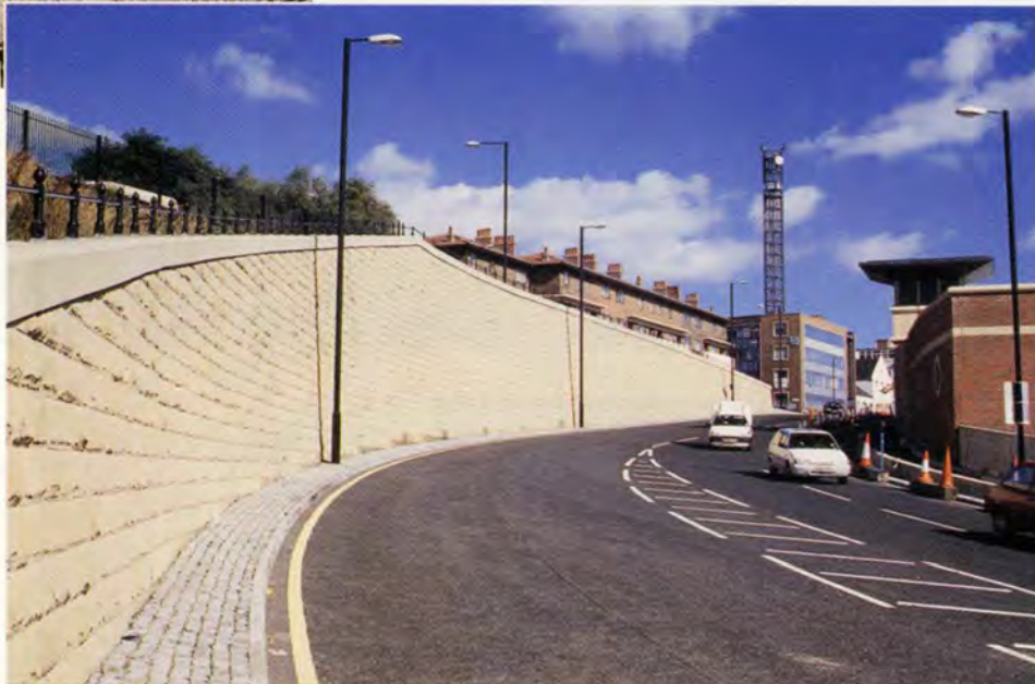
15. Below: Retaining wall K completed, September 1995.
