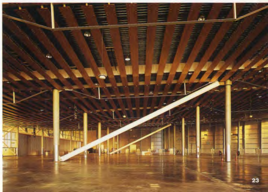
27. Right: General interior view of roof structure, showing composite timber trusses, supported on steel tie beams, with tubular columns serving displacement ventilation at low level. Diagonal bracing for stability was architecturally required to be expressed in the interior.
