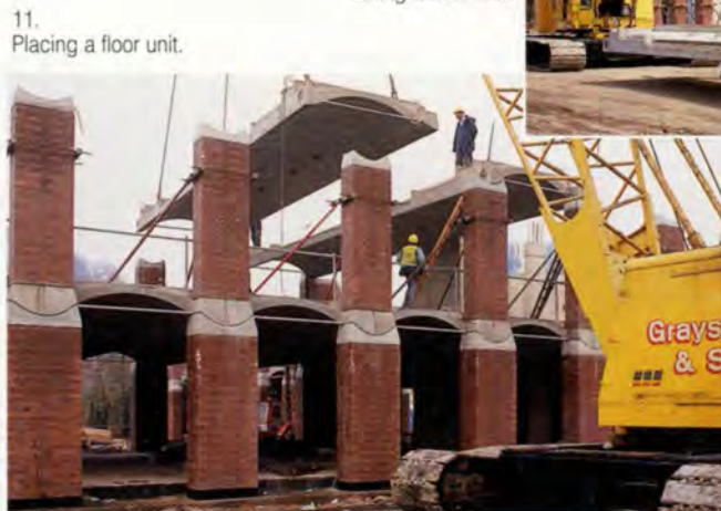
10. Lifting a floor unit.
