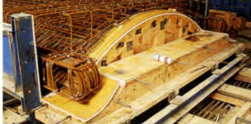
8. Timber mould for ends of units.
