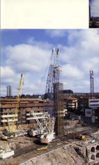
13. Left: Retaining wall B - Reinforcement cage, September 1993
