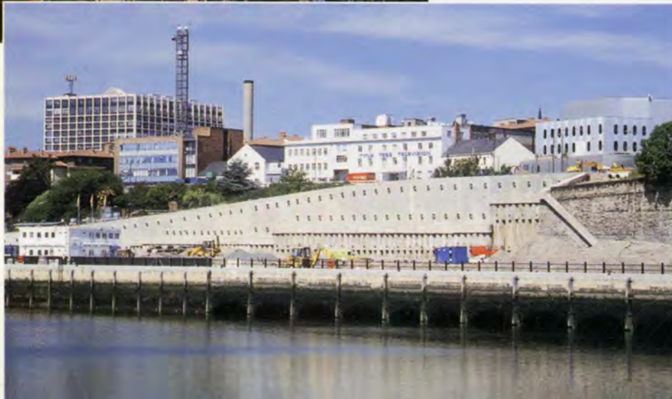
17. Completed retaining wall D, June 1995.
