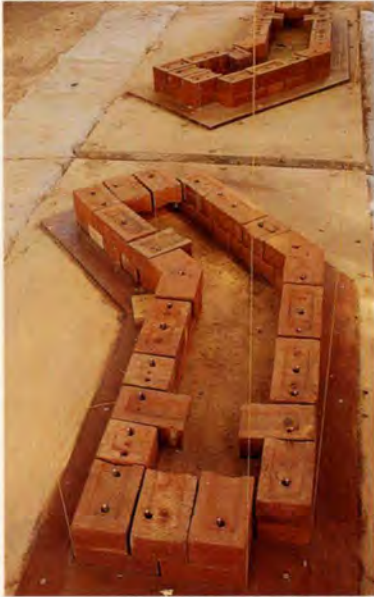
3. Base for preformed brick pier.
