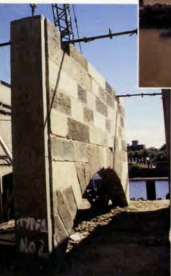
6. Left: Precast stone-clad arched panel, June 1994.
