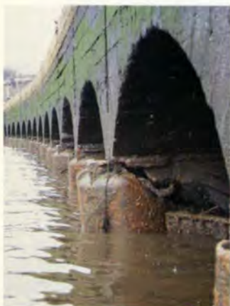
4. Quaywall - existing structure, February 1993.
