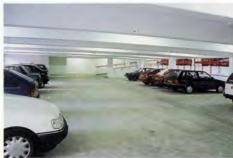
19. Interior of Phase 1 car park.
