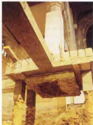
9. Underside of pier.
