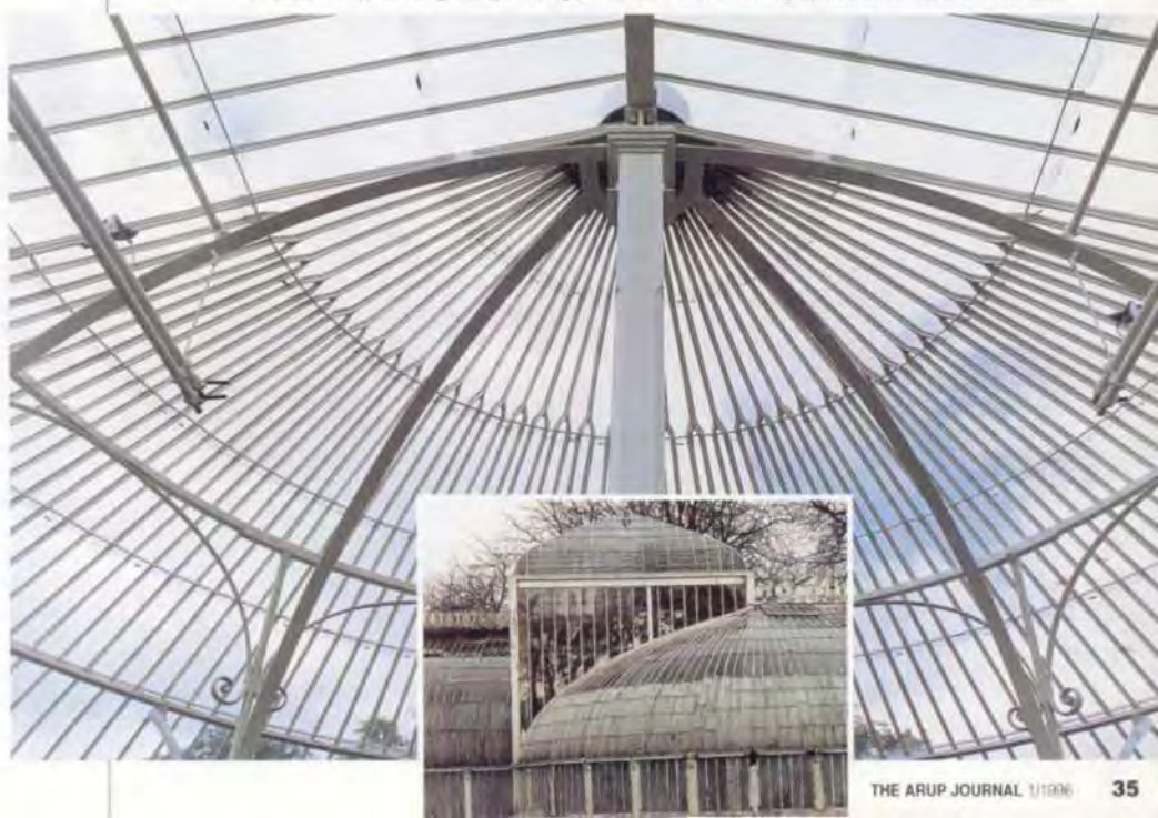
1. Restored spherical glazing in wings, with 2. (inset) Showing appearance before restoration.
