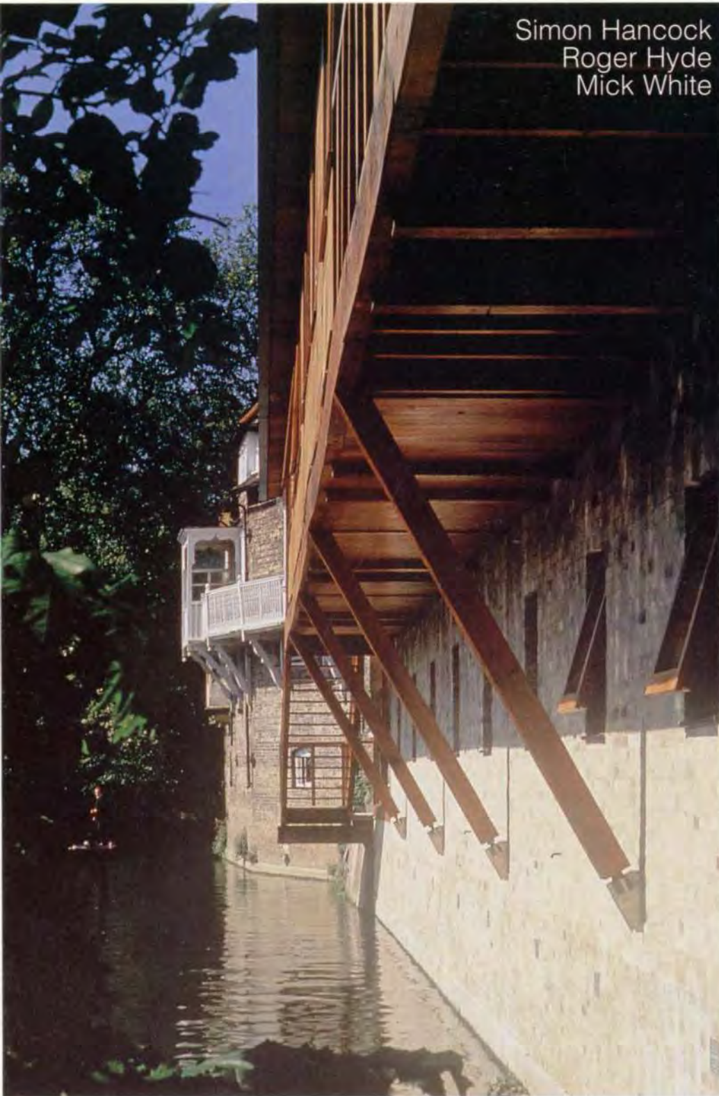
1. Darwin College: Oak beams support the cantilevered study area over the River.
