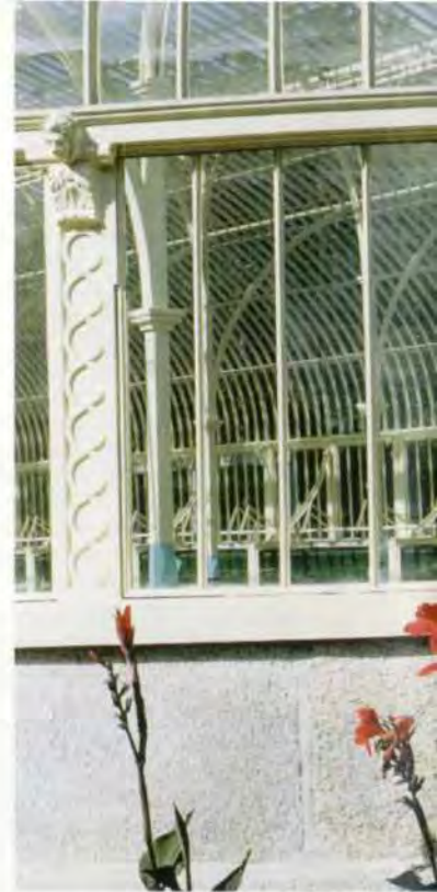
4. Pilasters, gutters and sashes in wings.
