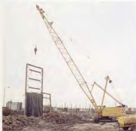
5. Lowering HDPE membrane into wall.
