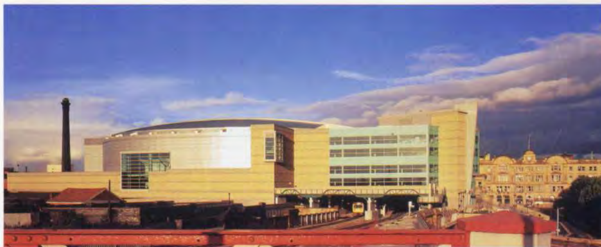
4. Elevation of completed Nynex Arena (left) adjoining Arena Point office block.
