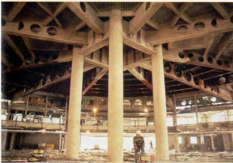
12. The four circular steel columns supporting the drum.
