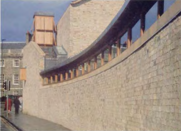
5. The study area, showing oak timber structure and 'stable' doors giving natural ventilation.
