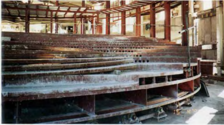
10. The auditorium under construction: the rail supporting one of the rotatable units is visible in the foreground.
