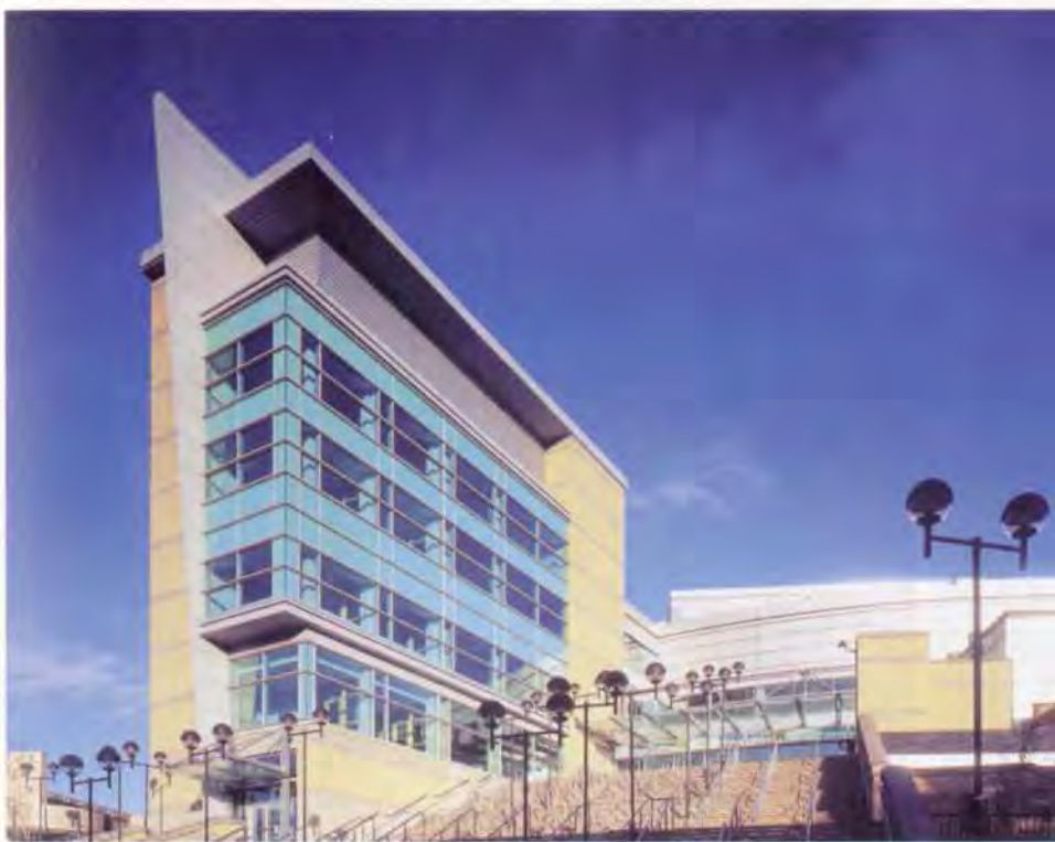
10. Arena Point office building.
