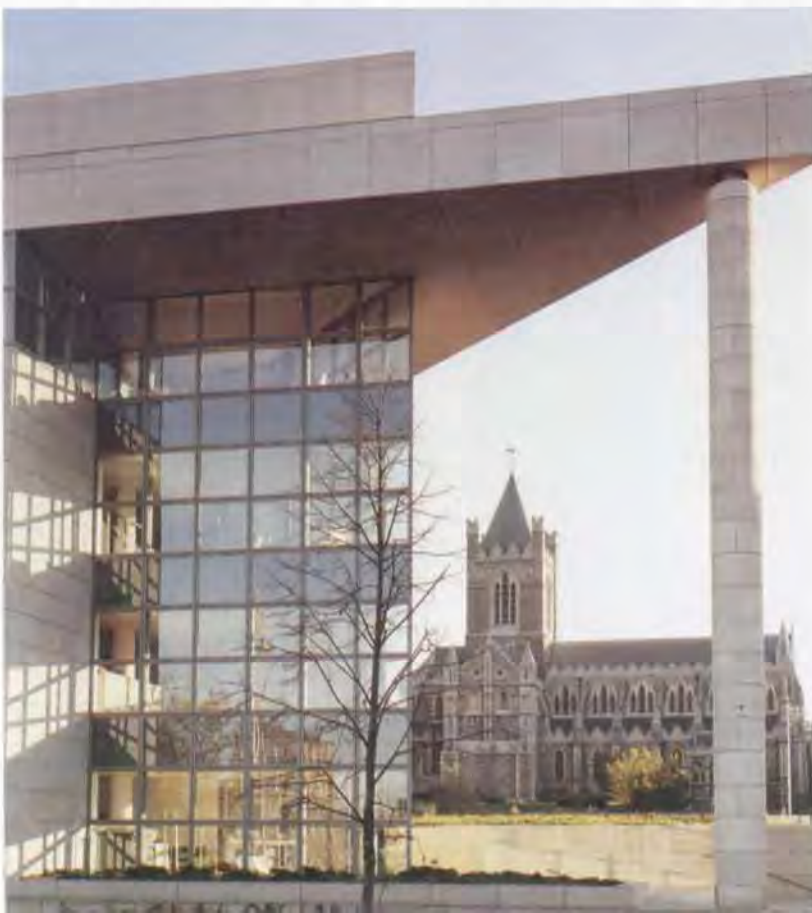
3. North-west corner of Block 4, with Christ Church Cathedral in the distance
