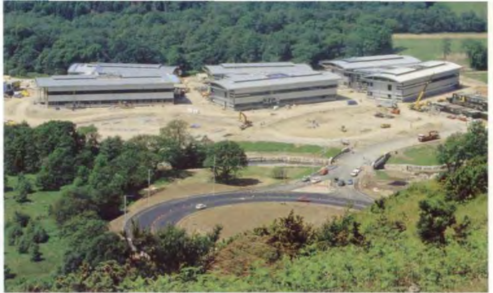
1. The site during construction.
