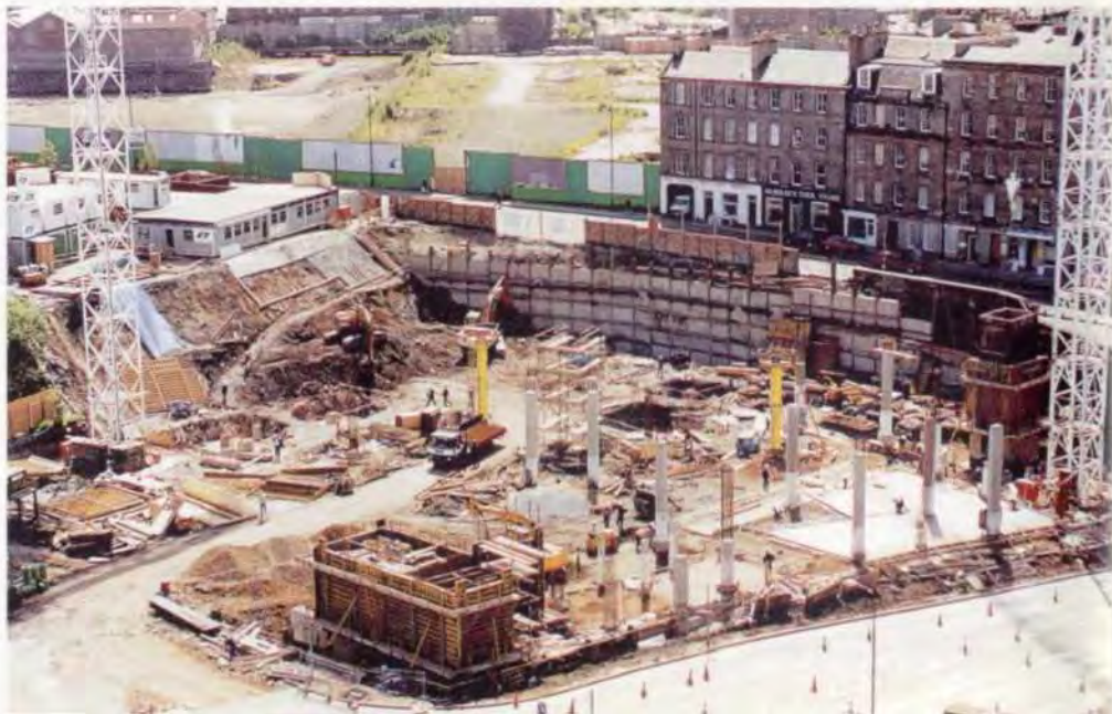
3. The site in May 1993, facing south-east, showing the temporary retaining wall to Morrison Street.
