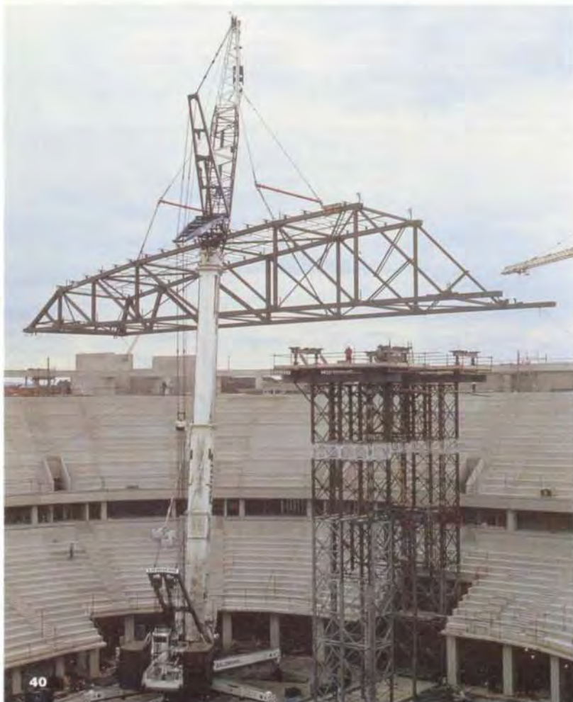
8. Roof truss lift.
