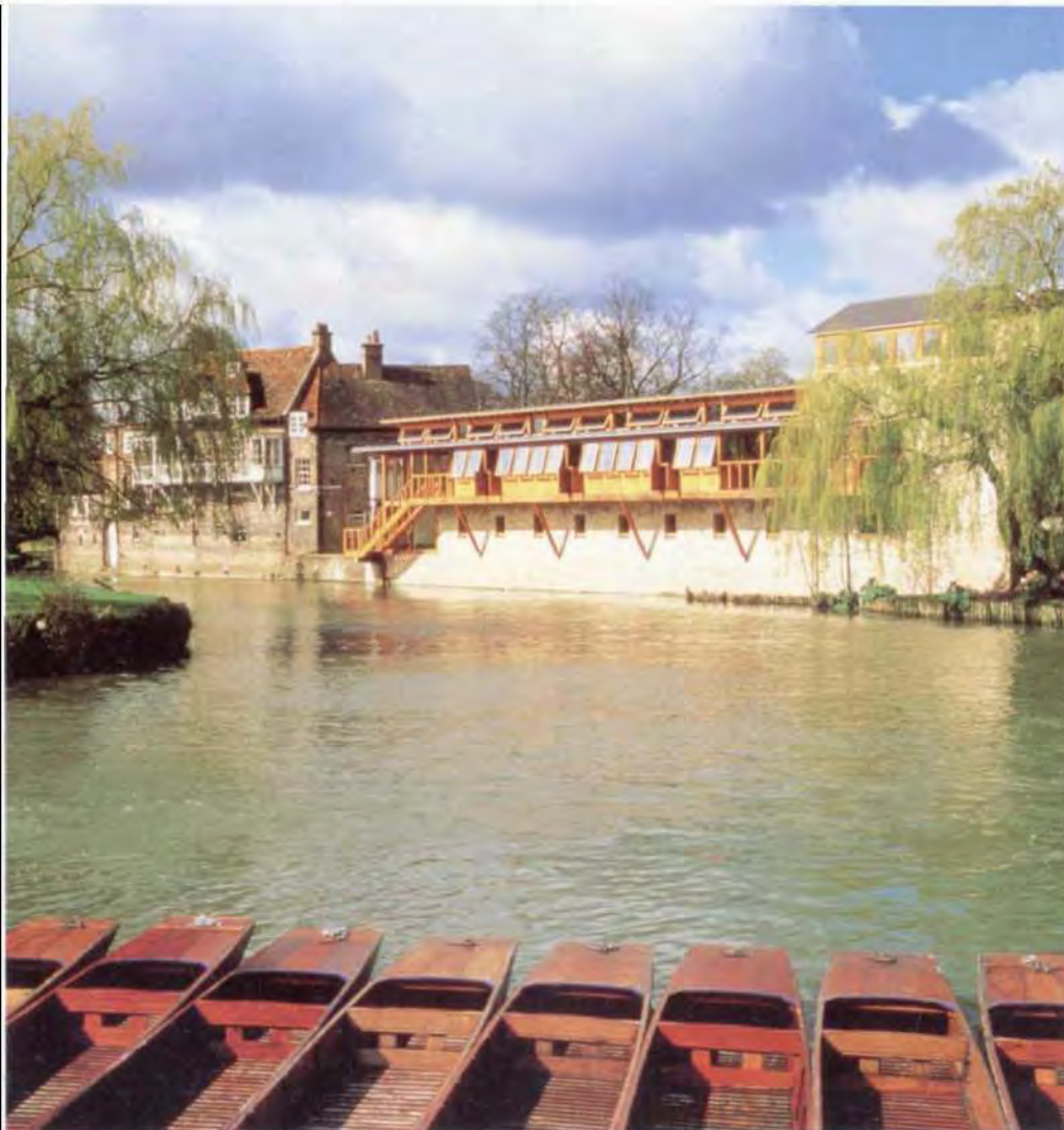
8. The completed building in its riverside setting.
