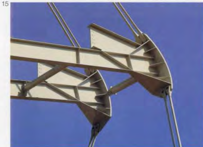
15, 16. Bracing element and A-frame, as built.
