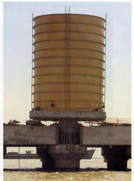
17. Preloading tank on precast deck.
