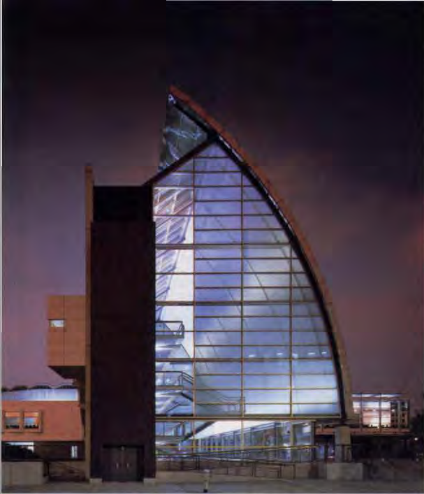
4. West elevation of Hall of Fame at night. The upper end of the exterior elevator is on the left.
