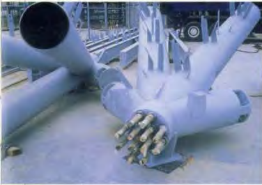
F. End of bowstring truss showing 12 Y50 reinforcing bars threaded through bottom chord.
