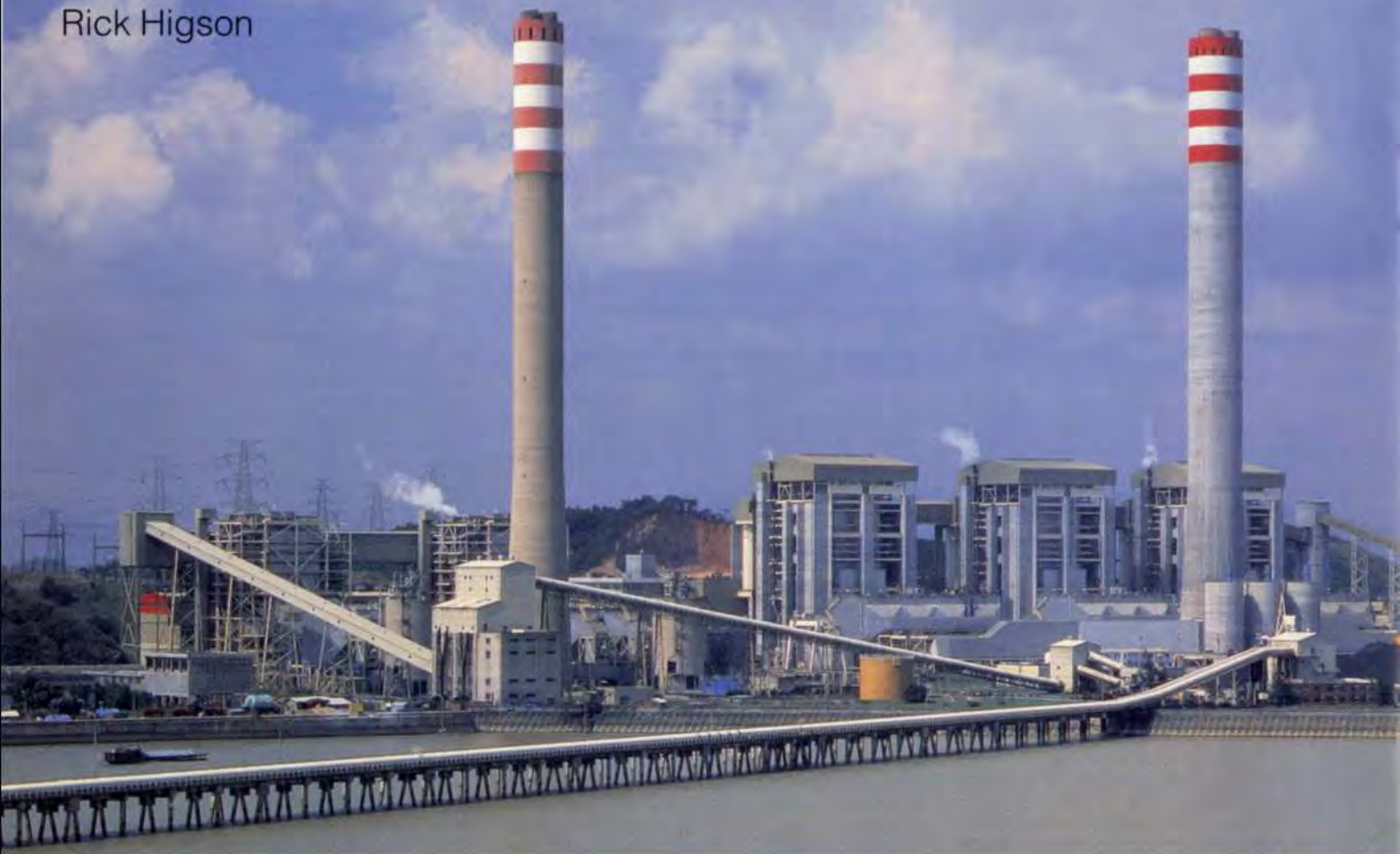
1. Left to right: the two 350MW units and 210m chimney of Shajiao B, and three 660MW units and 240m chimney of Shajiao C;
