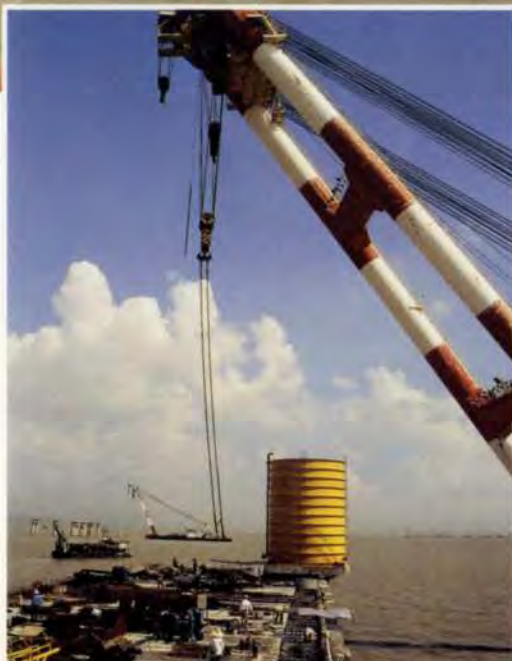
16. Placing caisson preloading tank, and in situ deck construction, August, 1994.
