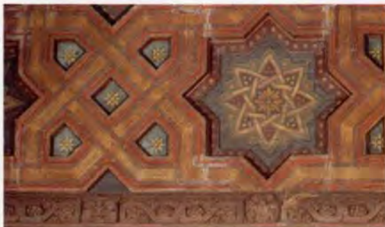
2. Reference Room painted cast plaster ceiling: pre-earthquake.
