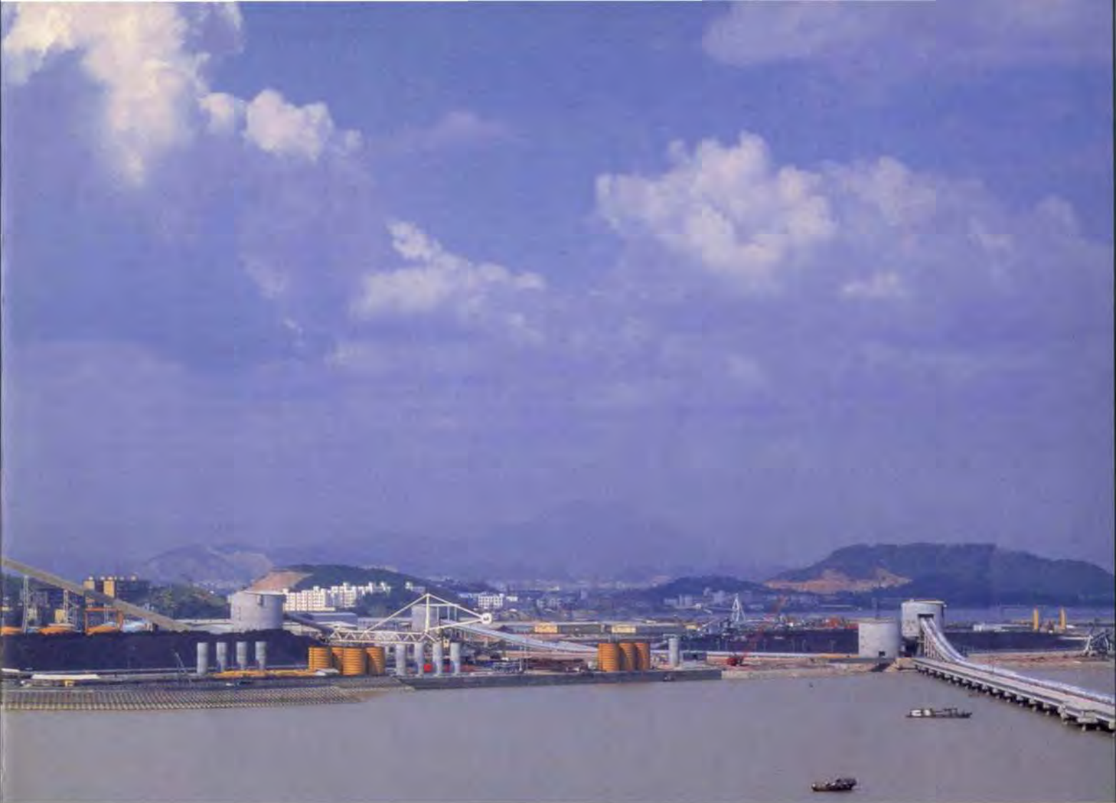
Shajiao B jetty access arm left foreground, Shajiao C jetty access arm extreme right. (photograph taken from Shajiao C jetty)
