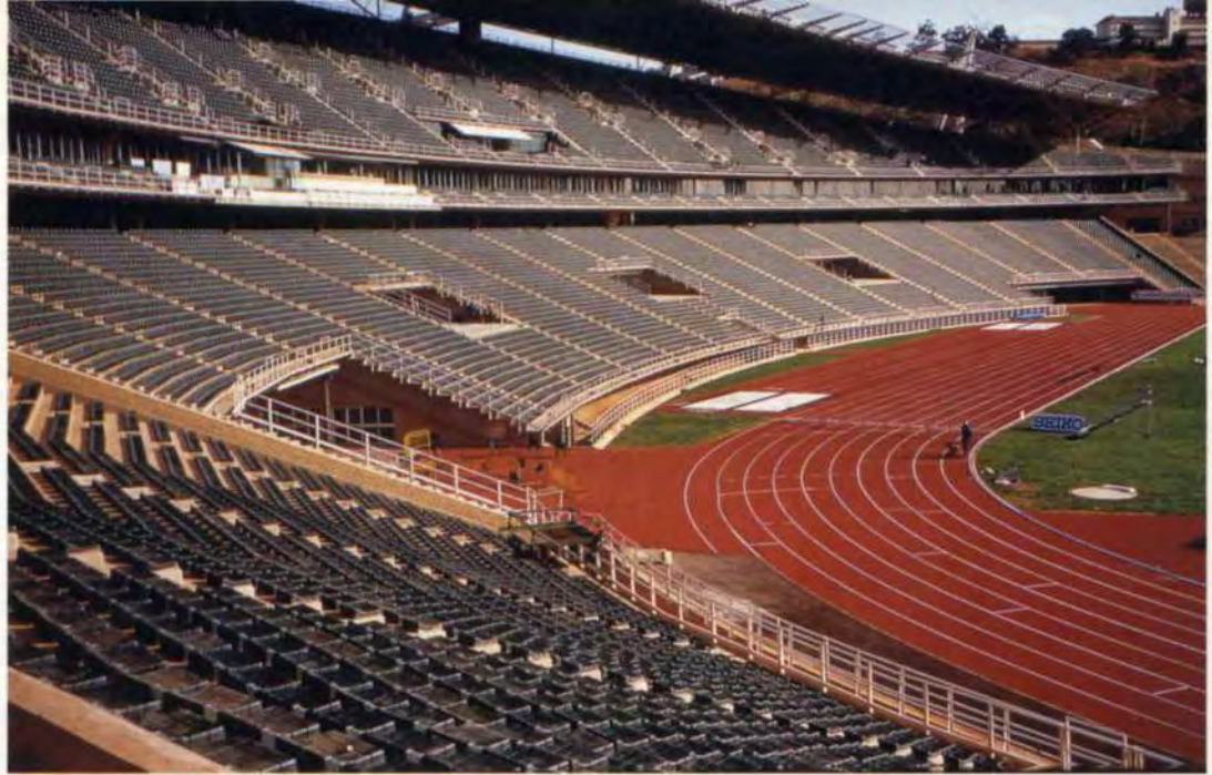
17. Completed interior of the stadium, showing wide pre- and post-event vomitories and (Left to right, mid-way up the lower bowl) the three dedicated terrace areas for media, VIPs, and officials.
