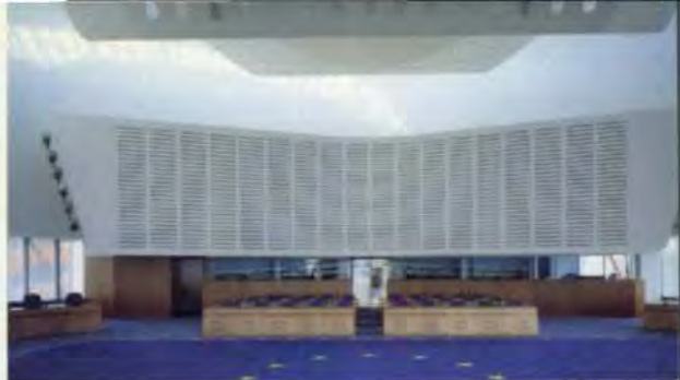
E. Interpreters' booths in the Commission Room. The perforated acoustic panel conceals the air handling plantroom.
