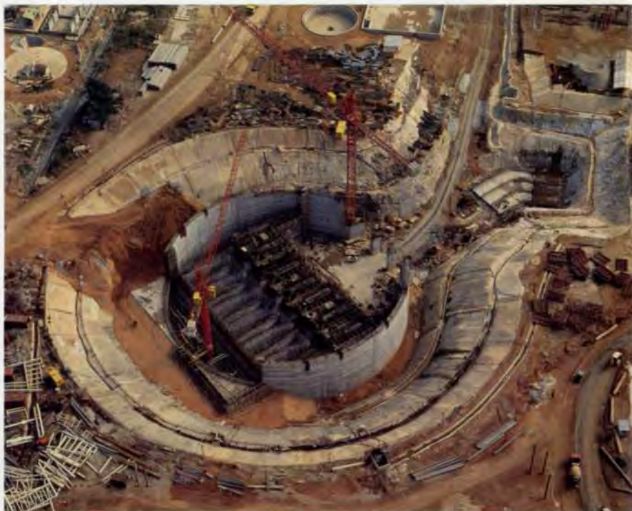
7. CW pumphouse external wall complete, pump chambers in progress, November, 1993
