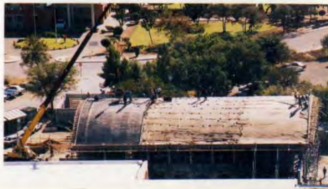
4. New building under construction.
