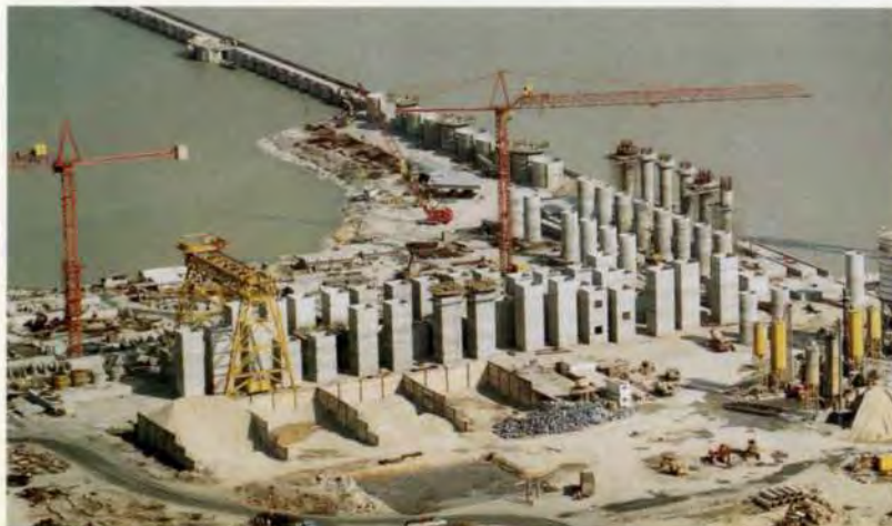
11. Culvert and caisson precasting yard and slipforming yard, May, 1994.
