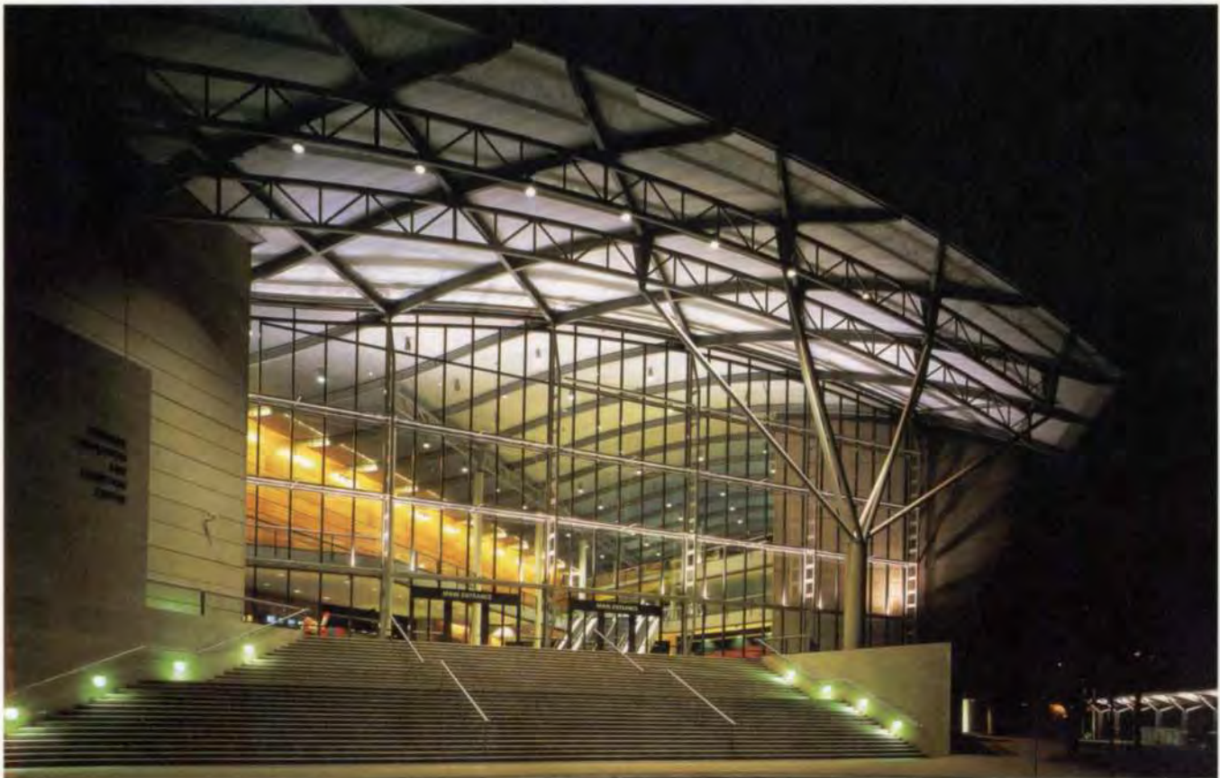
4. Main foyer entrance
