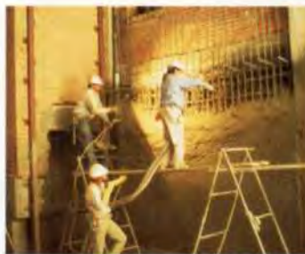
7. Shotcreting the Reference Room.
