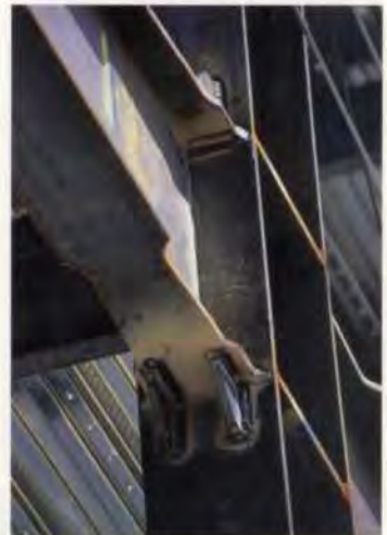
13. Outpatient clinic: moment connection after welding.
