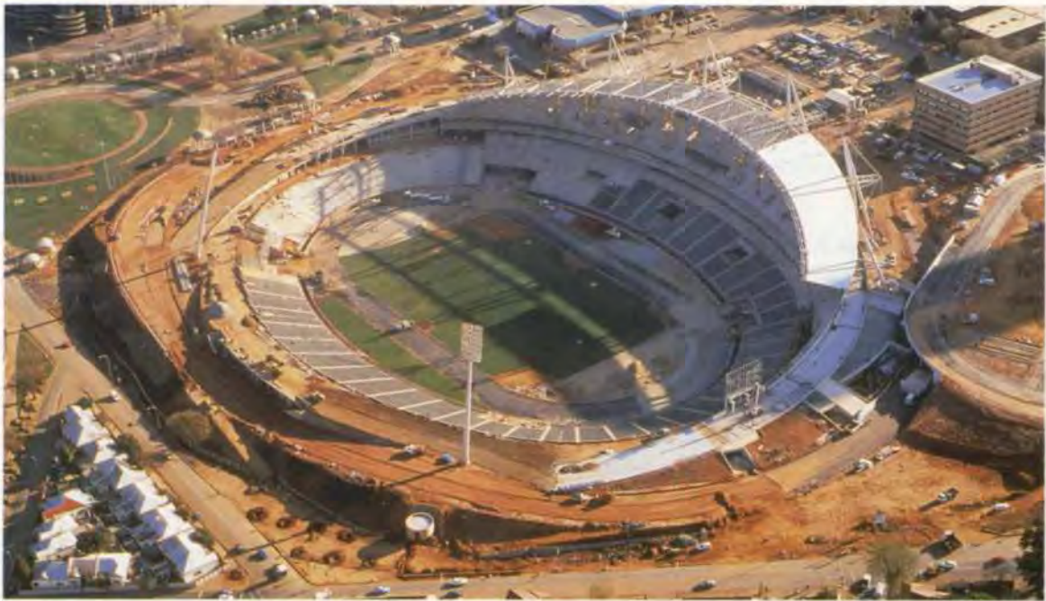
10. Site progress, October 1995.
