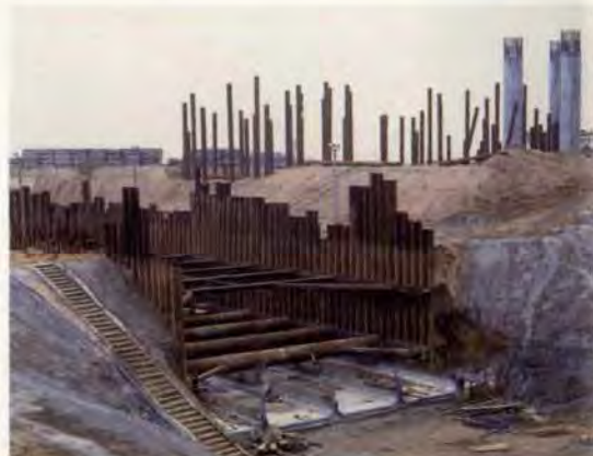
8. CW intake and outfall cofferdam under construction, March, 1994.
