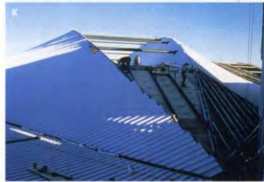
• Finally, the purlins, roof sheeting, and ceiling were installed (K).
