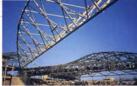
G. Bowstring truss stabilised by overhead cables with perimeter frame and V-truss.
