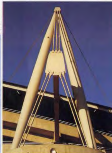
15, 16. Bracing element and A-frame, as built.
