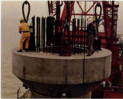
15. Attaching lifting frame to jetty caisson.
