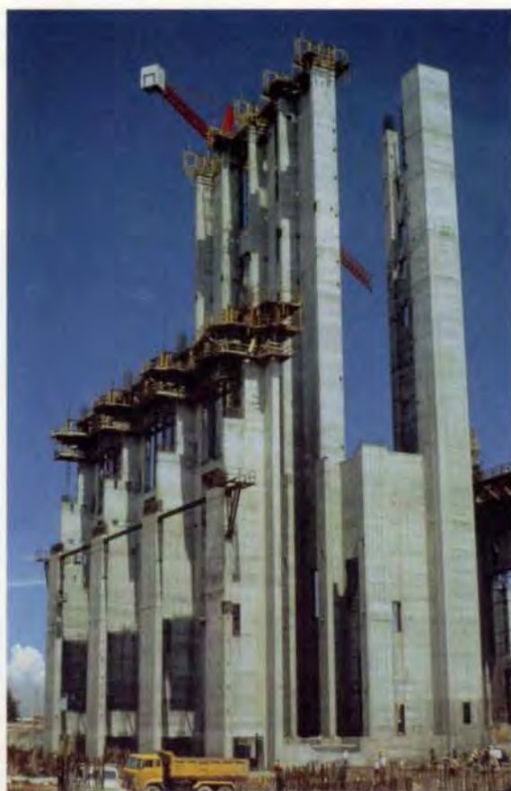
5. Slipforming unit 1 boiler and turbine hall, November 1993.
