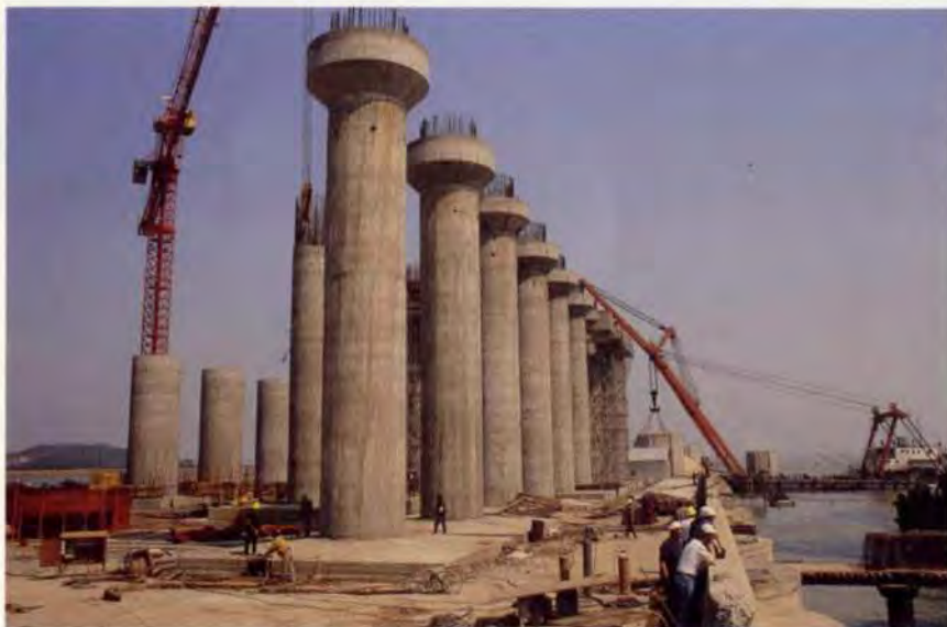
13. Slipformed jetty caissons awaiting placement, March, 1994.
