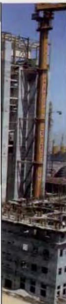
5. Slipforming unit 1 boiler and turbine hall, November 1993.
