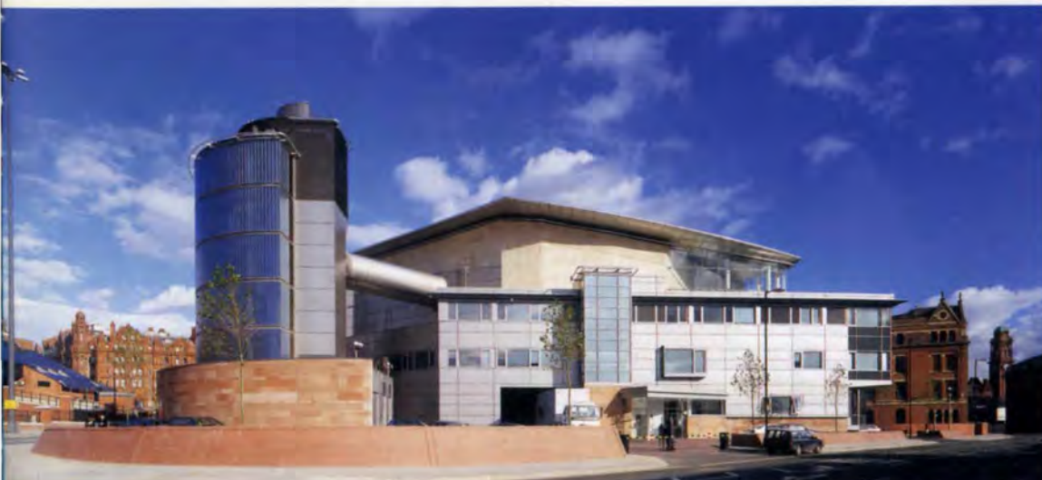
2. Rear view from south west, showing free-standing services tower.
