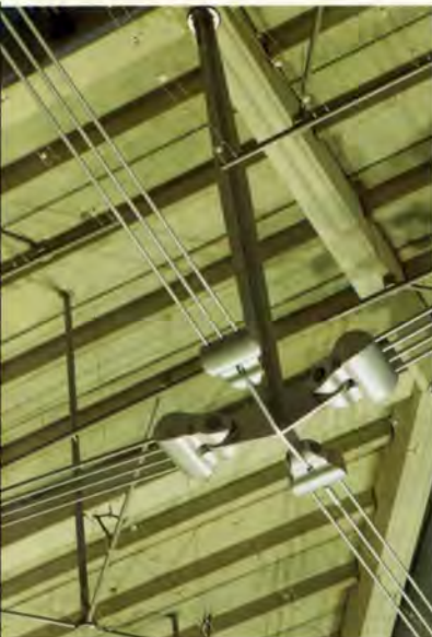
8. Close-up of roof support steelwork.
