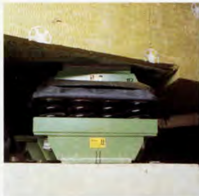
4. Spring box with cover off.
