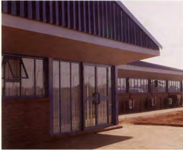
1. Administration block: front entrance.
