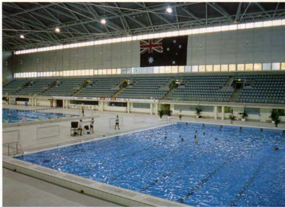
7. Utility pool, showing the removable wall for Olympic seating extension.
