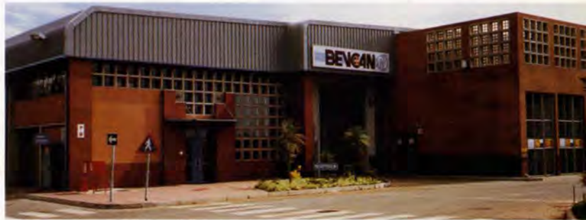
2. End plant exterior.
