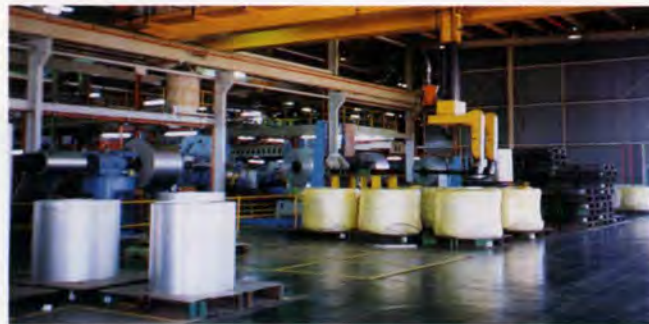
3. Coil store area.
