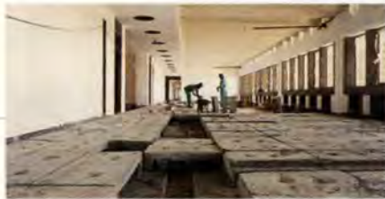
Office bay under construction, above 5: precast heat exchange sections being grouted into place, and below 6: Finished screeding to precast stools.
