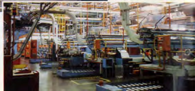
7. End plant interior.
