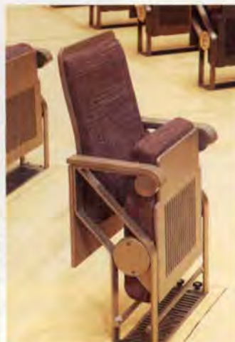
11. Stalls seat showing acoustic baffle, with underseat air grille.
