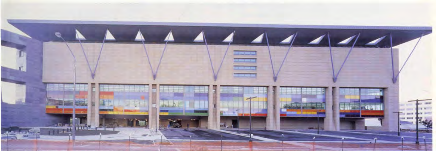
21. Southern elevation from Cable Street. Uplift pressures of up to 7.5kpa were designed for on the cantilever roof..
