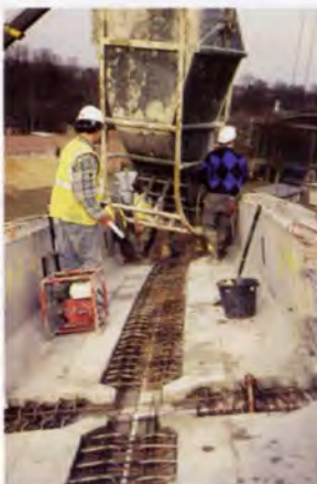
10. Pouring in situ stitches to roof lower precast units.
