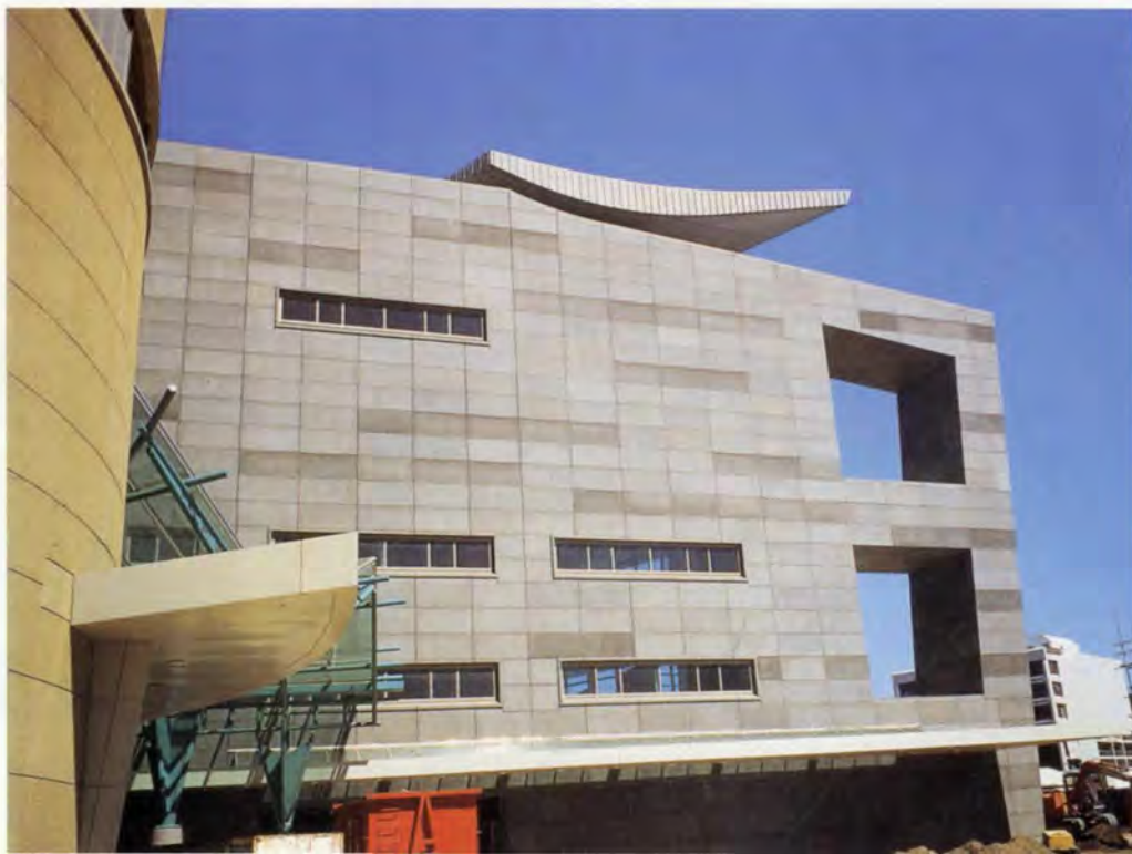
14b. (Below) South end of the Wall fully clad in basalt precast cladding.
