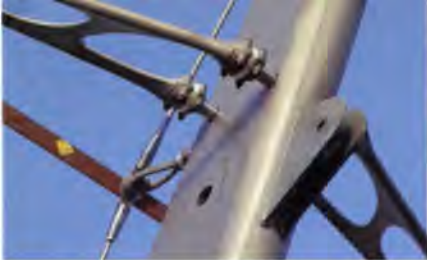
9. SG cast iron glazing brackets at Western Morning News.
