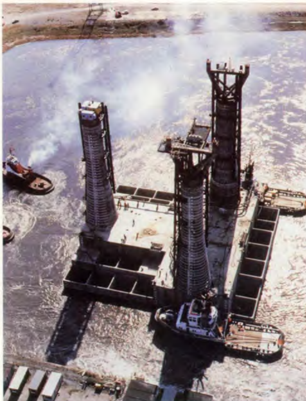
6. Ravenspurn concrete gravity oil platform.
