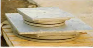
11. Two sizes of sliding bearings, awaiting installation below walls.
