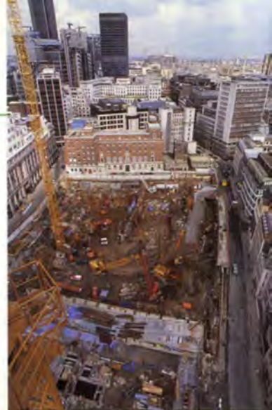
3. Minster Court excavation.
