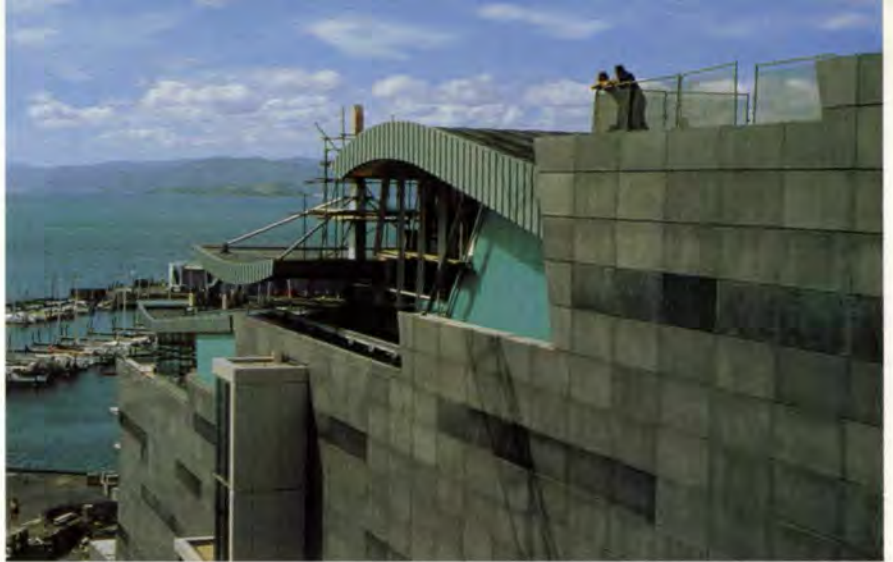
7. Looking down the harbour from the touring exhibition gallery, during construction.
