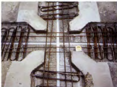
10. Pouring in situ stitches to roof lower precast units.
