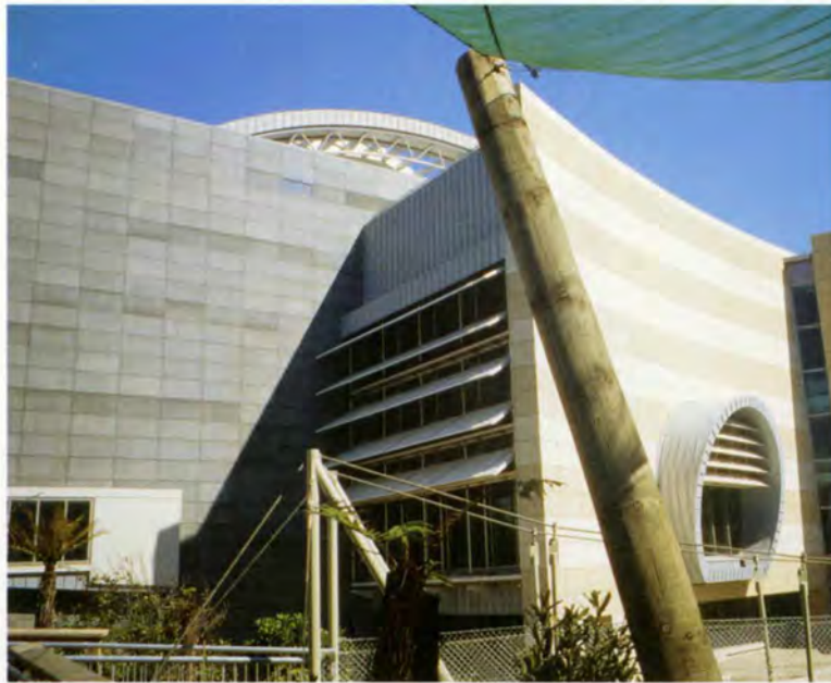
18. Orientation lobby from Harbour Park, showing curved precast panels.
