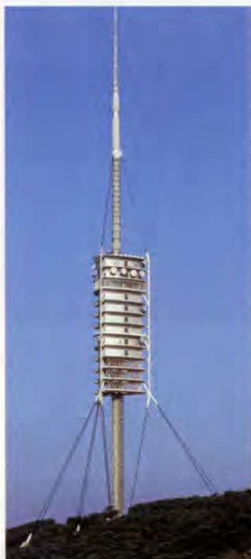
2. The upper guys on Torre de Collserola, Barcelona, are of non-conductive aramid, invisible to radio signals.
