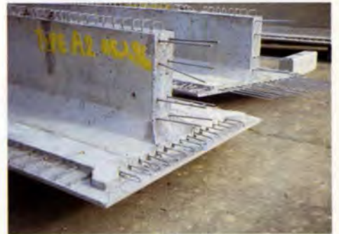
7. Lower precast units showing cast-in reinforcement for the in situ connections.
