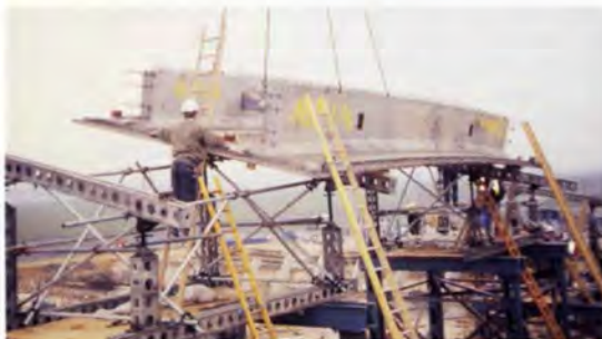
11 (below). Erecting and placing upper precast units.
