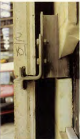
13. Panel/wall connection detail.
