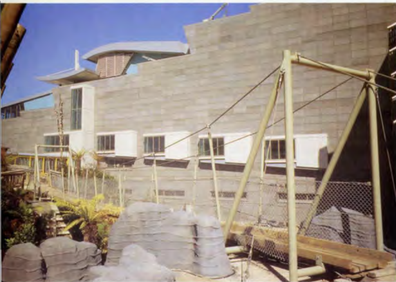
20. Harbour Park 'swing bridge' springing from replica limestone cave.
