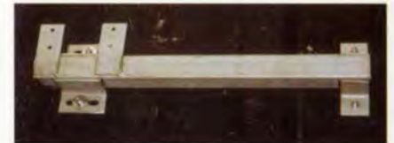
15. Bridging steel across seismic joint.
