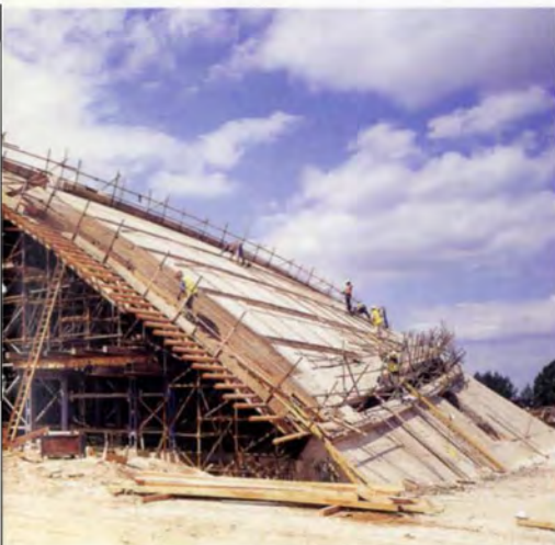
17. The completed shell roof prior to de-propping, June 1996.
