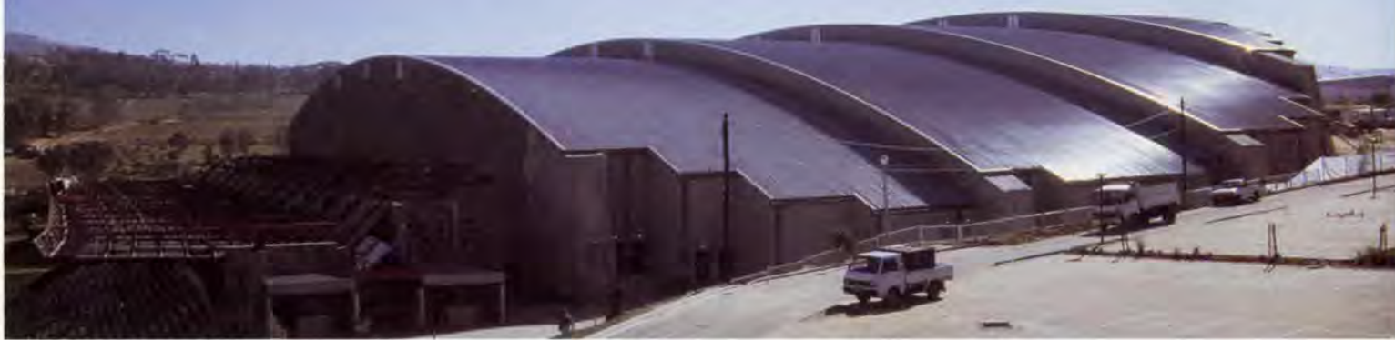
7. View of completed exterior, July 1997.
