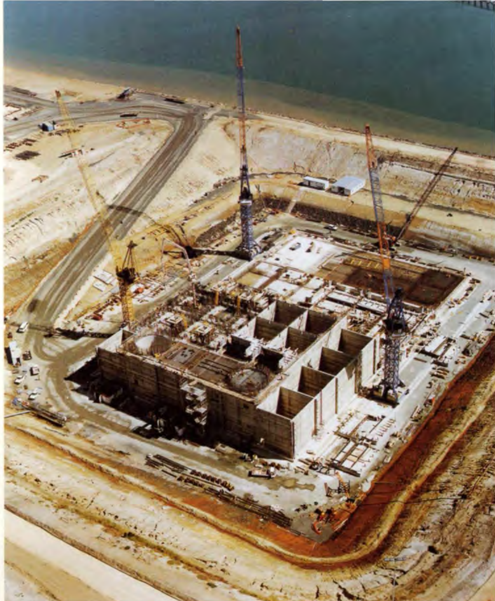
2. Caisson slipforming in progress, December 1995.
