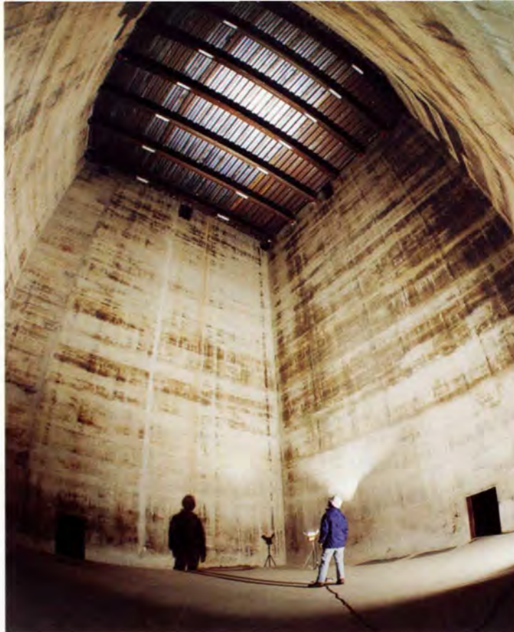
5. Interior inspection of closed cell during hydrotesting, July 1996.
