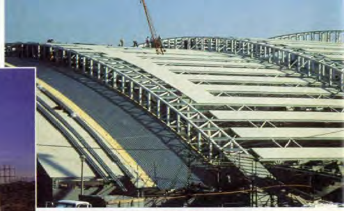
4 Above: Roof cladding in progress, May 1997.
