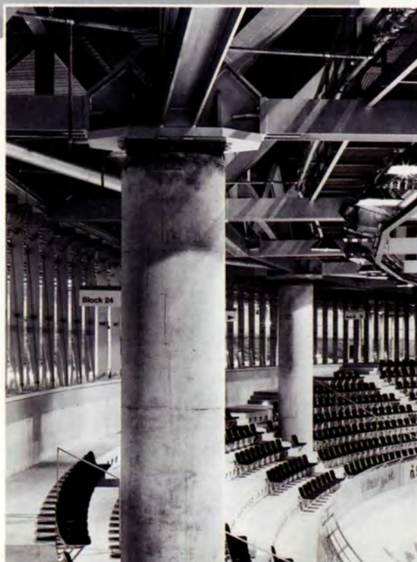
16. Column/roof connection detail.
