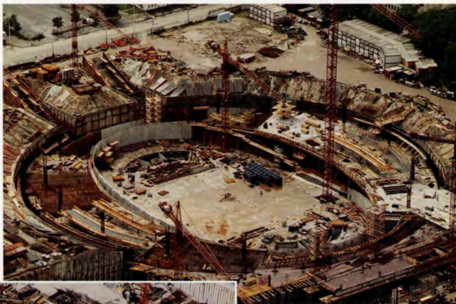
4 above: Before roof construction, June 1995.
