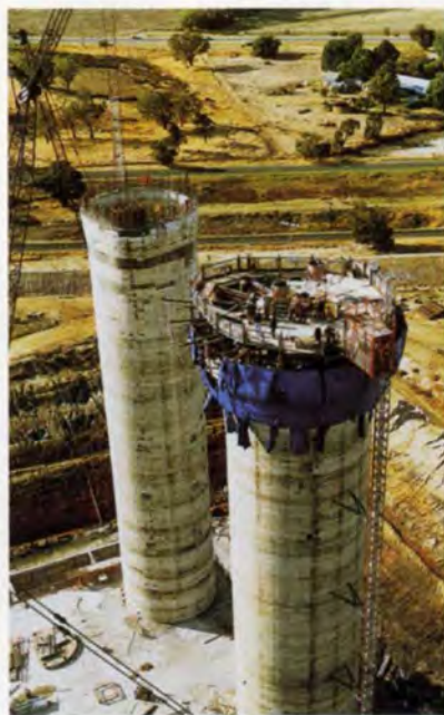
4. Shaft slip-forming, April 1996.
