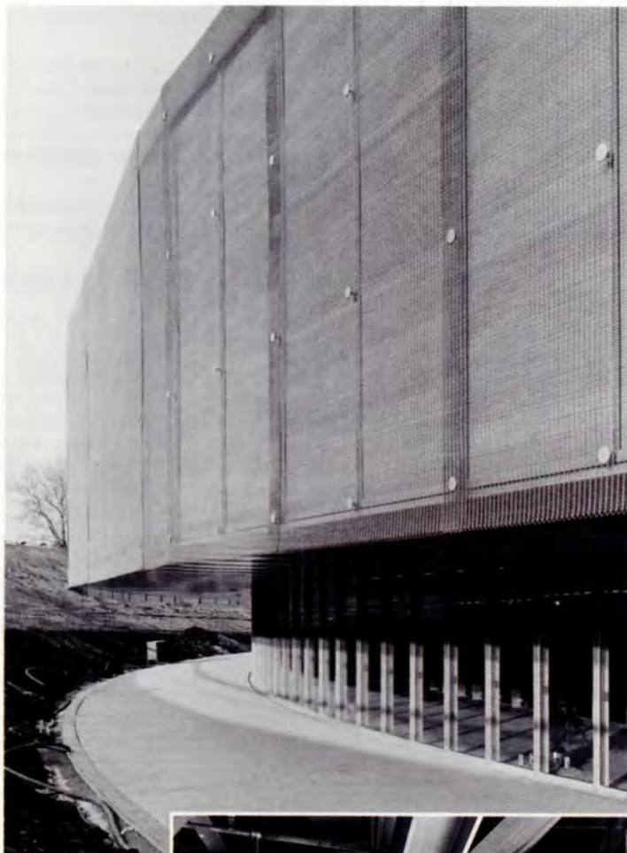
15. Stainless steel chain mail covers the walls and roof.
