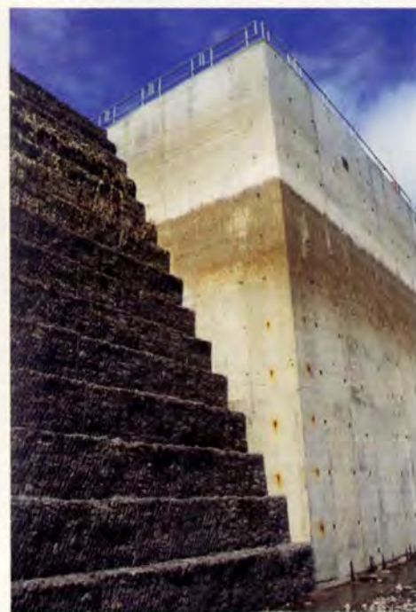
10. Completed Terramesh and counterfort retaining walls.
