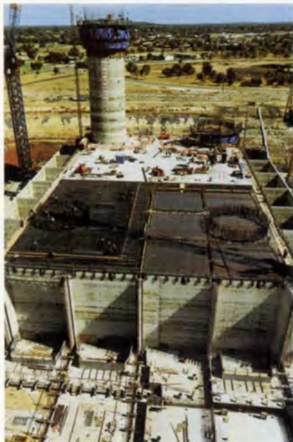
3. Progressive decking-out and concreting roof slab, with first shaft half-completed, March 1996.
