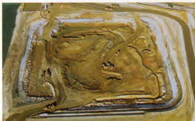
B. Casting basin construction, April 1995.
