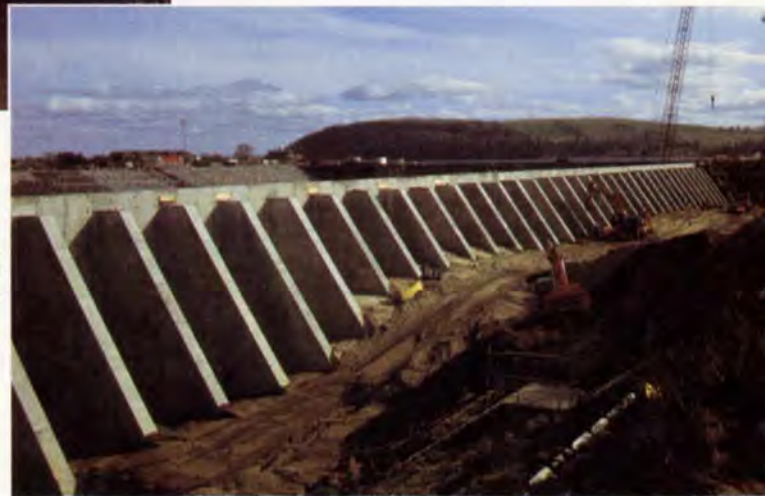
7. Back filling of the wall.
