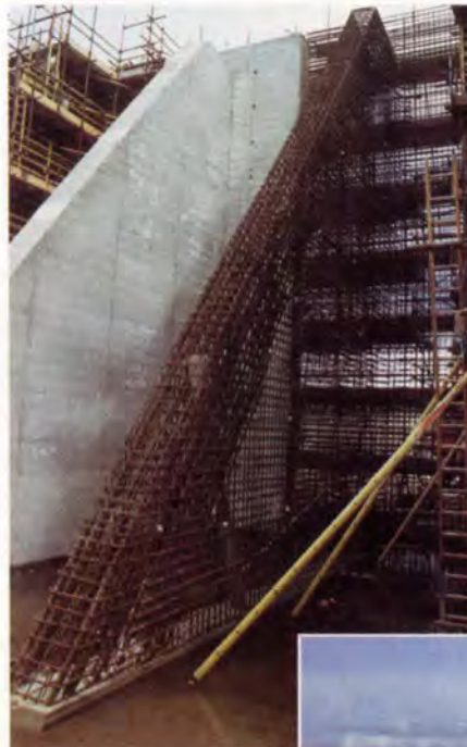
6. Counterfort reinforcement.
