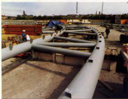
9. Plate girders supporting lower balcony. 10. Site welding primary arch.
