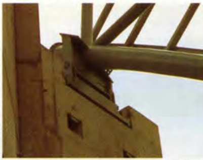
11. Connection between braced shell and flytower walls
