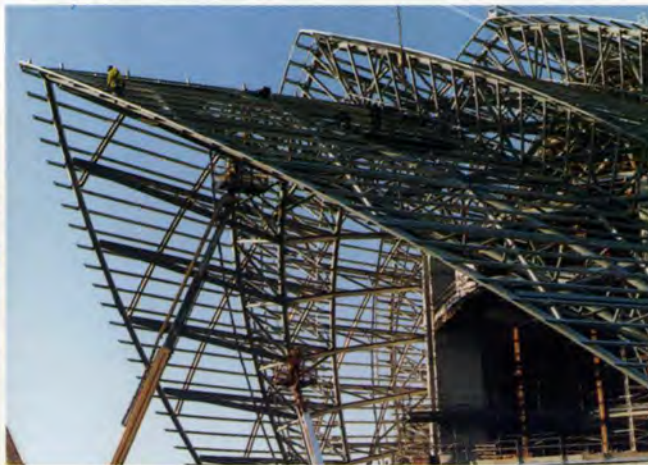
12. Braced shells 5 and 6 erected.
