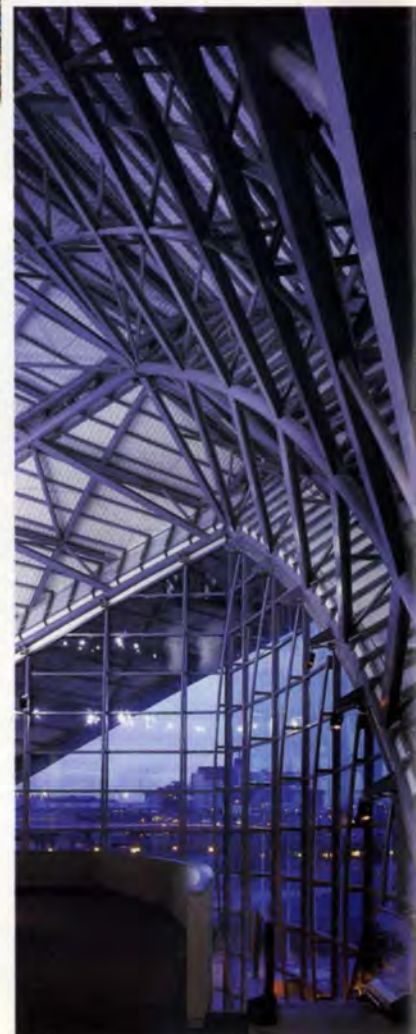
14 below: Steelwork over main reception area.
