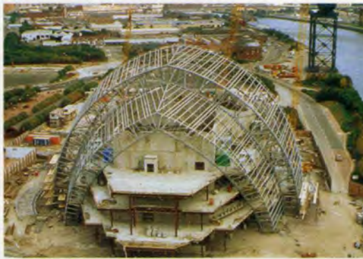
12. Braced shells 5 and 6 erected.
