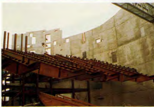
9. Plate girders supporting lower balcony. 10. Site welding primary arch.
