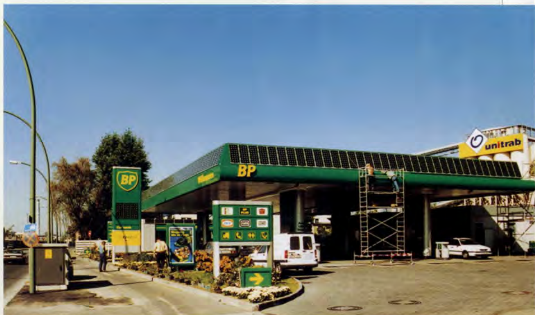
5. PV modules installed on Muhlenstraße filling station in Berlin.
