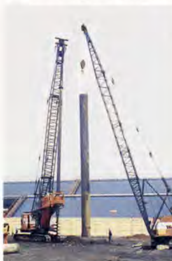
7. Bored pile: casing required to rockhead.
