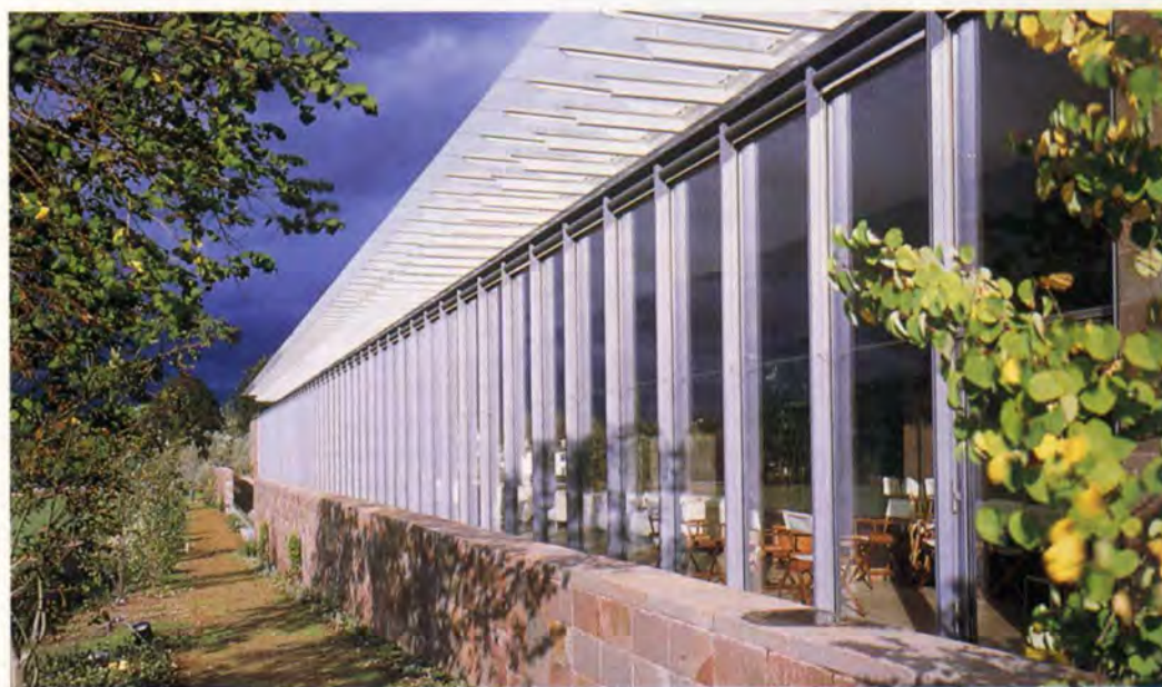
6. The west wall, looking north.
