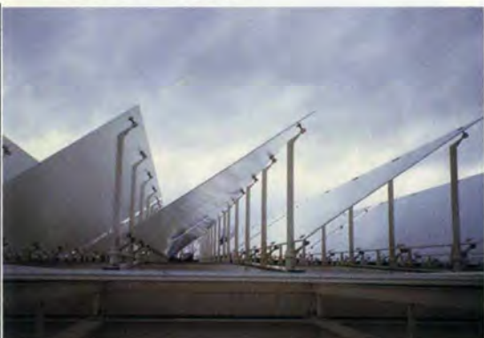
8. Brises soleil, looking west.
