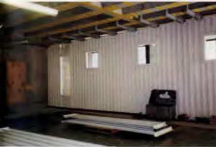
12. Blast protection to computer room.
