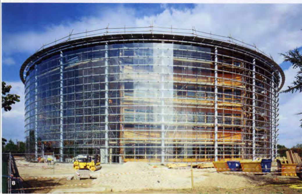
19 below: The circular design for Nº 4 The Square further develops the double wall theme with a shiplapped outer glass screen.
