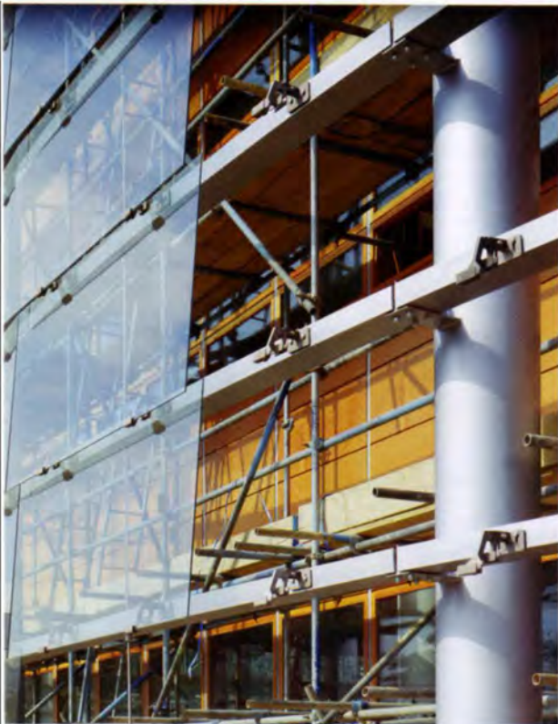
18 left: Nº 4 The Square: double wall under construction.
