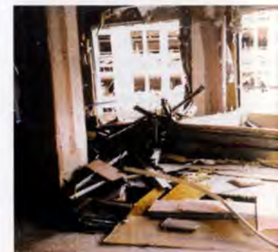
9. Bomb damage at Bishopsgate.
