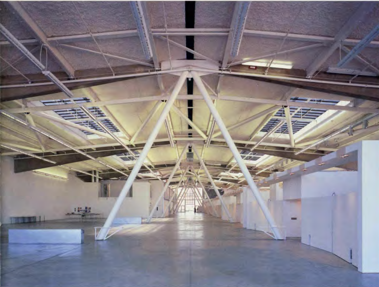
7. Interior view showing chevron braces and diaphragm trusses. Moveable partitions for graduate studios are to the right; enclosed classrooms and second floor graduate studios are to the left.
