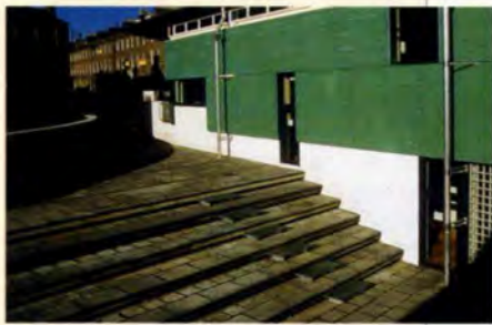
8. Terrace steps. Air conditioning intake grills are incorporated in step risers.
