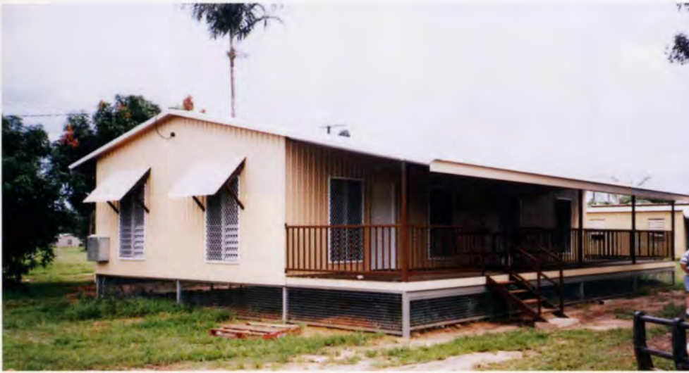
8. Completed housing in tropical Northern Territory.
