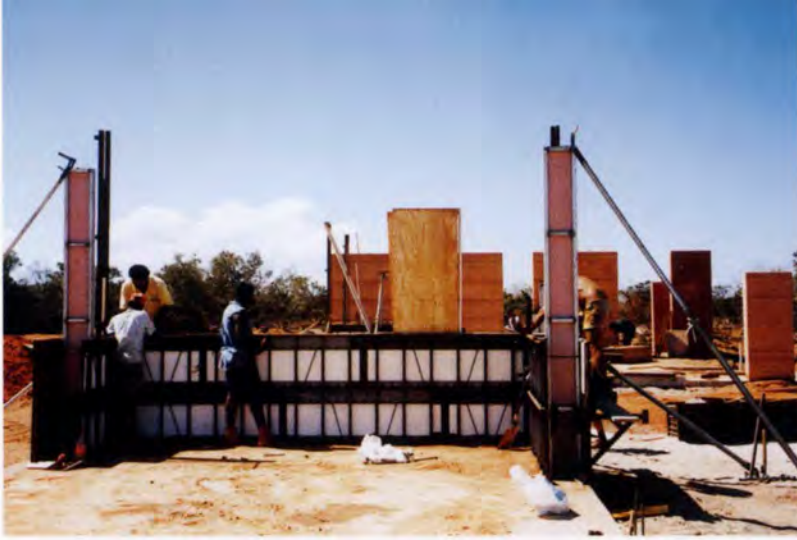
7. Rammed earth construction by local workers from remote community.
