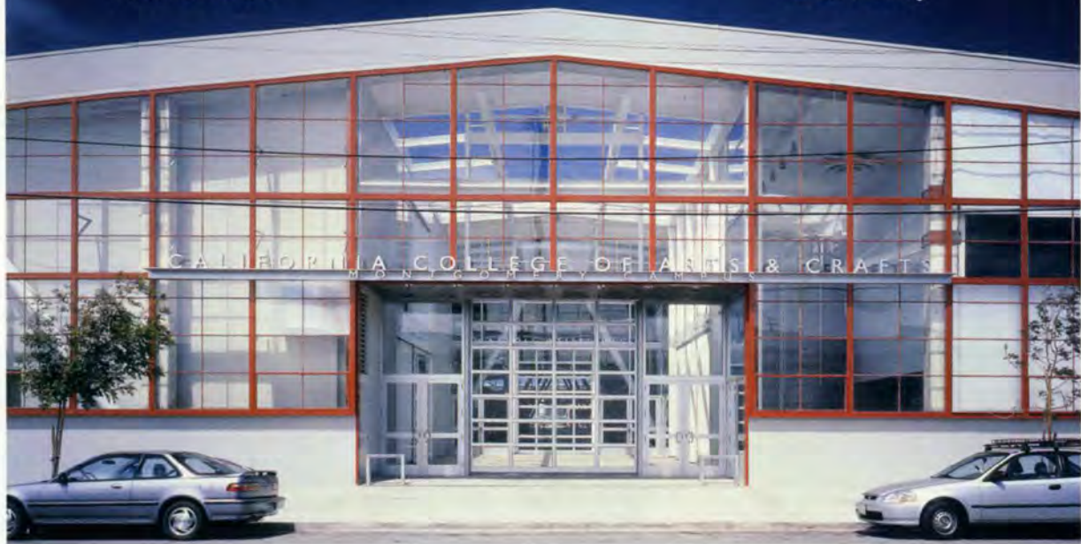
1. New main entrance to CCAC: the café is to the right and the Logan Galleries to the left.
