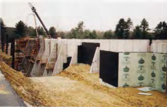
4. Counterfort retaining walls for Bar Building.
