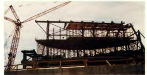
12. Temporary formwork for Gathering Space roof structure.
