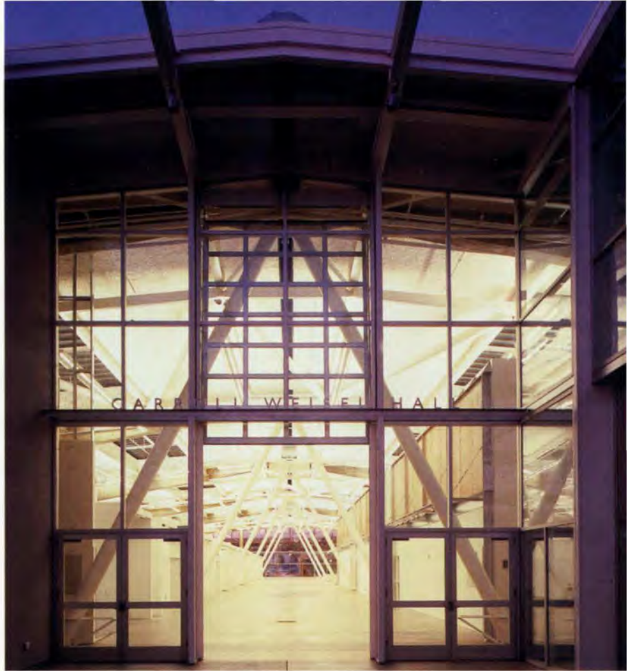
3. View down the nave from entrance courtyard, showing cantilever braces.
