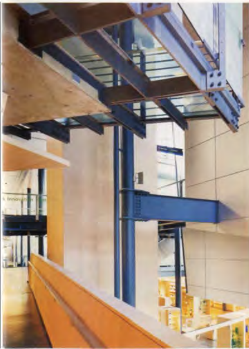
7. Underside of cantilevered glass floor of Windows Gallery.
