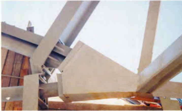
7 below: 'Bell' connection at top of Gathering Space.
