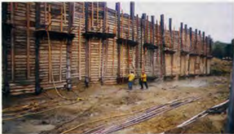
9. Waling structure for deep basements.
