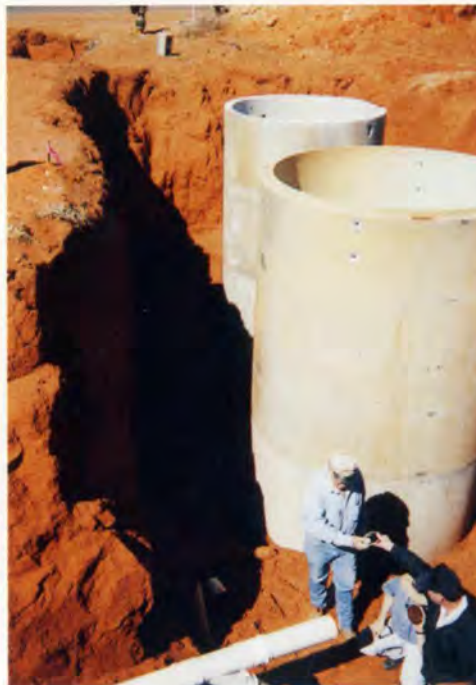
3. Pump station construction in desert community.
