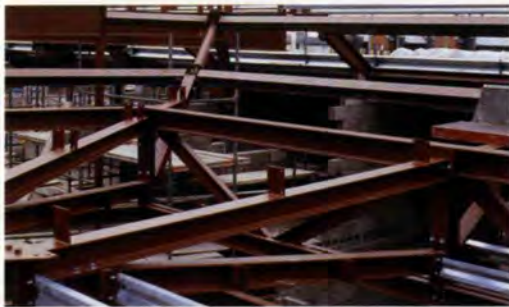
11. Roof steelwork at valley.
