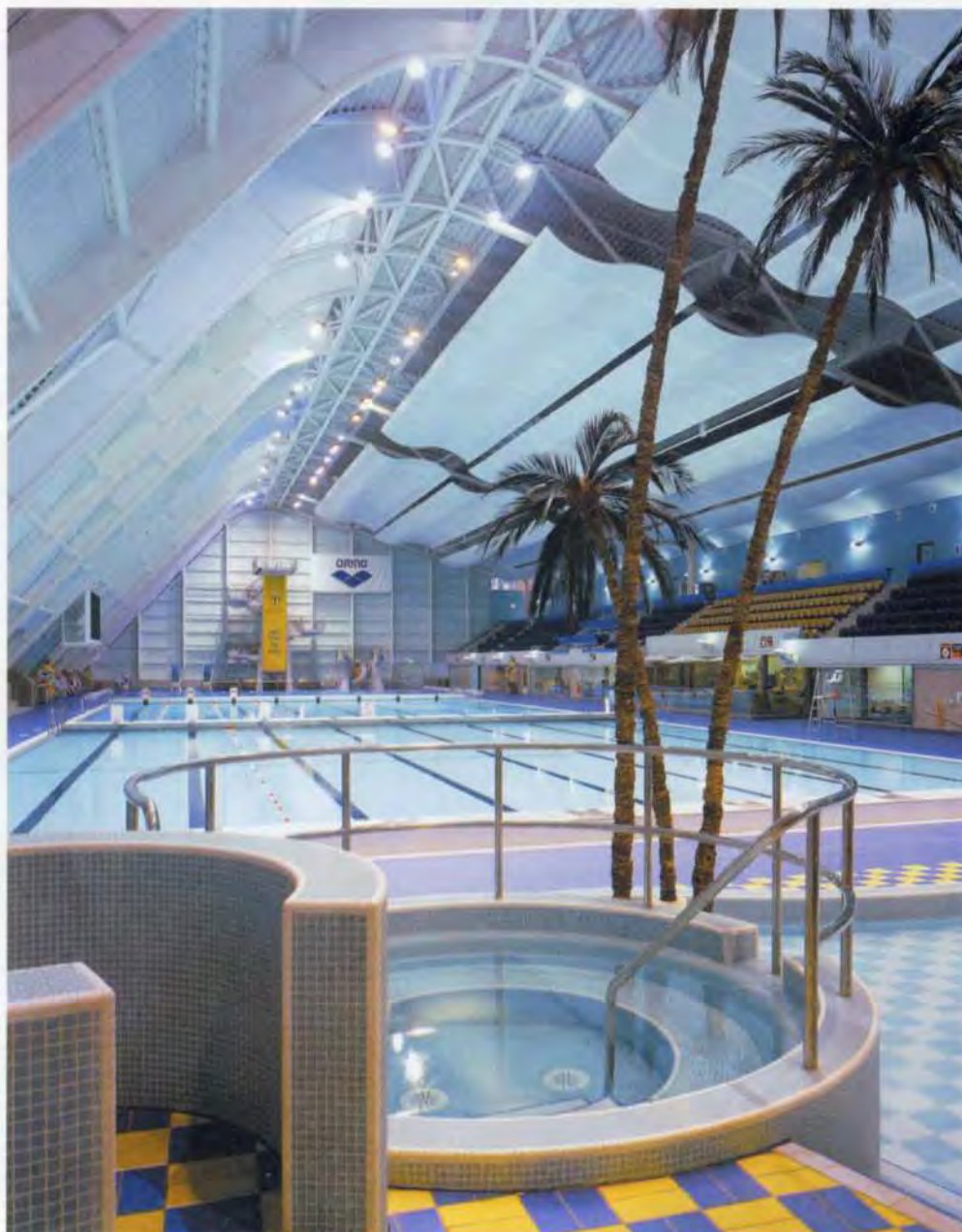
12. Floodlighting in the main pool.
