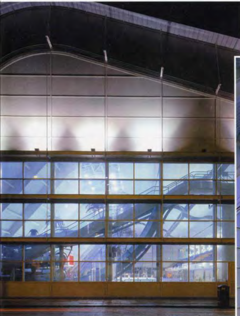
6. Flume access stair.
