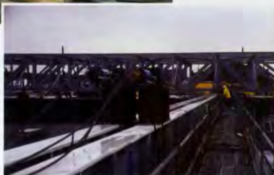
7. Launch rails and jacking point.
