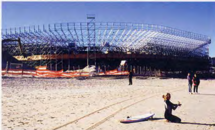
5. Temporary velodrome on Bondi Beach under construction.
