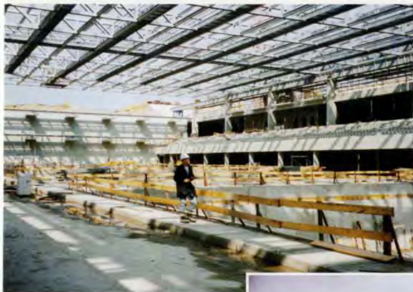
6. Partially launched Schwimmhalle roof.
