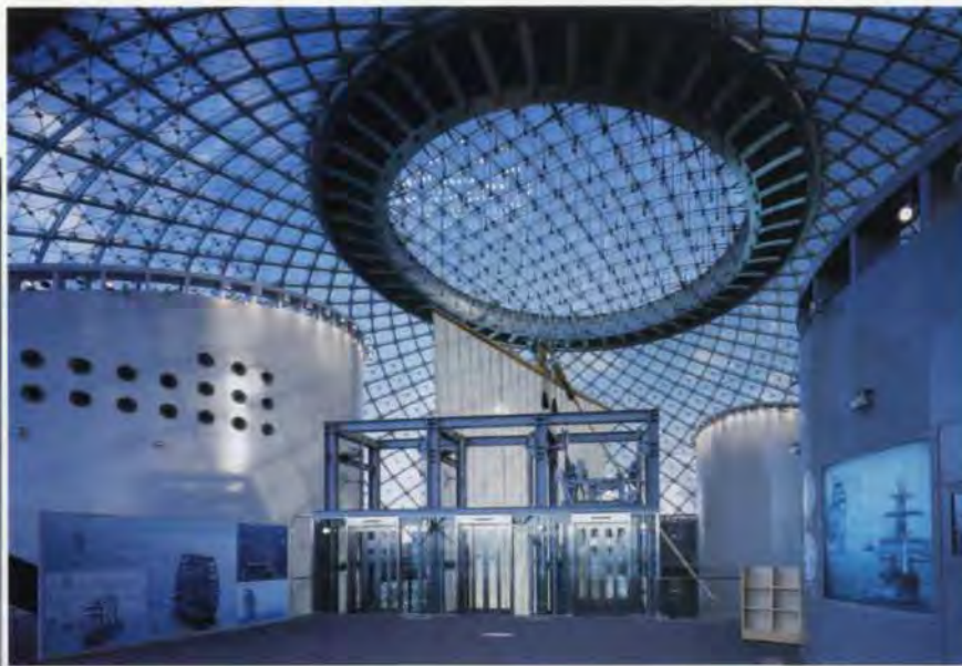
10. The third floor, showing the three core structures, the transparent riser, and the ring beam above.
