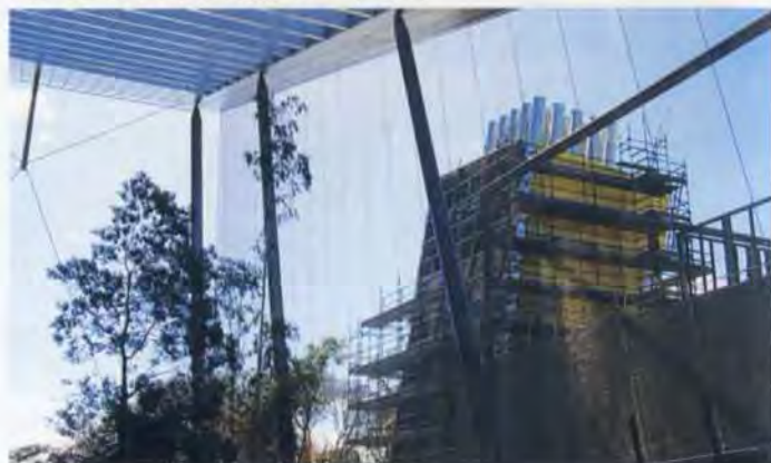
9. One corner of the Forest Gallery, showing cable-supported mesh enclosure and its degree of transparency.
