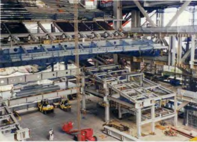
17. The auditorium under construction.
