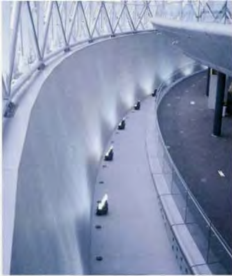
13 above: Inside the dome perimeter, showing the space between the dome and the internal floors..
