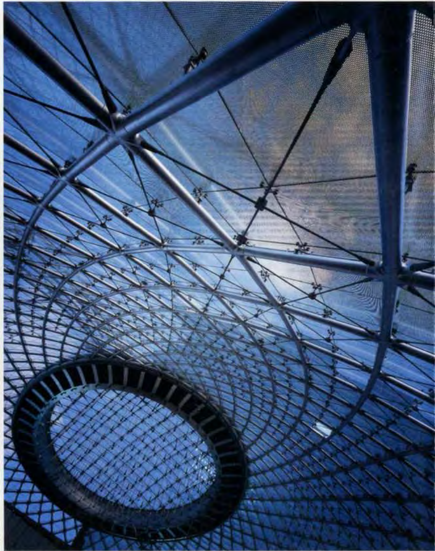
15. The diagrid shell and the ring beam.
