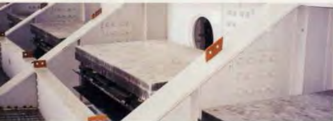
19. Tuned mass dampers.
