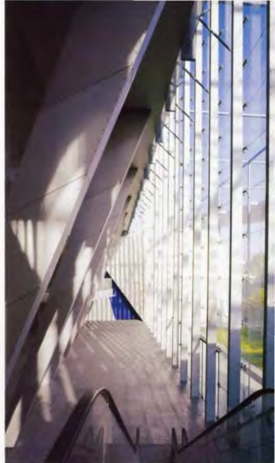
13. Internal view of the 22m high glass wall to the foyer.
